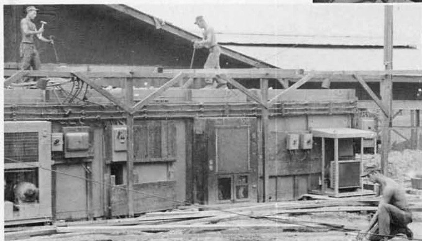
Bravo Company UT's went to work remodeling the galley.
