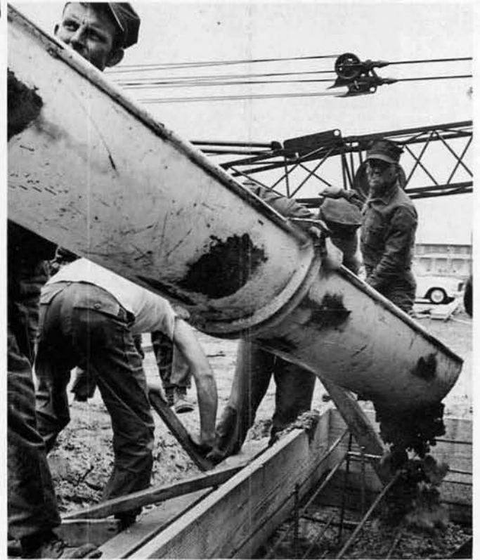
Pouring concrete for the base of the mast.
