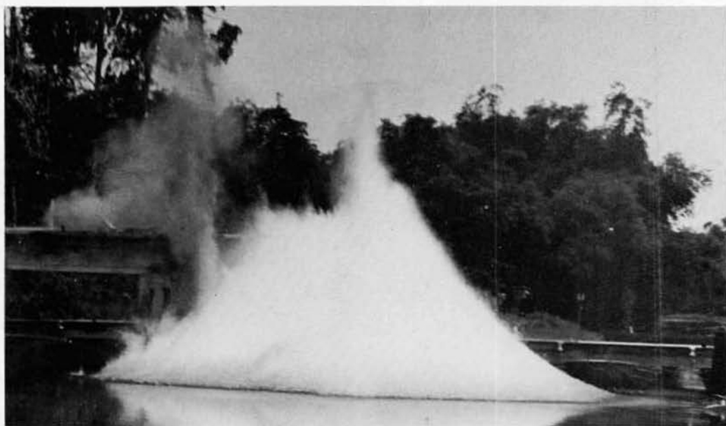
Divers from Alpha and Companies blast debris so bridge crews can get to work near Phu Lo
