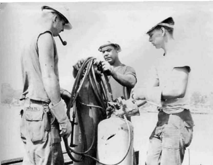
"SMITTY — KEEP THE PIPE AWAY WHEN THE ACETYLENE IS ON"
