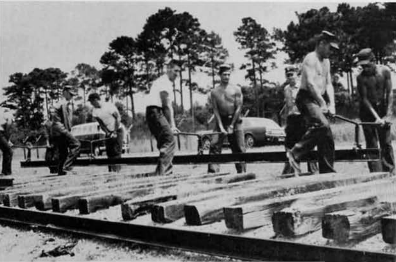
"I'VE BEEN WORKING ON THE RAILROAD"
