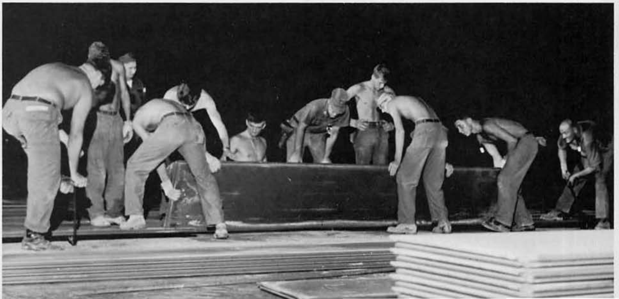
Night Crew on Matting Project
