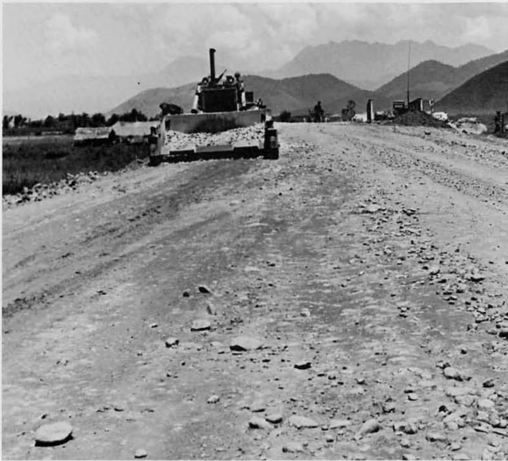
ROUTE ONE UPGRADING
