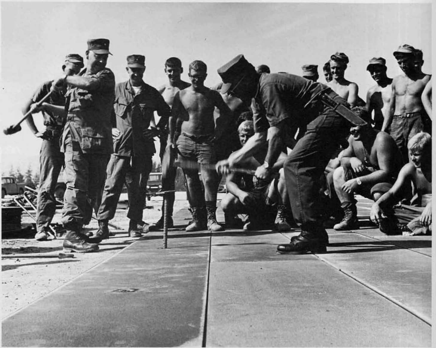
AIRFIELD MATTING (PHU BAI AIRPORT RUNWAY)
