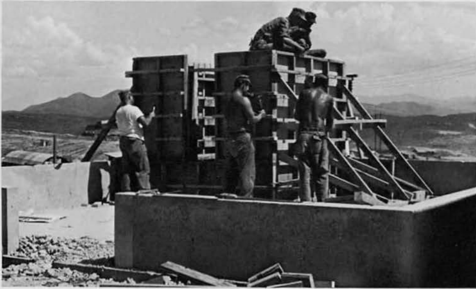
CONCRETE POURS AT 32nd N.C.R.
