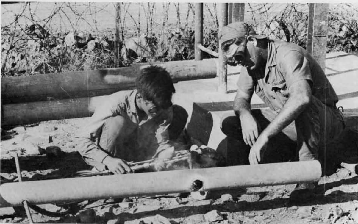
13301's M. D. Snyder and Steelworker trainee constructing power pole.
