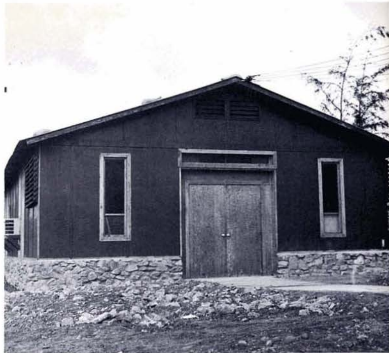
Chapel Renovation Underway
