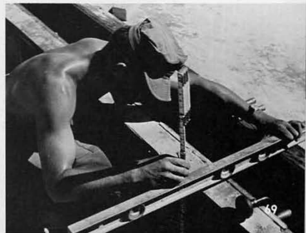
Jones checks forms for Ice Plant.
