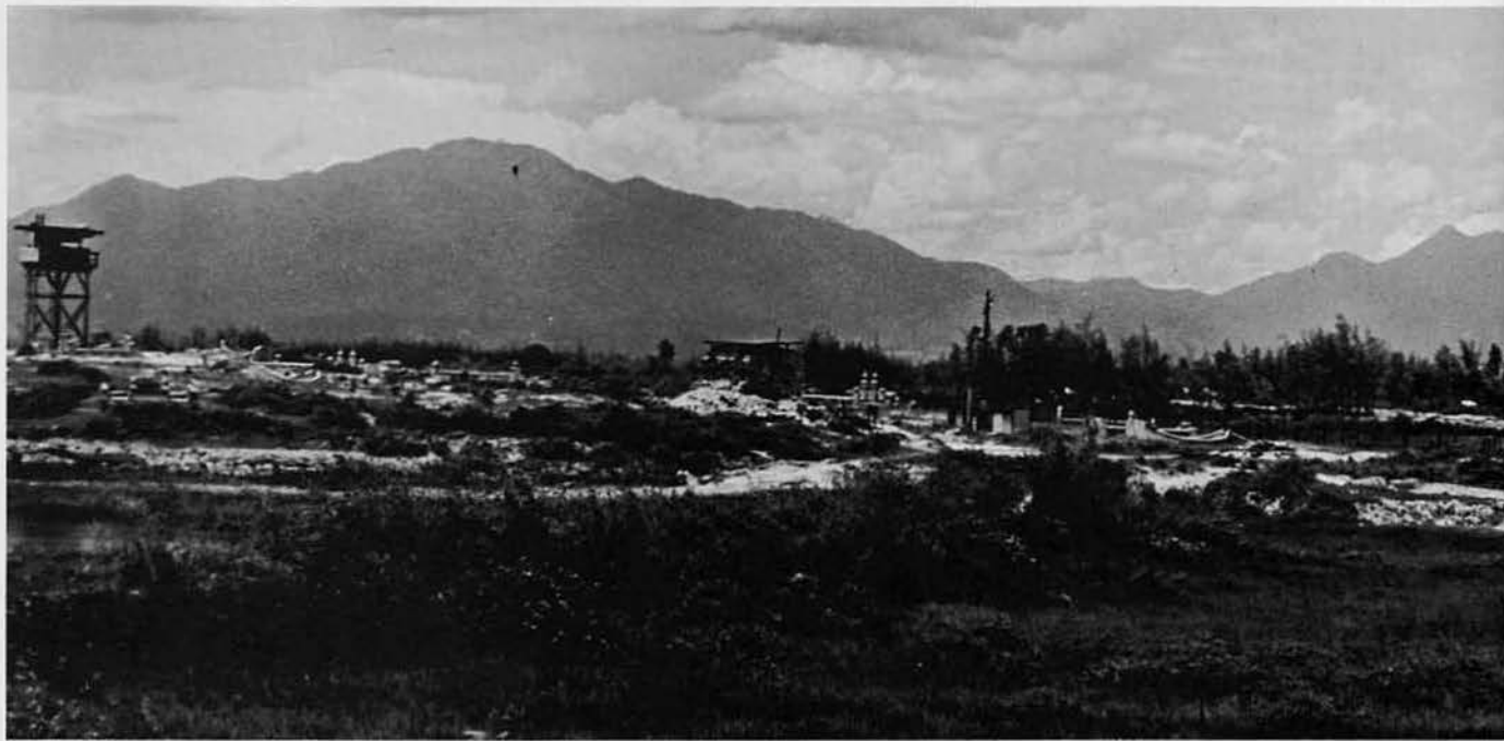
The stern face of the line perimeter
