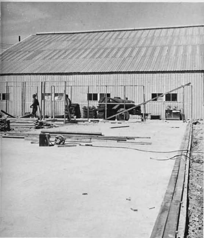
Construction begins at Marine Air Group 36 Operations building.
