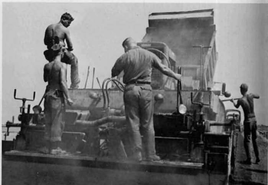
SPREADING ASPHALT
