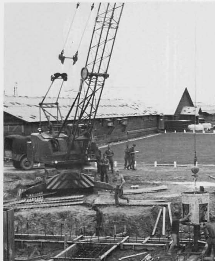
Above: Job at XXIV Corps where concrete footings are being poured for the Tactical Operations Bunker.
