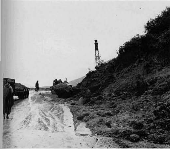
A Landslide due to heavy Monsoon rains
