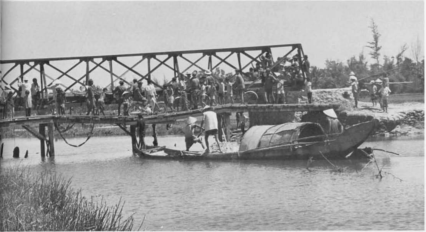
Villagers inspect My Loi Bridge
