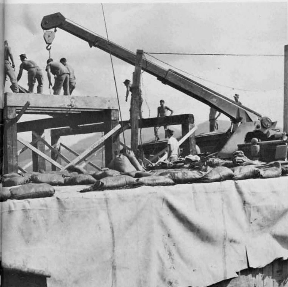
Building a radar tower at Fire-base Birmingham.
