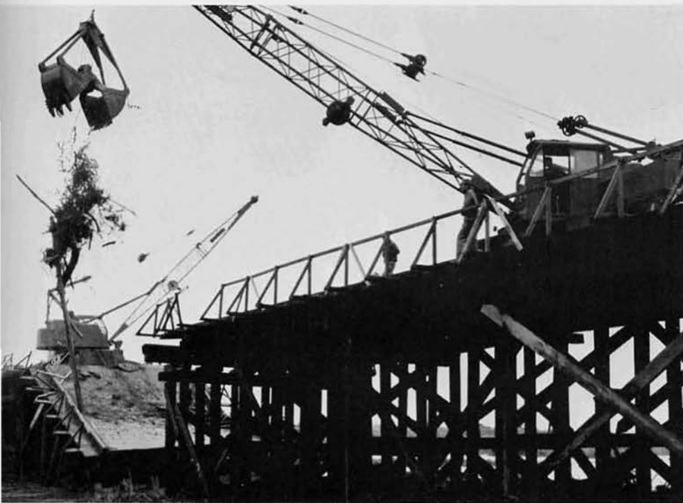
EO3 Settlemyer operating a clamshell rig at bridge 1-14.
