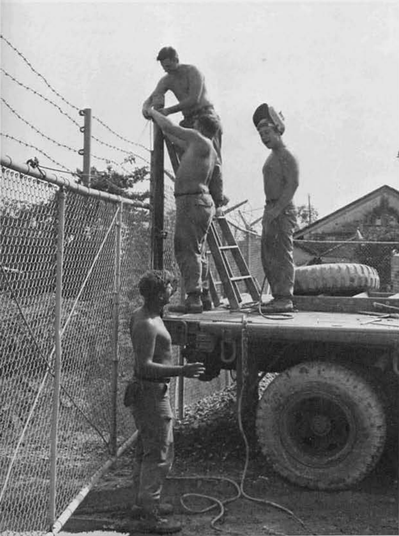
Another fence—this one at the East Hue Ramp.
