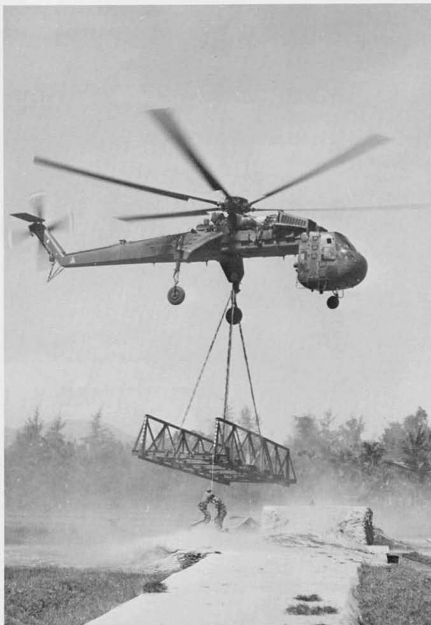
Helo sets My Loi Bridge into place
