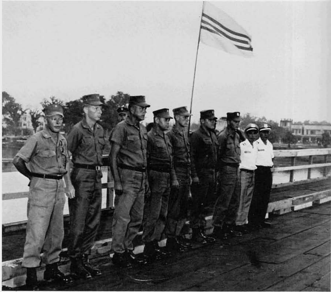
The Republic of Vietnam presents MCB 133 Seabees with Technical Service and Civic Action Medals for rebuilding the center span of the Hue Bridge.
