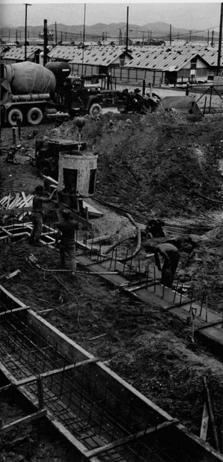
the XXIV Corps Tactical Operations Center.
