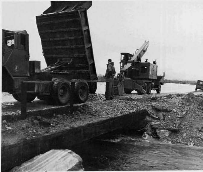
Repairing a washout in highway one.
