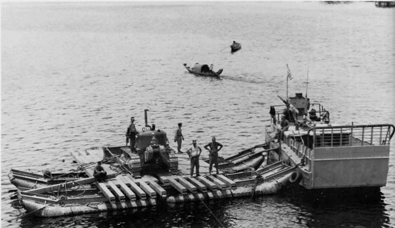
"Alfa afloat" while working on the Hue Bridge Project. The dozer was used to winch part of the debris from the ruined bridge out of the river.
