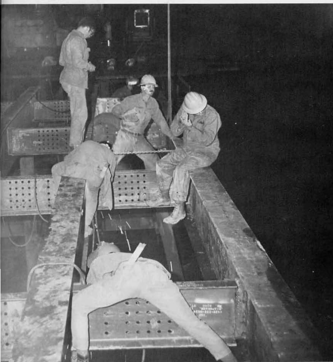
Welding stringers on the Hue Bridge.
