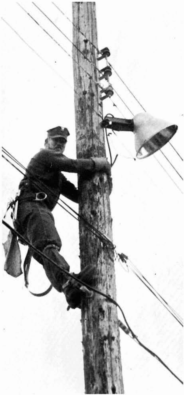
CE2 BURCHFIELD looks like he was born for pole climbing as he repairs a floodlight.
