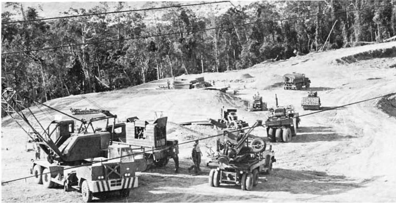
Seabee machinery set to continue carving out the housing relocation site
