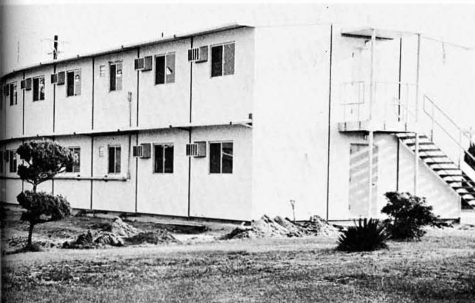
One of the fine Custom House BOQ's erected by the Bees of KANGROO
