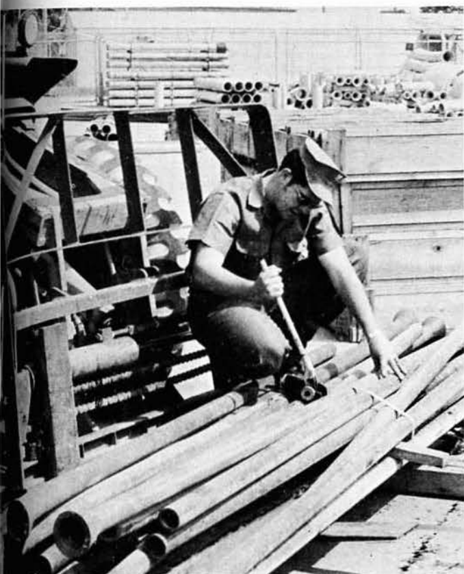
New pipe is banded in the MLO yard by EO3 BRANNEN.
