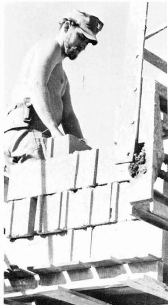
Concrete blocks for fire walls are unloaded by BU3 DELOZIER.
