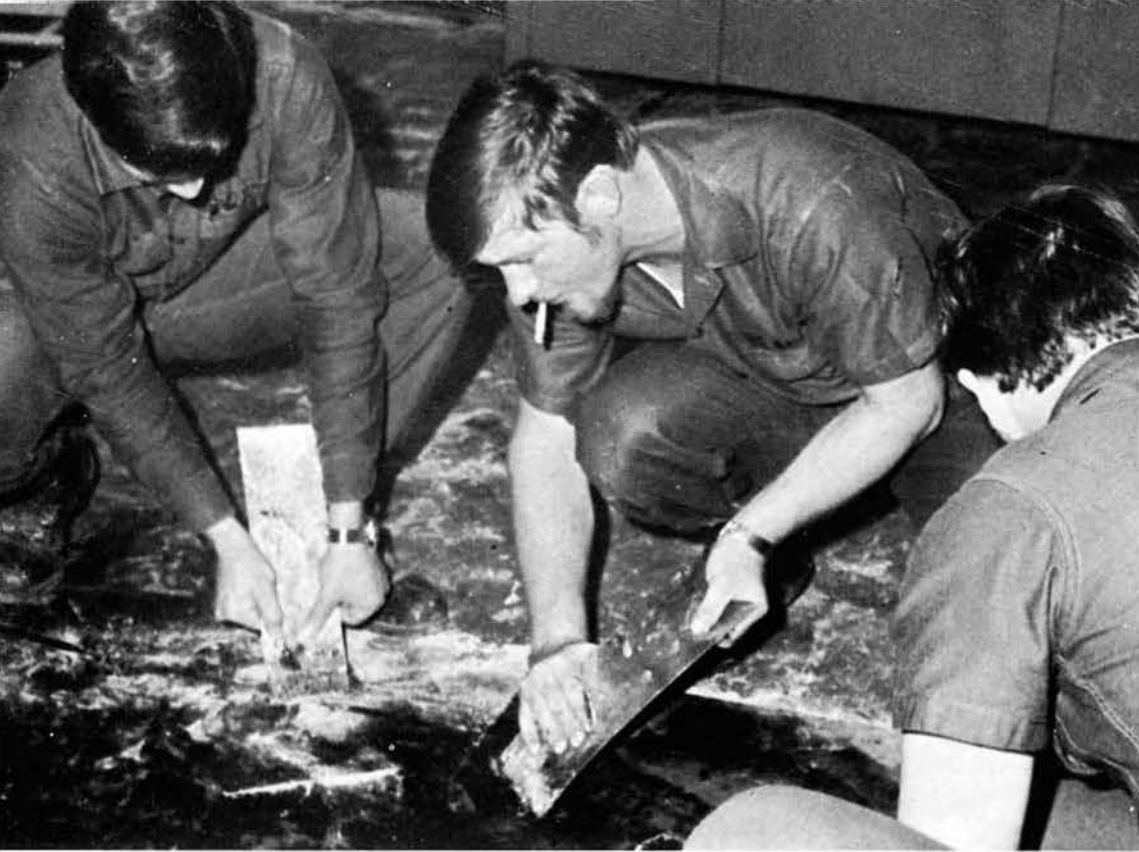
Coming to the aid of the disbursing office by replacing tile are Builders HAWLEY, KLEMETSON, and PLUTE.
