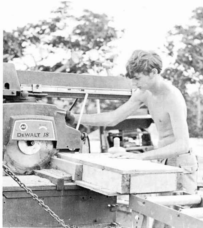
BU3 DIEBEL cuts forms on the versatile radial-arm saw
