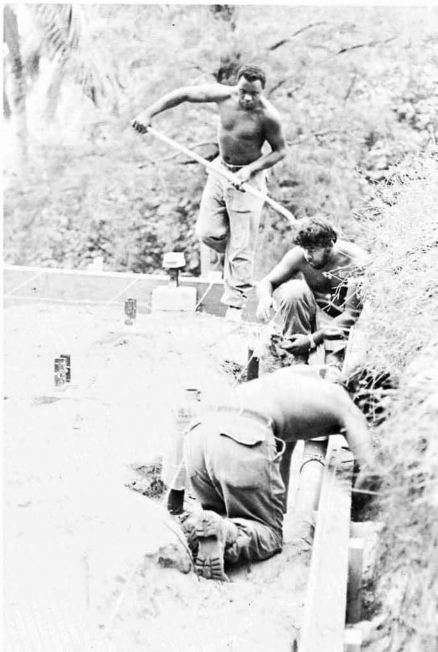
Form construction on the A-frame beach cottage
