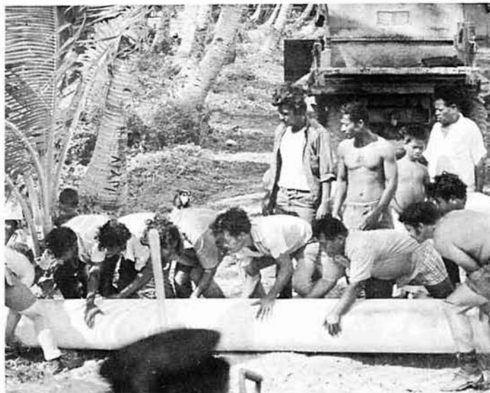
All hands take part in pipe installation.
