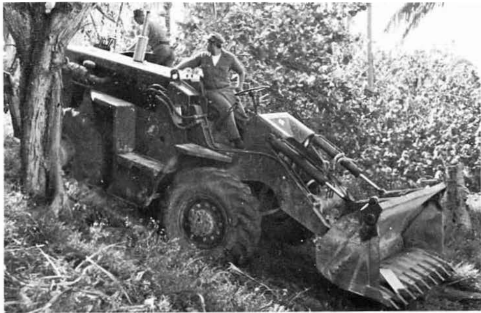
The multi-purpose front end loader with backhoe attachment excavates a ditch.
