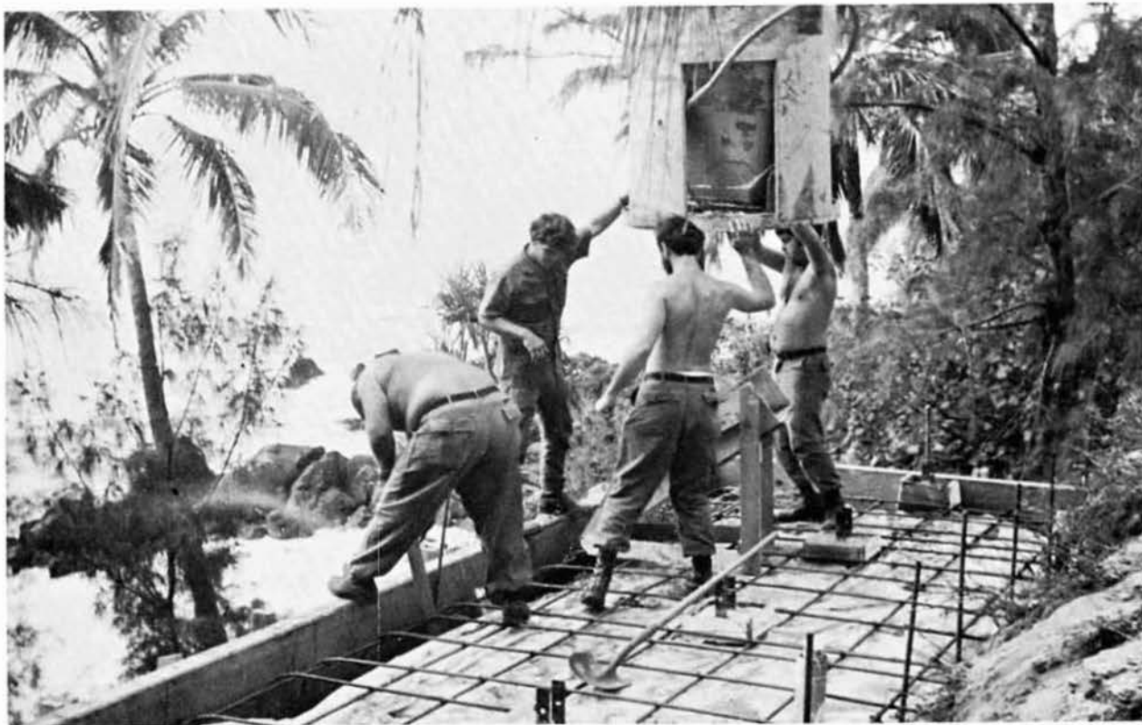
Cement is poured on the A-frame cottage utility porch.
