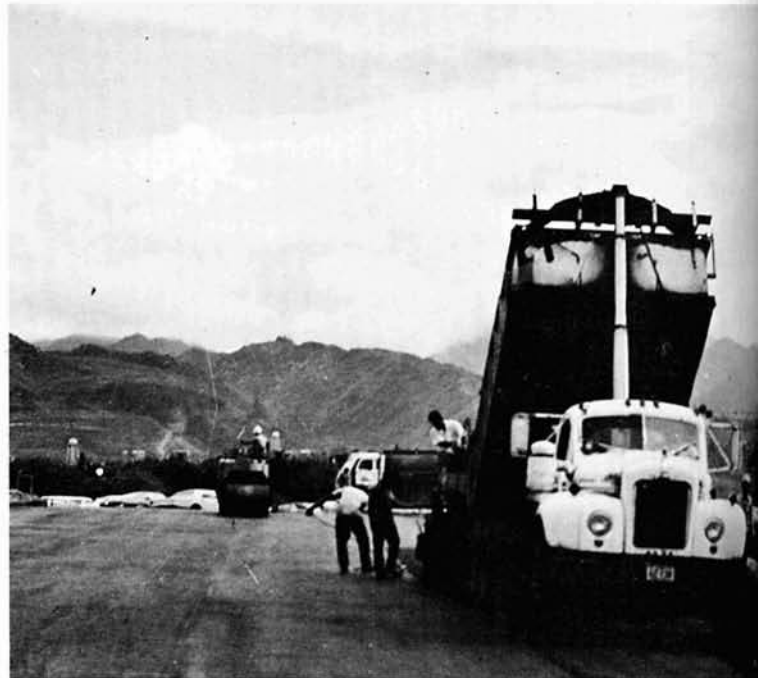
Early stages of the Makalapa Crater parking lot construction
