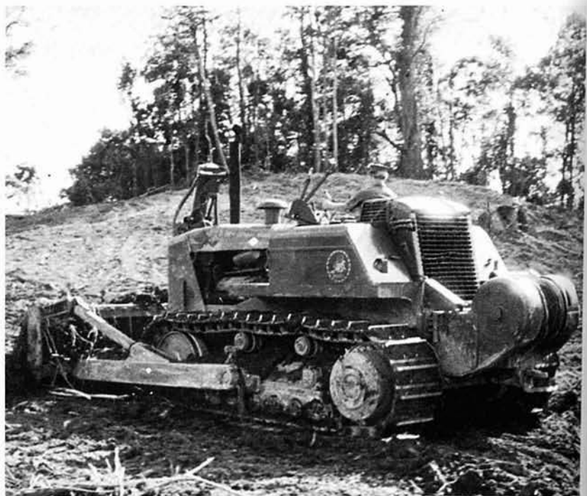
Clearing and grubbing were initial tasks.
