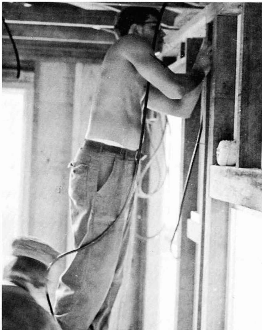
Rewiring the interior of a duplex unit
