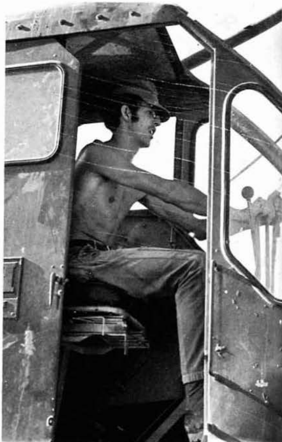
EO3 SWINDELL cuts loose with a mobil truck crane.
