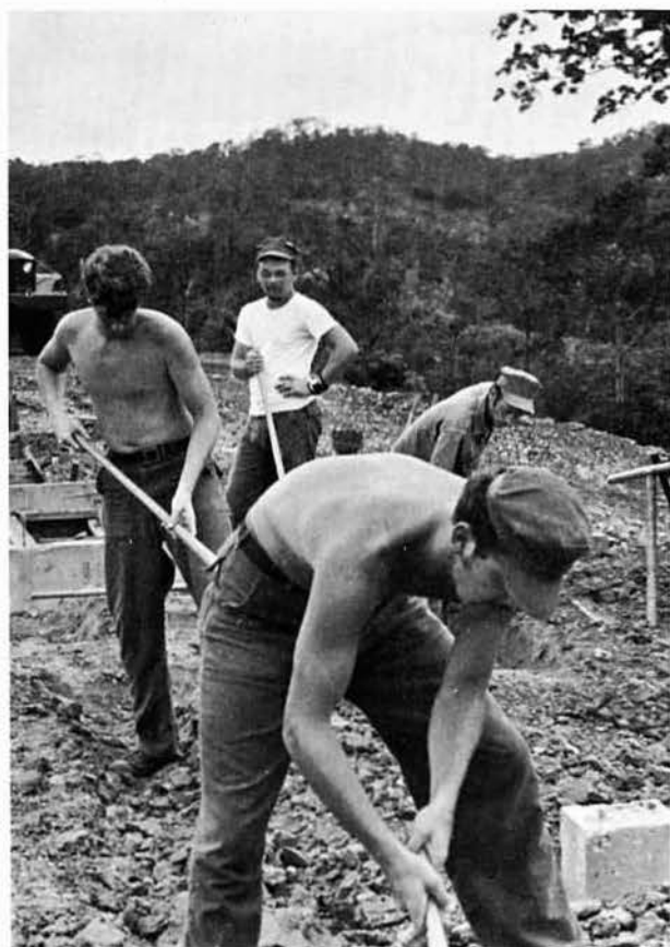
WALLABY's Builders had plenty to do in preparing the housing pads.
