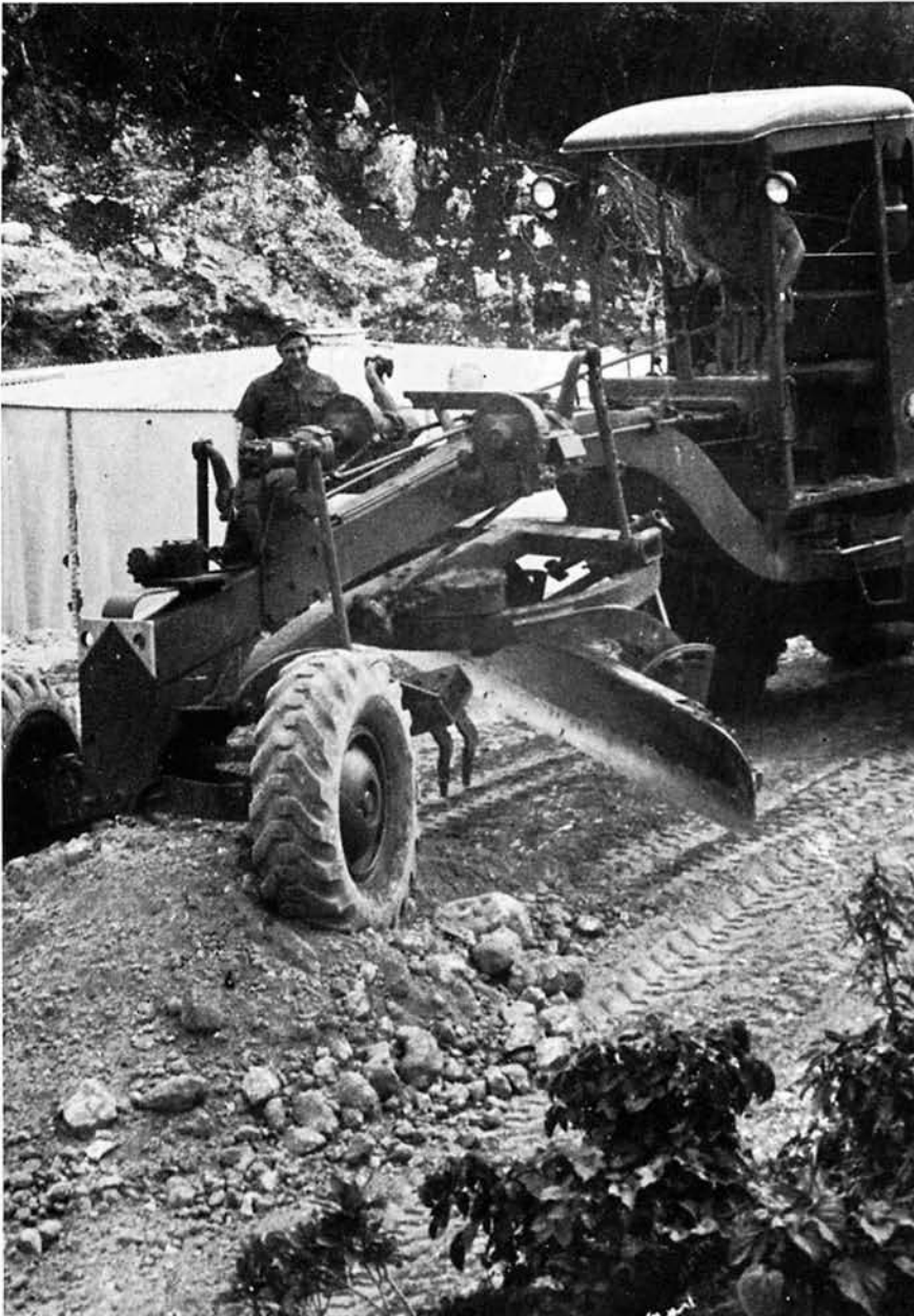
Roadwork leading to the site of Camp Shield's O-Club construction
