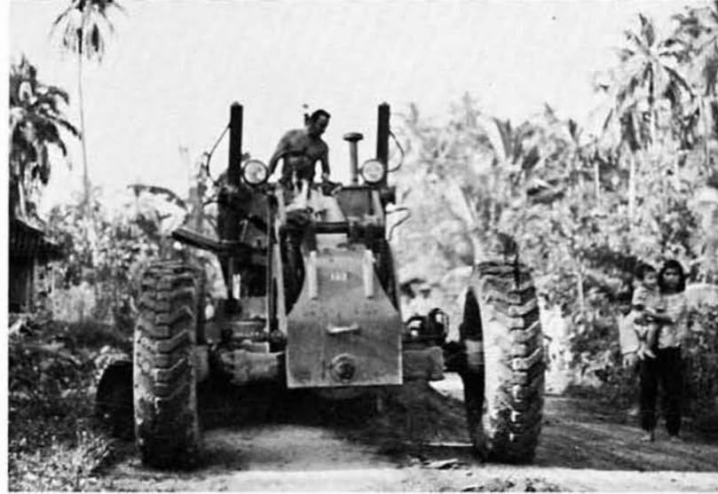
Upgrading the An Hiep Village road-EO2 GOLDEN
