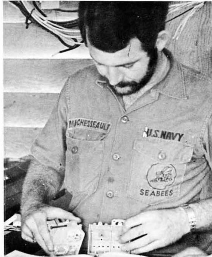
CECN MARCHESSEAU inserts fixtures into a 2S4 electrical box.
