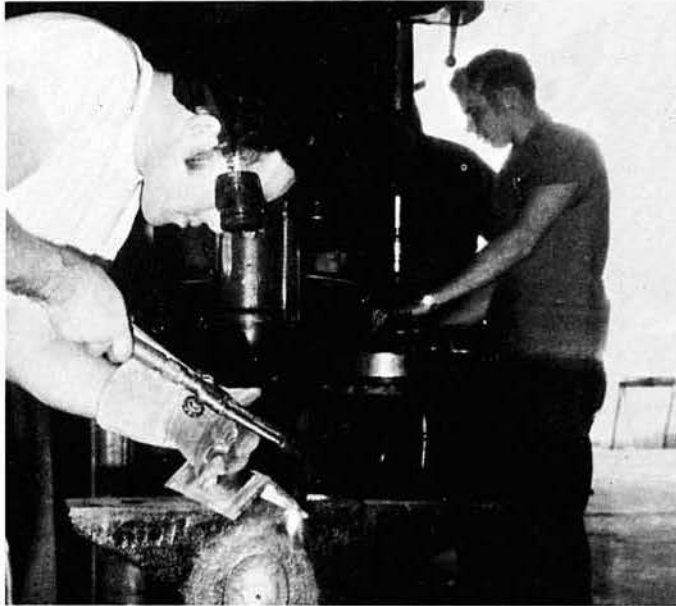
Busy Bees in the steel shop
