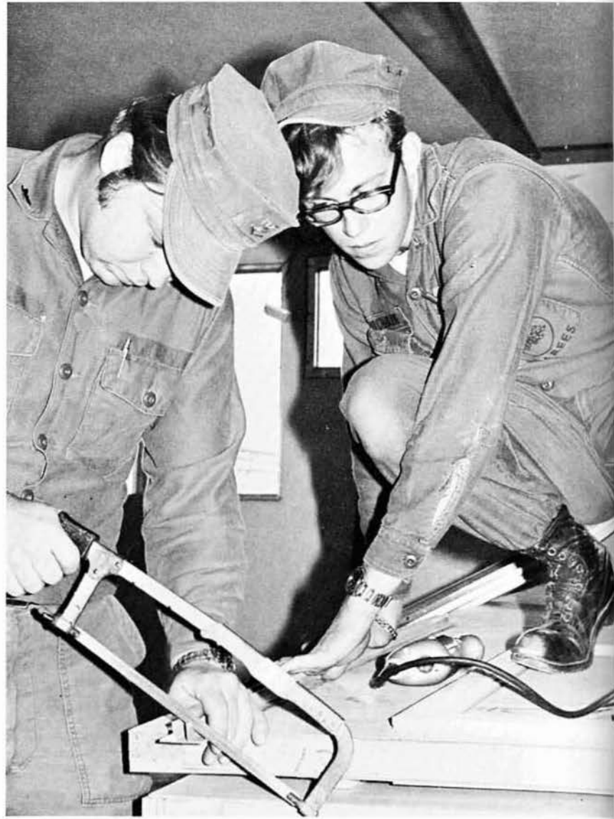
Builders WILLIAMS and BUCHANAN cut overhead T-bar.
