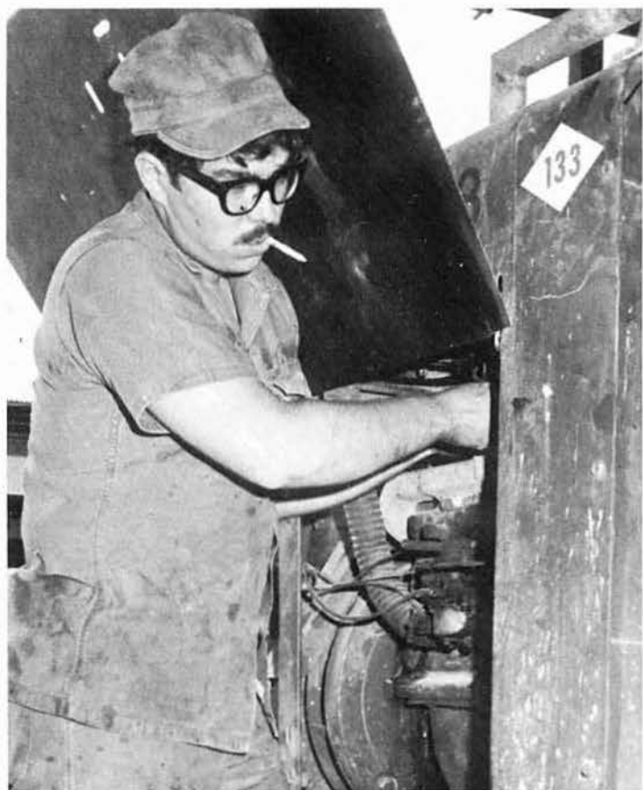
Replacing a fan belt to cool down a generator is CMCN HANLAN.
