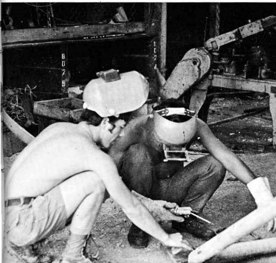
Welding a backstop angle are SW3 STEWART and trainee.
