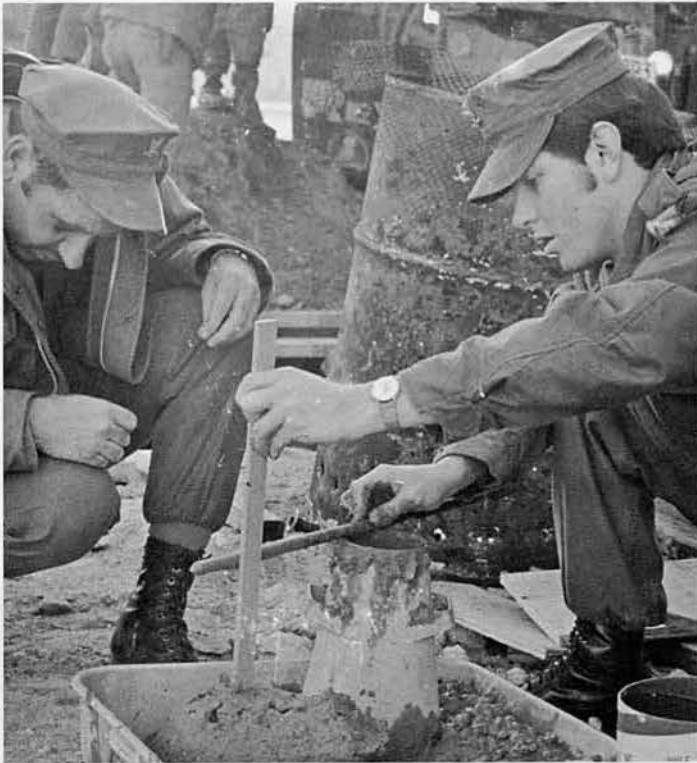
MEAD AND KELLY TESTING THE CONCRETE.
