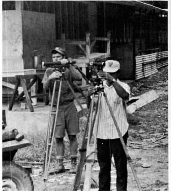
TRAINEE UNDER SUPERVISION BY TEAM MEMBER SETS ELEVATION.
