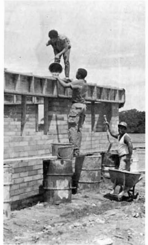
FILLING OF CONCRETE ON FORMS AS WORK ON UTWA DISPENSARY PROGRESSES.
