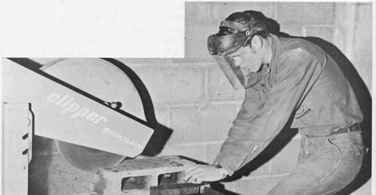
CONCRETE BLOCK CUTTER BUCN KIMBALL DOING HIS THING AT THE COMPUTER ROOM.
