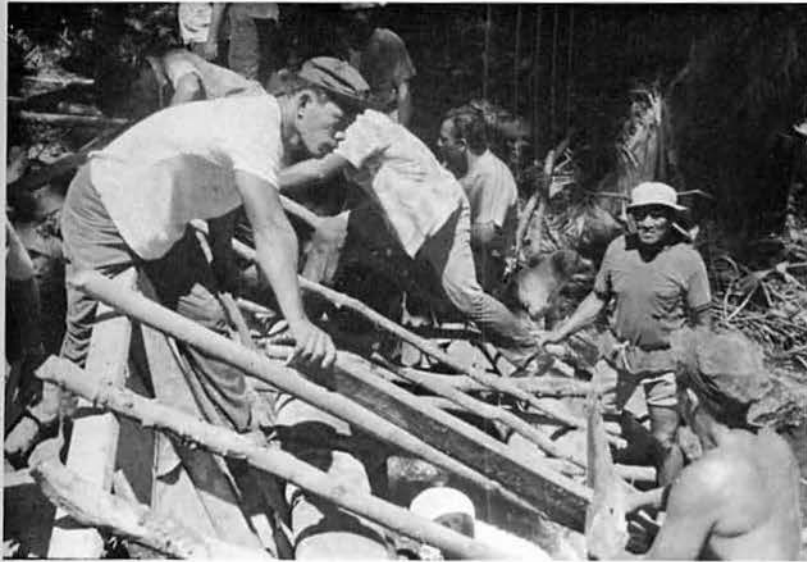
TEAM AND TRAINEES WORK TOGETHER ERECTING A WATER CATCHMENT.
