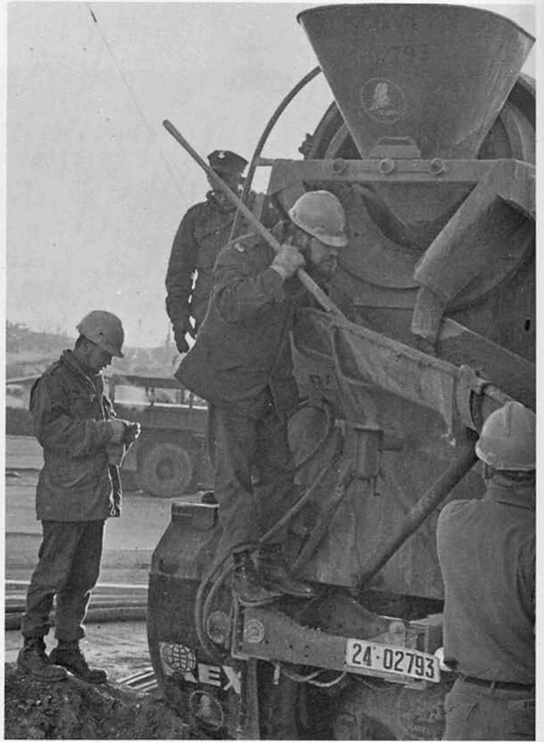
MORE CONCRETE FOR THE SCHOOL.
