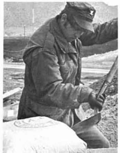
CONCRETE BY THE BAG FULL.
