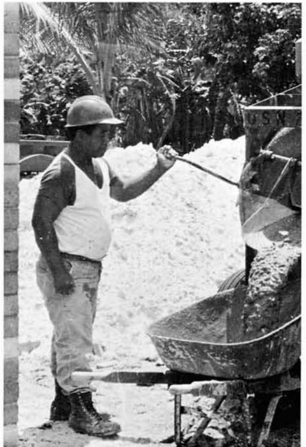
TRAINEE OPERATING MIXER DURING WORK AT UTWA DISPENSARY SITE.
