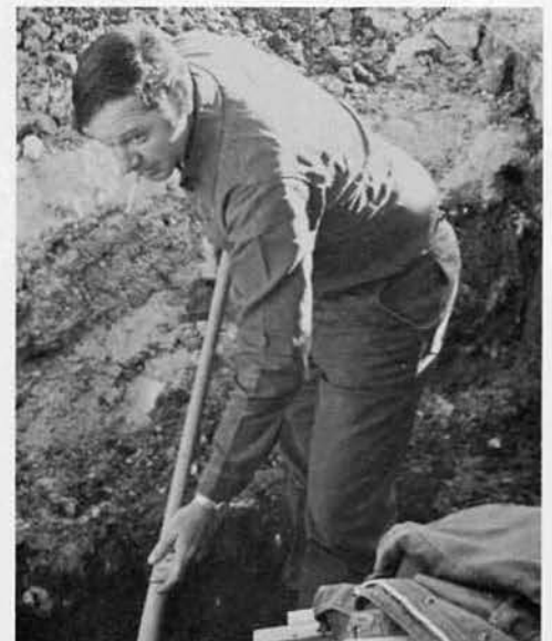
EA3 MEAD DIGGING FOOTERS AT THE GYM.
