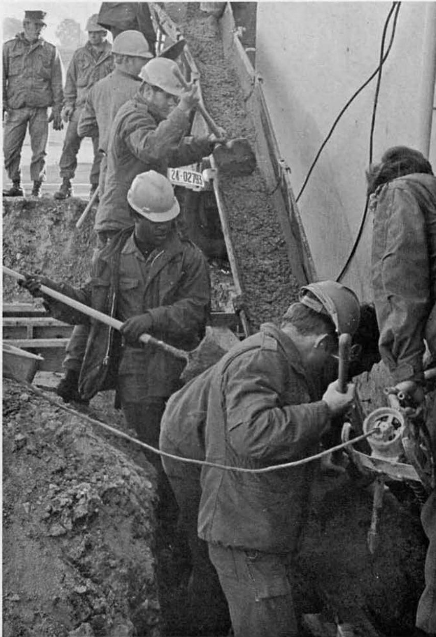
CONCRETE DAY AT THE GYM.
