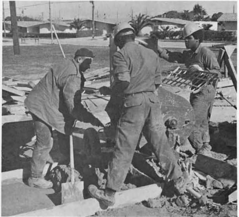
THE GYM EXTENSION MORTAR CREW TURNS TO.
