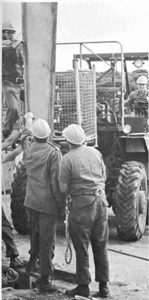
KANGROO MEN BUILDING A NEW SHED FOR MLO.
