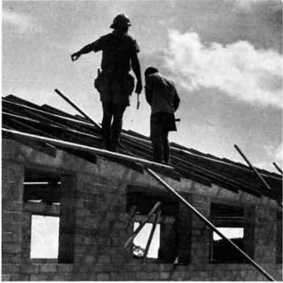
WORKING ON ROOF TRUSSES AT UTWA DISPENSARY BUILDING.
