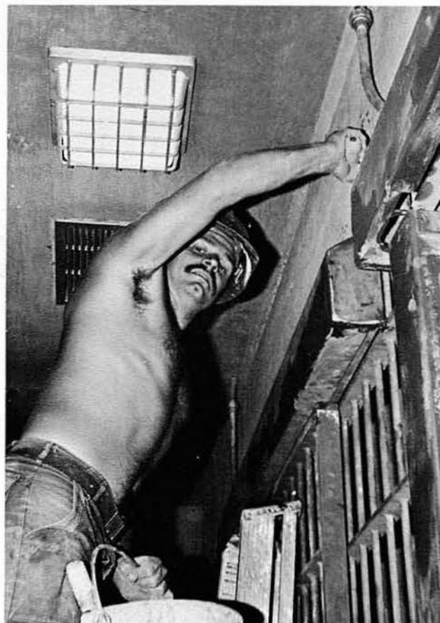
CN Bennington preparing the secret escape hatch.
