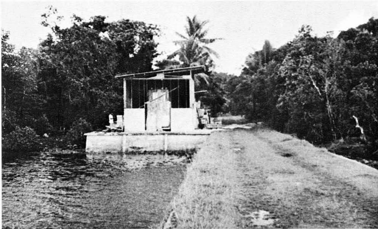
Ngeremnglui Ice Plant
