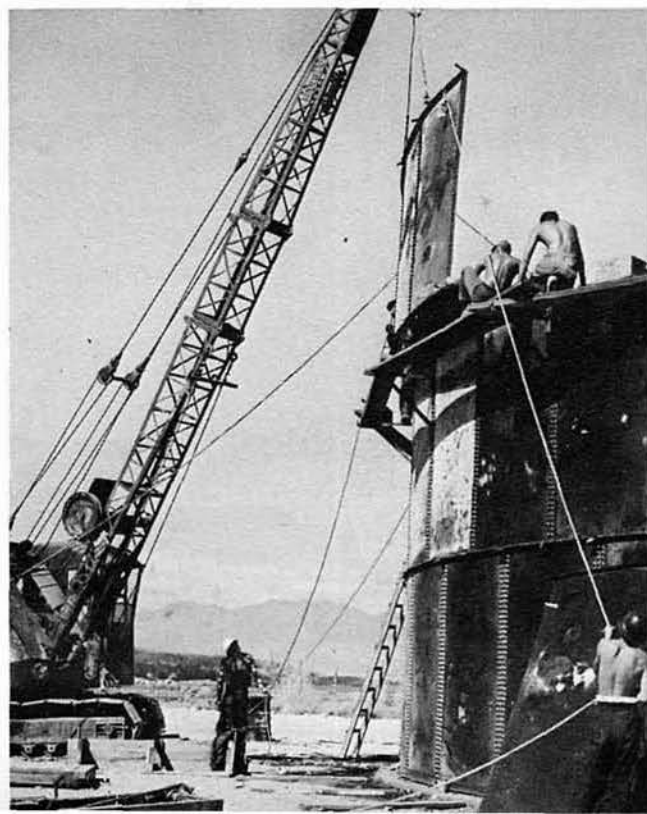
Works goes ahead at the tank farm
