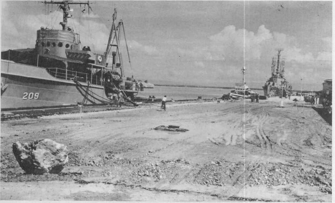
Wharf Baker old paving removed
