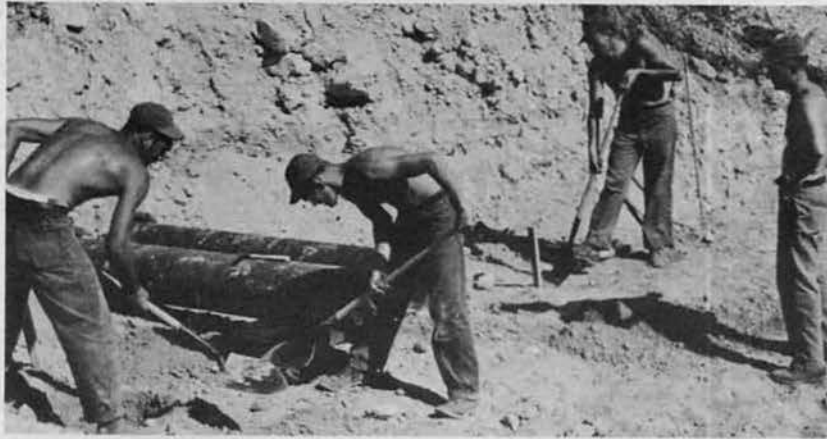
Laying Drain Pipes
