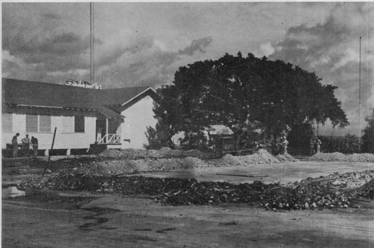
Site of Addition
