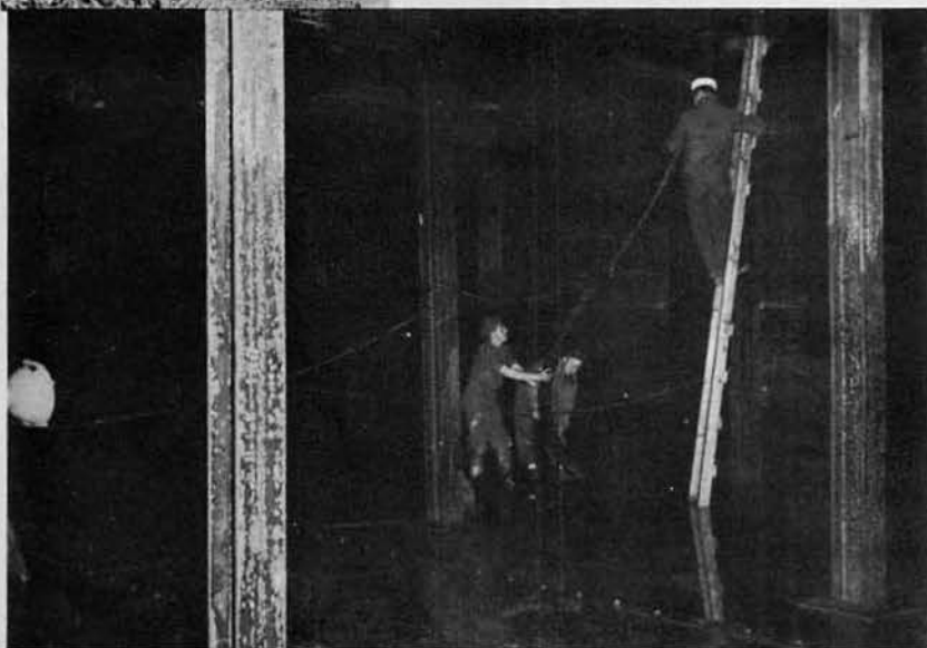
Jet Fuel Tank
