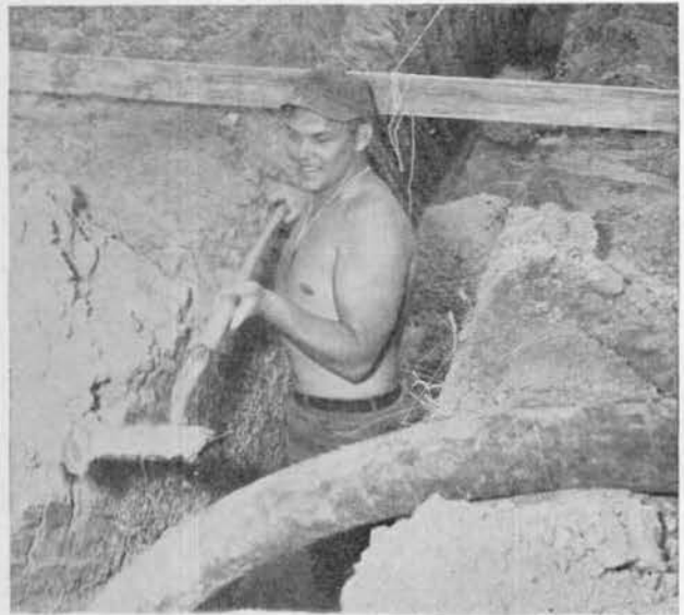
Digging in utilities at the Service Station.
