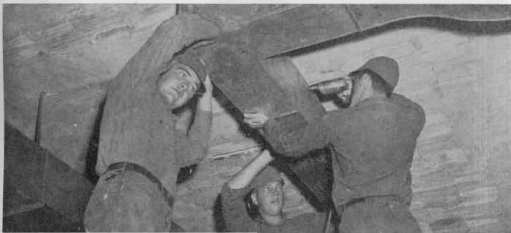
Installing the interior heating system at the Hobby Shop.
