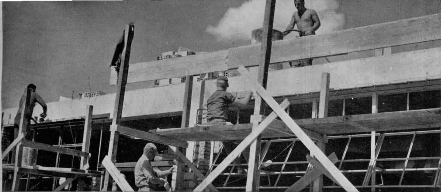
The brick laying crew keeping the mortar flying.
