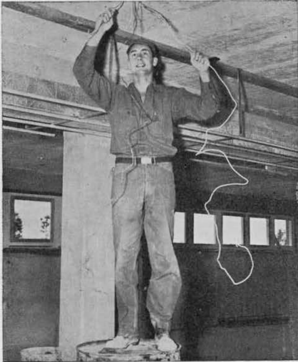
L. F. DOW does some interior wiring at the Library Project.
