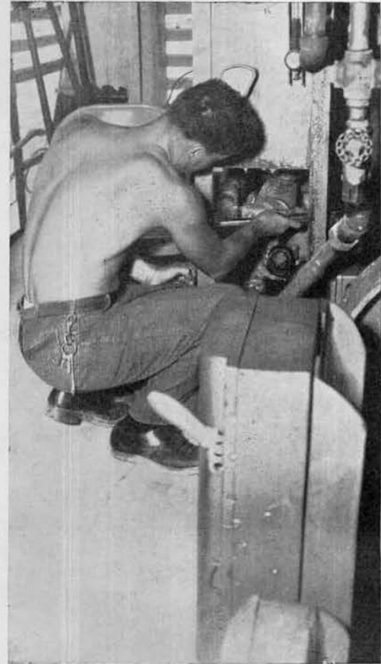
Fixing the Galley steam boiler.
