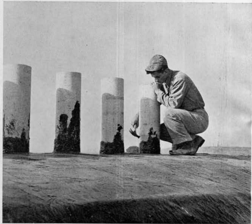
Above: Installing exhaust ports.
