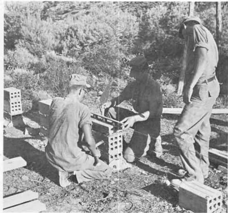
A little off-duty construction work. MOLINE, BROWN, and MOORE level blocks for an orphans' building.
