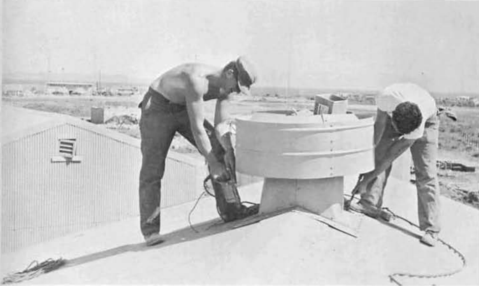
1600 : BOLT ON ROOF AND ATTACHMENTS
