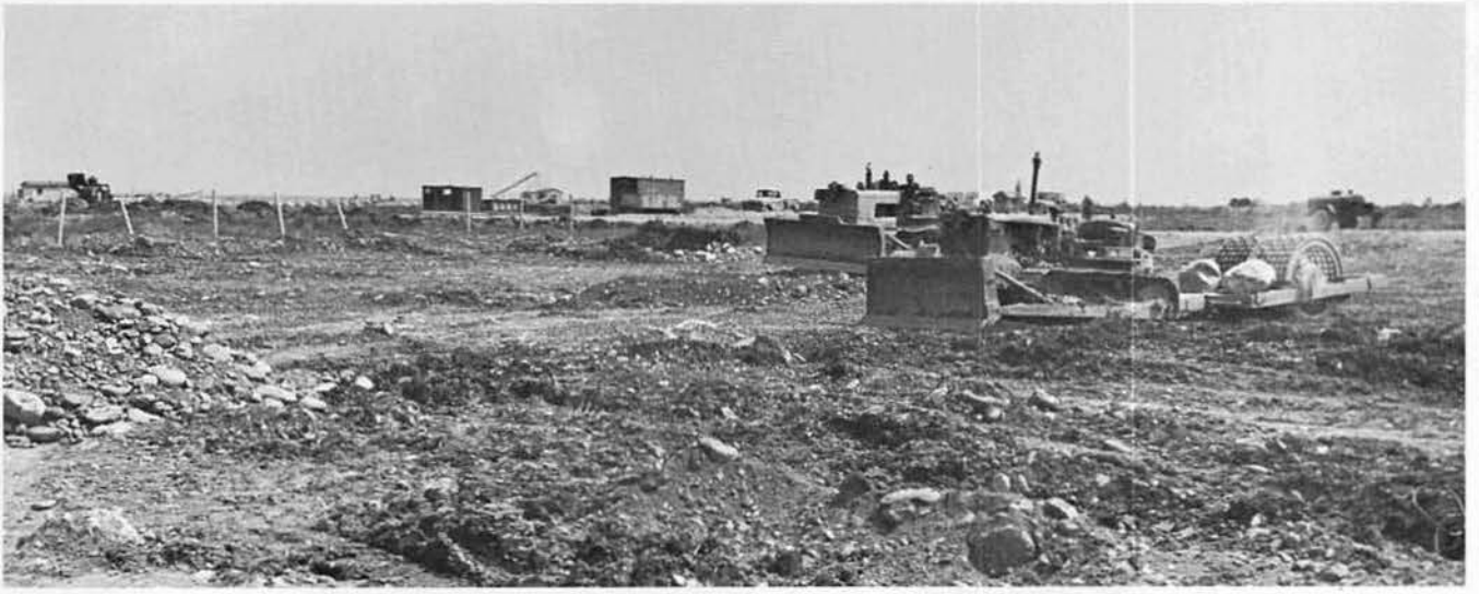
Fill and Haul and Fill and Compact and Fill—
