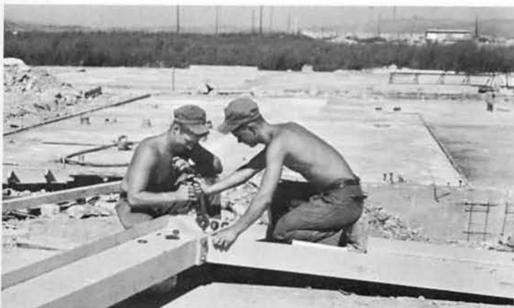
0900 : PREFAB COLUMNS AND BENTS
