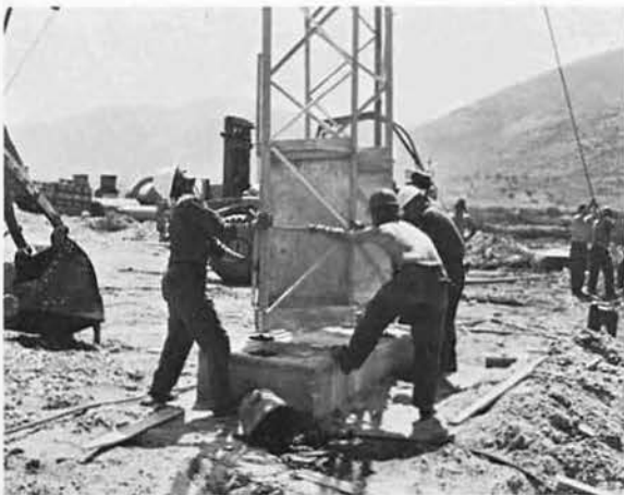
Tell DEBERRY we're not driving piles!
