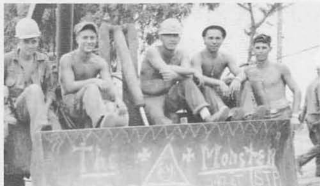
STEEL WORKER LINE UP FOR INSPECTION.
