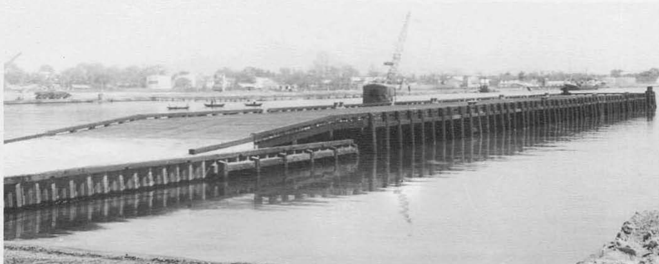
LCU/LCM RAMPS AND 300 FOOT TIMBER PIER COMPLETED
