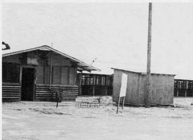
NSA SENTRY DOG KENNELS DOG HANDLERS QUARTERS AT LEFT. BUILT BY D CO.
