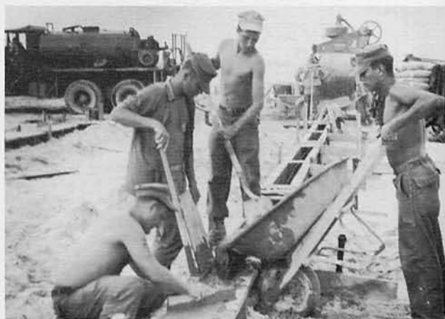
POURING A CONCRETE FOUNDATION AT THE "POW" CAMP
