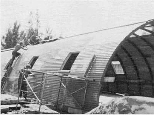
'C' CO AT WORK ERECTING SHIPS STORE AT CAMP TIEN-SHA
