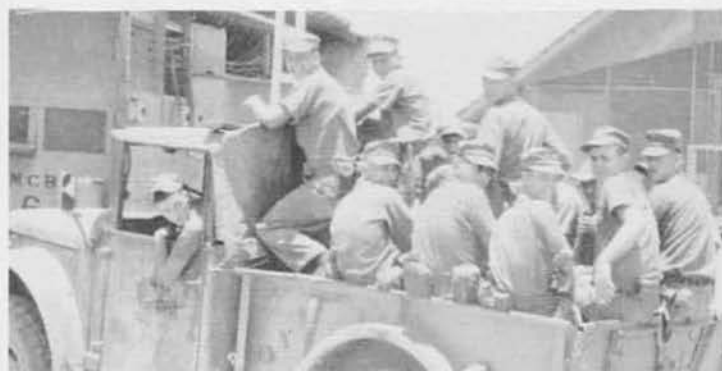
STEELWORKER'S TWENTY MAN BUS
