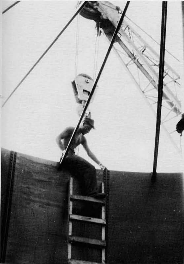
VIEW OF PARTIALLY COMPLETED 3000 BARREL WATER TOWER AT CAMP TIEN-SHA
