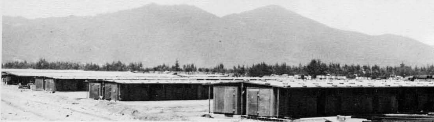
VIEW OF REEFERS AND ROAD WORK AT COVERED STORAGE DA NANG.
