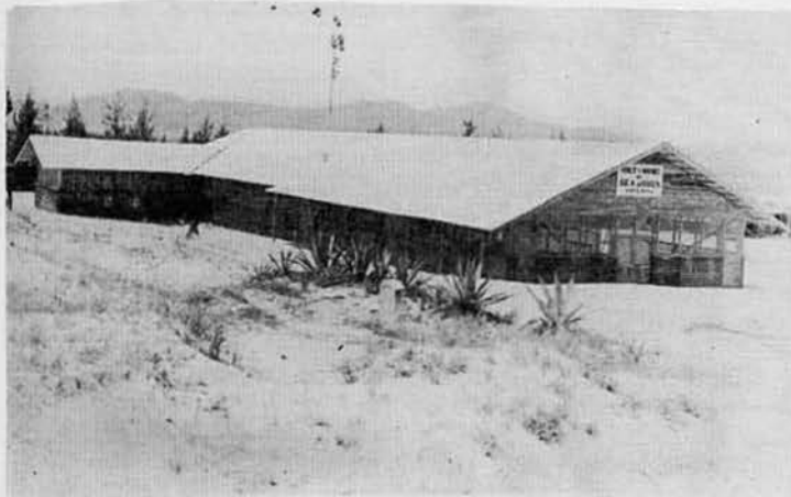
A NEW EATING PLACE --This completed 500 man galley for 3/1 Marines outside Da Nang is just one of several built by the Seabees of MCB-6 and other units.
