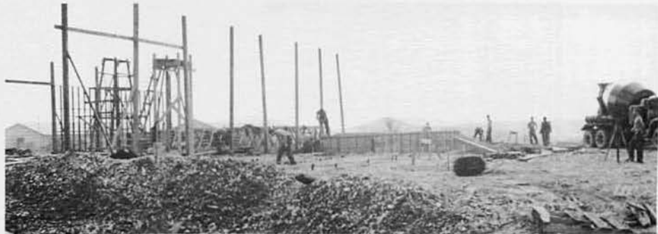
'C' CO AT WORK ON MAINTENANCE FACILITY AT 5TH SPECIAL FORCES
