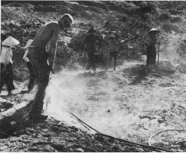
DRILLING ROCK FOR CAMP TIEN-SHA LAUNDRY
