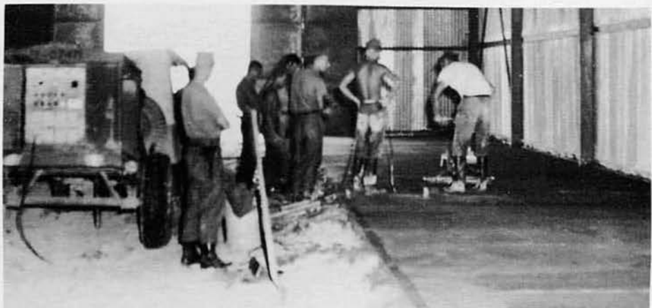
'C' CO FINISHING CONCRETE PAD AT 5TH SPECIAL FORCES
