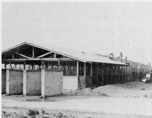
NSA SENTRY DOG KENNELS VIEW OF PARTIALLY CONSTRUCTED ROOF D CO
