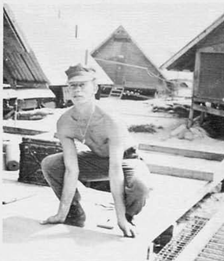
ARE YOU SURE THE WALLS GO HERE?
