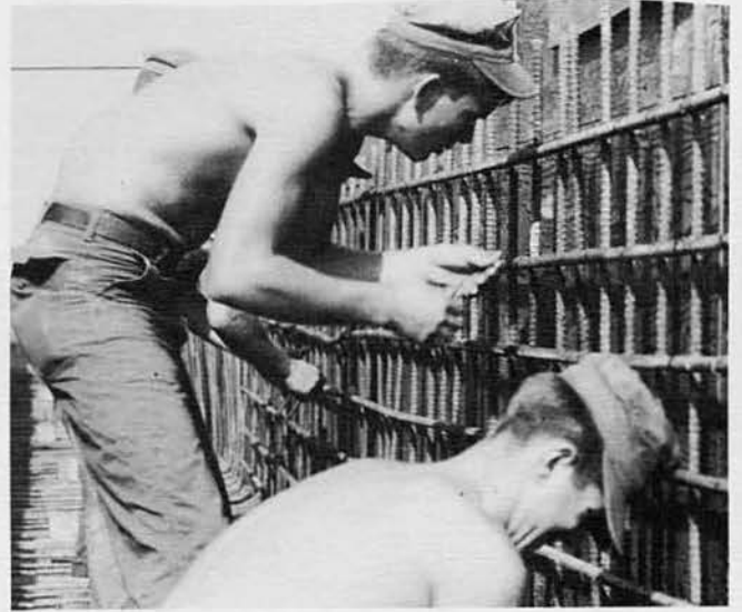
C CO STEEL WORKERS TYPING RE-INFORCING STEEL ON DRAINAGE DITCH SYSTEM
