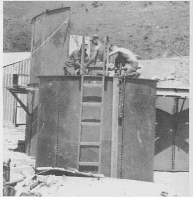
'C' CO STEEL WORKERS ERECTING TANK AT CAMP TIEN-SHA
