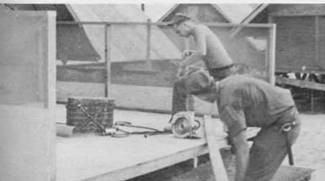
BRAVO BUILDERS WORKING ON THE EXTENSION TO THE SOG HUT
