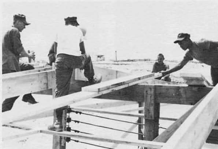
C CO SETTING RAFTERS OVER REEFERS AT COVERED STORAGE.
