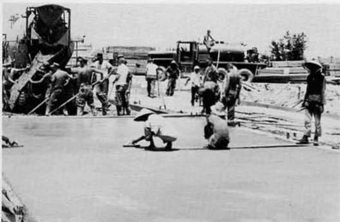
'C' CO POURING REEFER SLAB WITH VIETNAMESE ASSISTANCE AT COVERED STORAGE.
