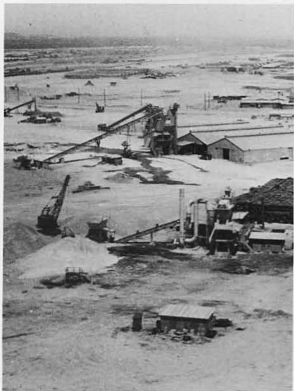
Six's crusher operation
