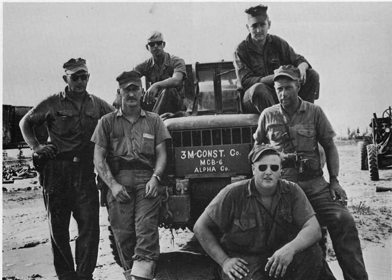
Alpha Company's detail at Tien Phouc
