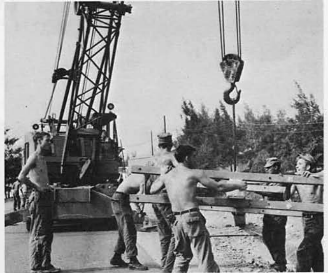
The power poles go up
