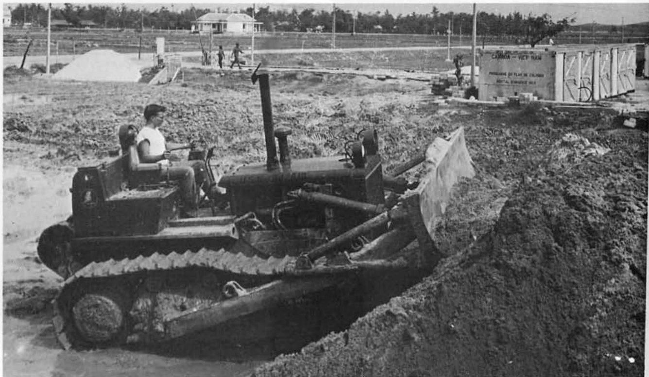
Moving earth the Seabee way
