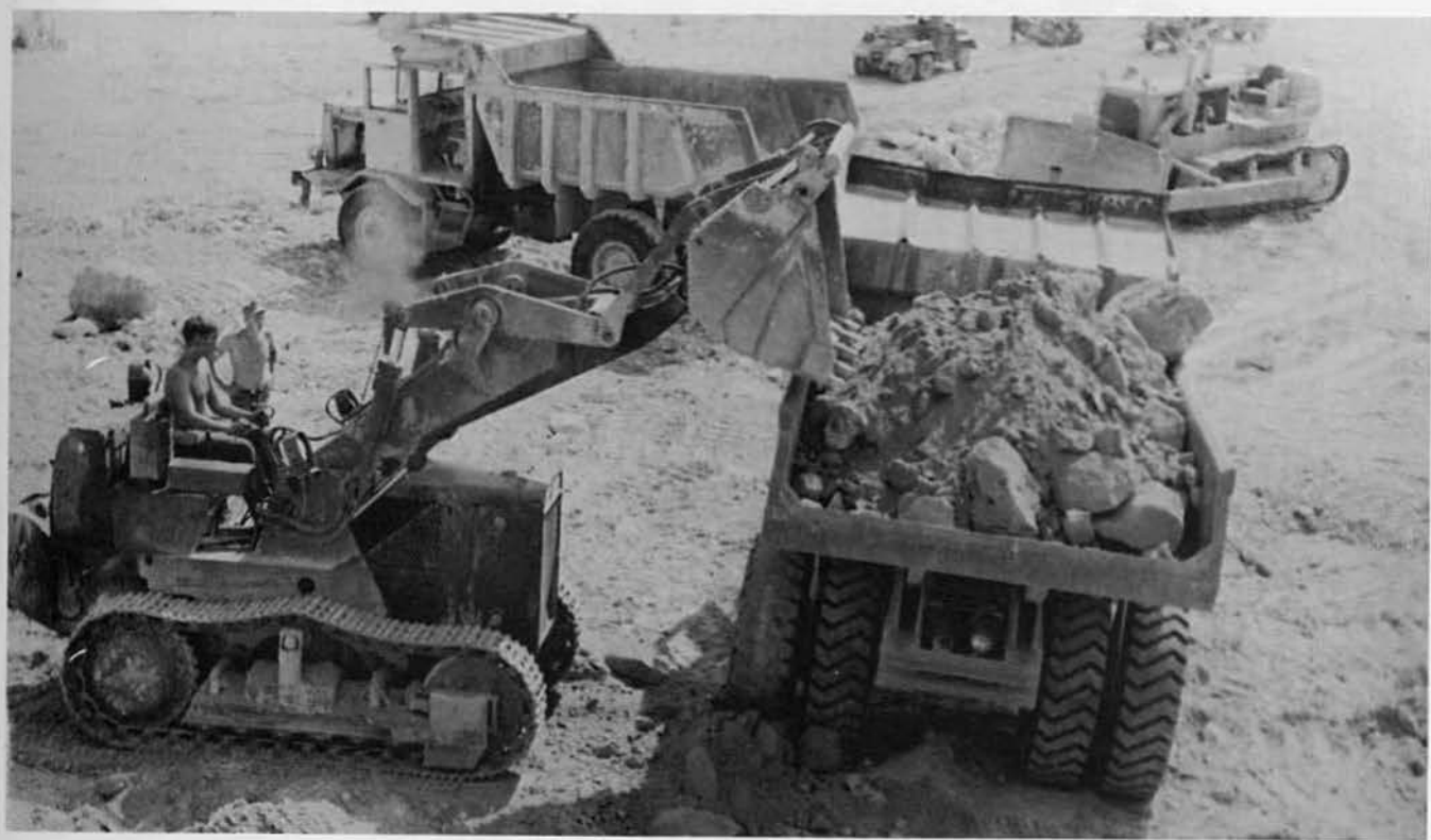
Loading boulders to feed the rock crusher
