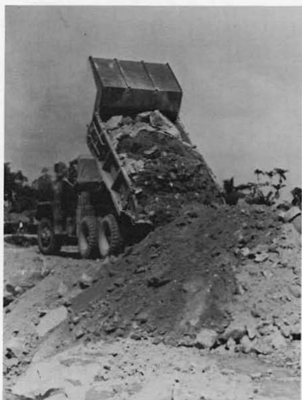
Fill-in work along Route 1
