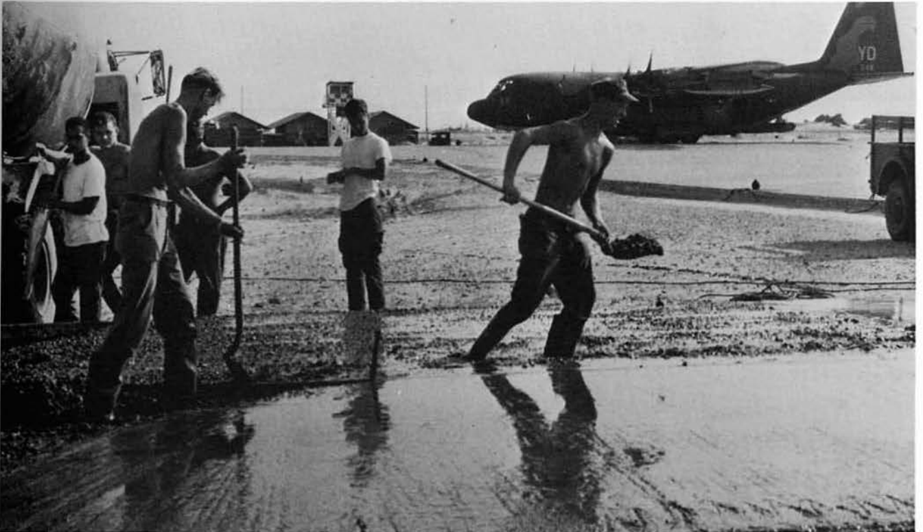
Concrete is our specialty
