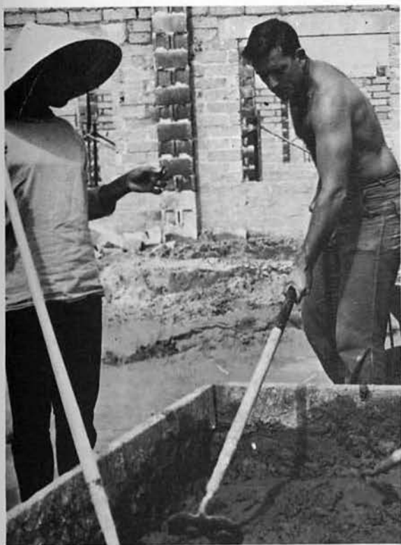
Mixing mortar
