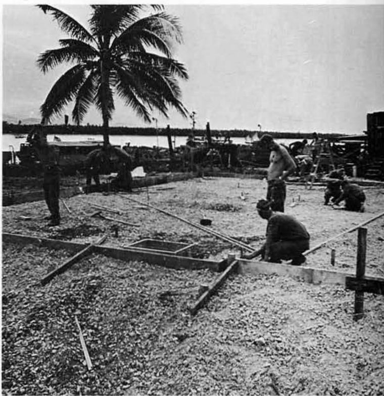
First, the foundation...
