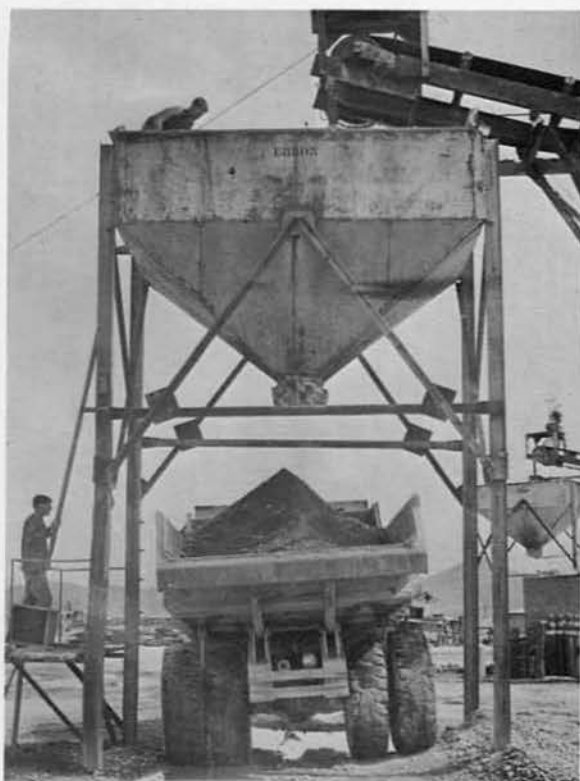
Loading a truck at the crusher
