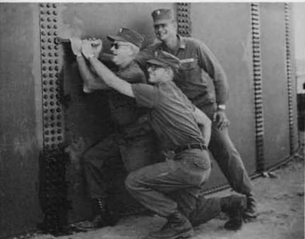
Some high-level work on a POL tank
