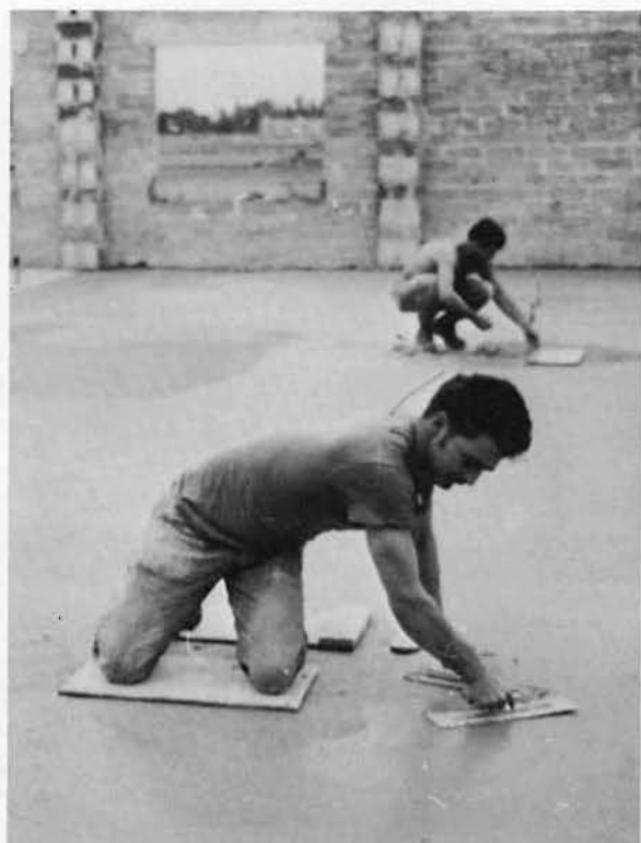
Smoothing the floor
