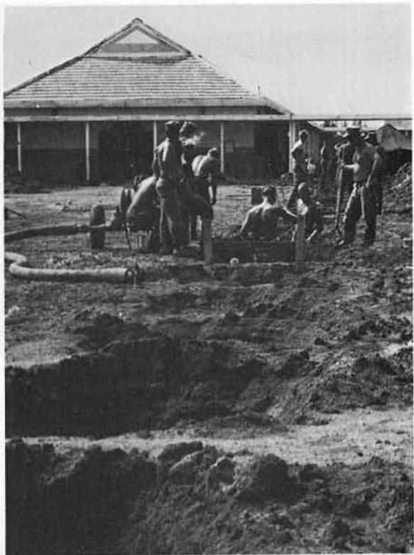
The foundation comes first
