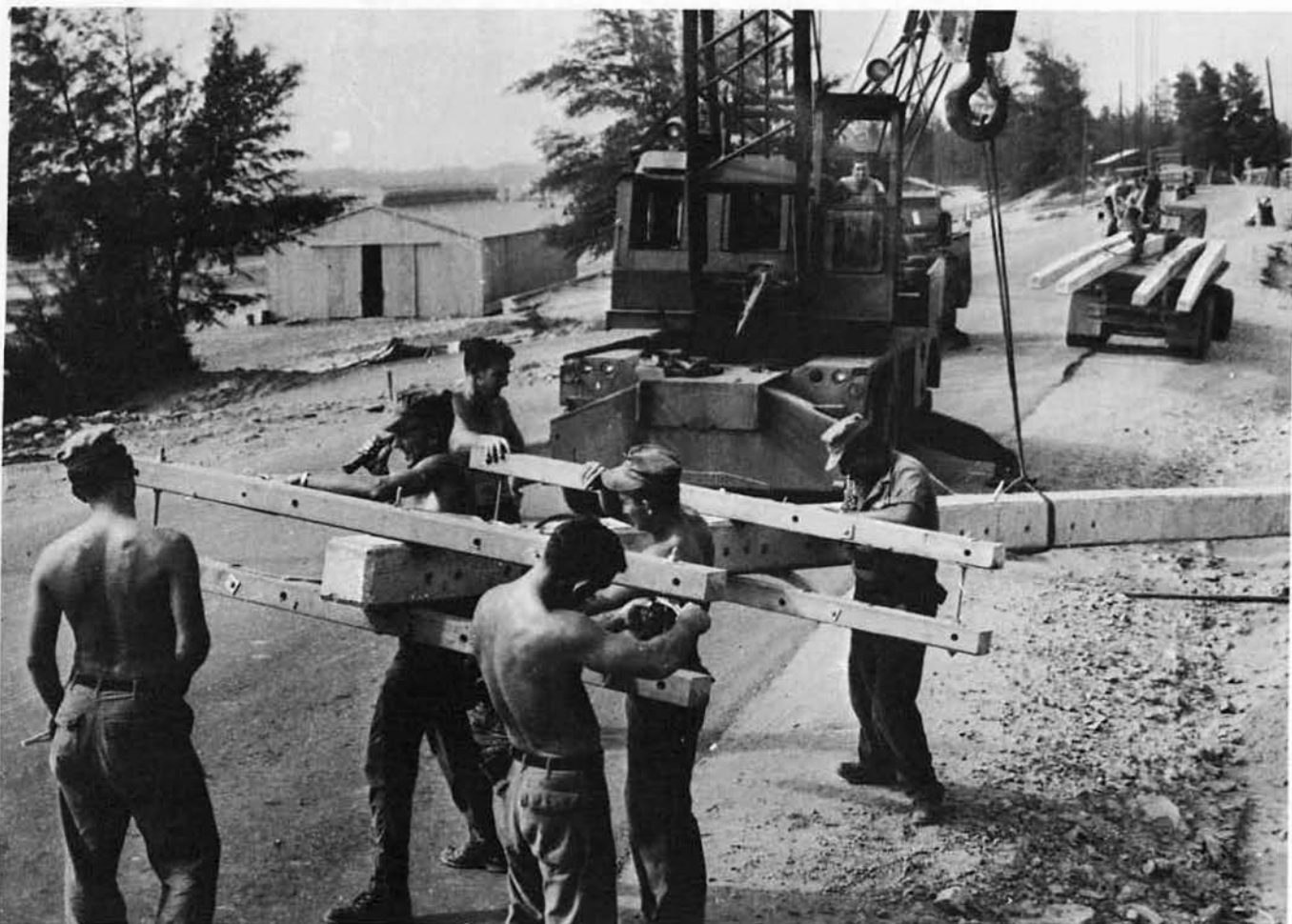
The poles go up
