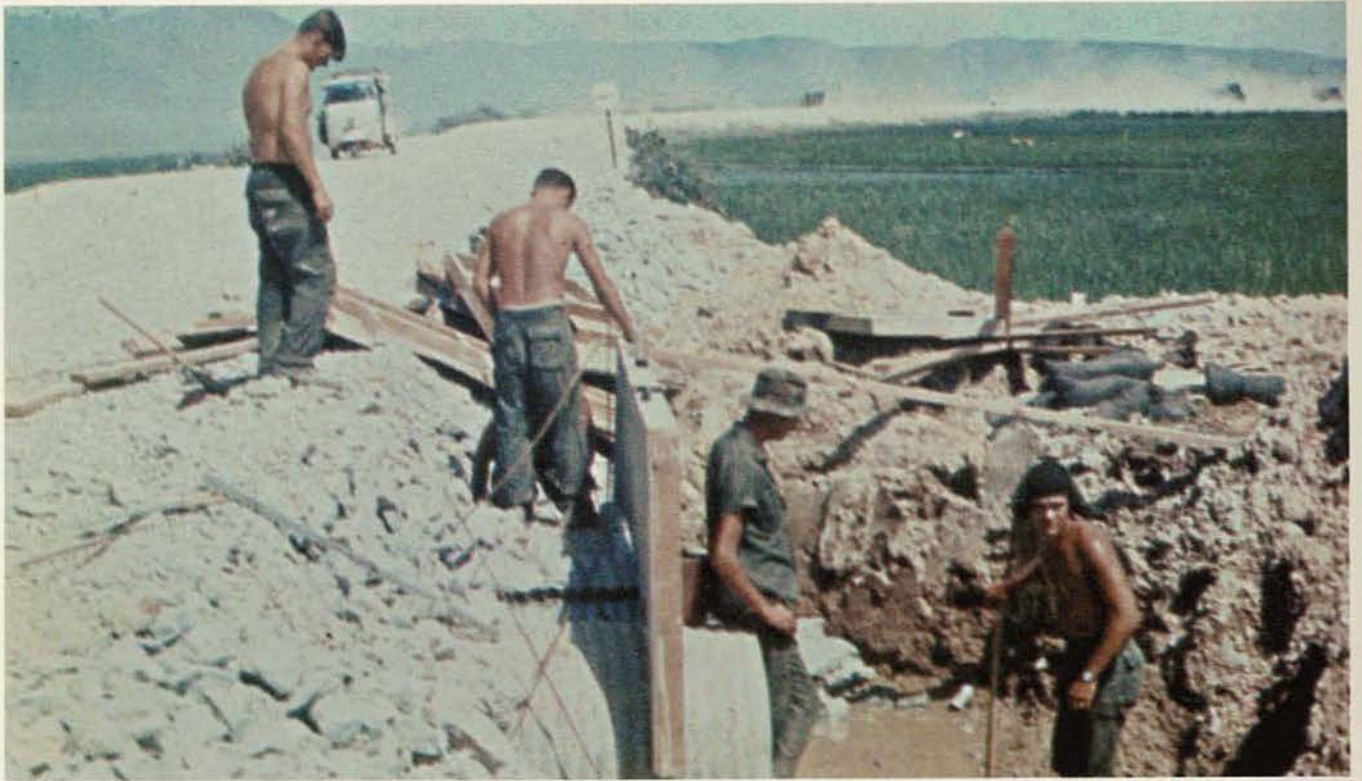
One of the culverts we built on Route 1
