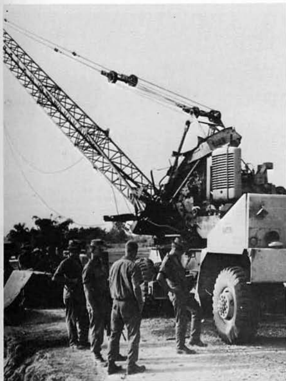
This damage due to VC -- not CM's
