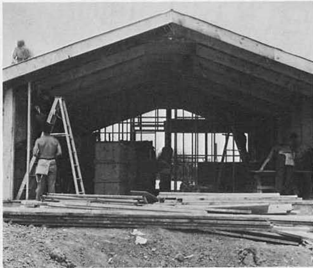
MAG 36 telephone exchange
