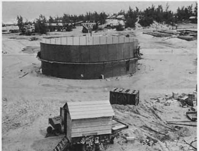
One of three oil storage tanks we built
