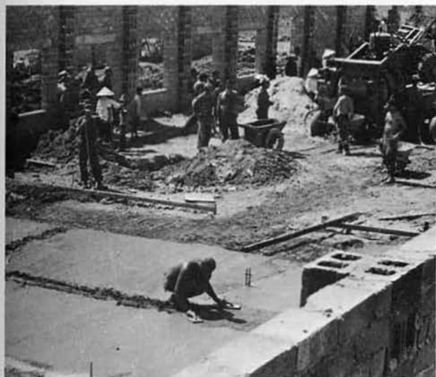
A floor for the hospital
