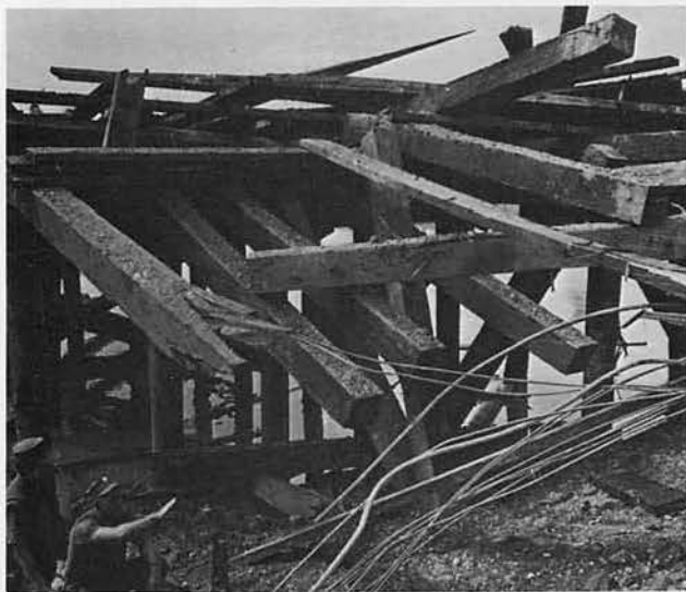
VC destruction at Bridge 13
