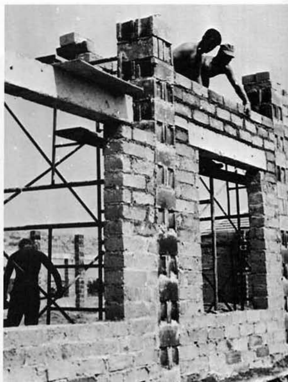
The walls go up
