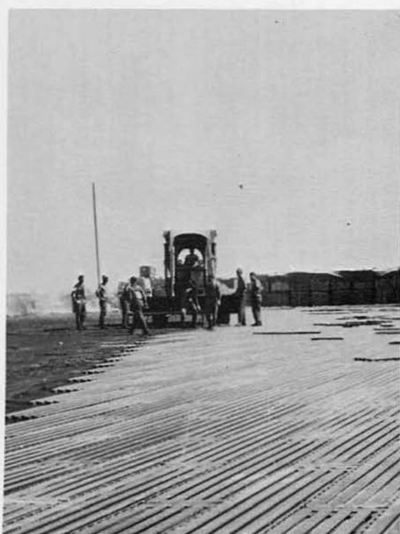
Laying matting at Class II and IV Storage
