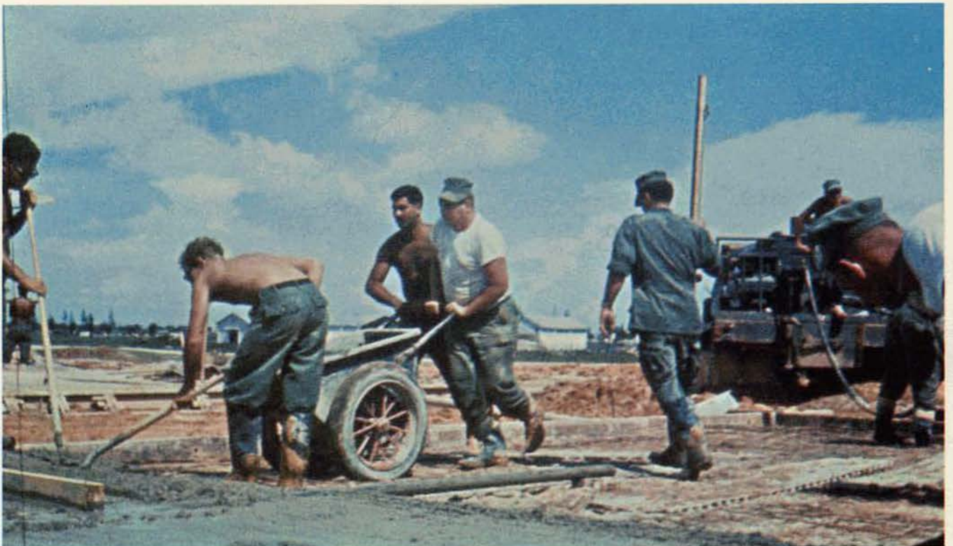
A solid building starts with a strong floor
