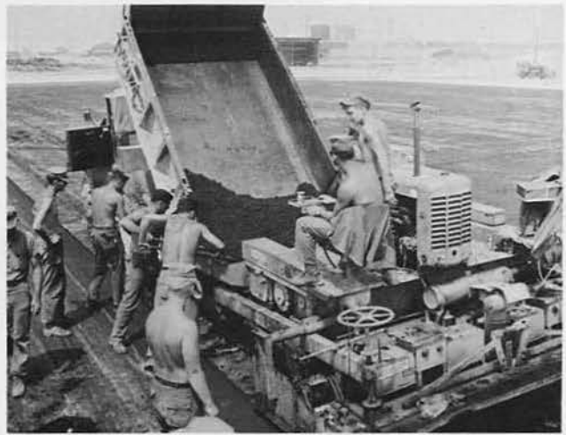
Laying asphalt at NSAD
