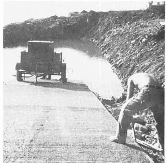
LAUNCHING RAMP NEARS COMPLETION
