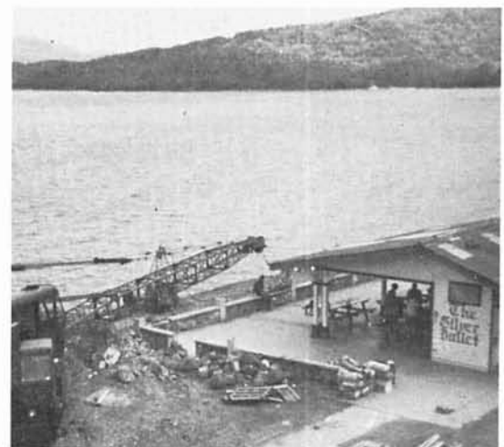
CONVENIENT SPOT FOR A JOBSITE
