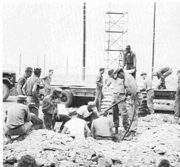
WORKING ON A TOWER FOUNDATION
