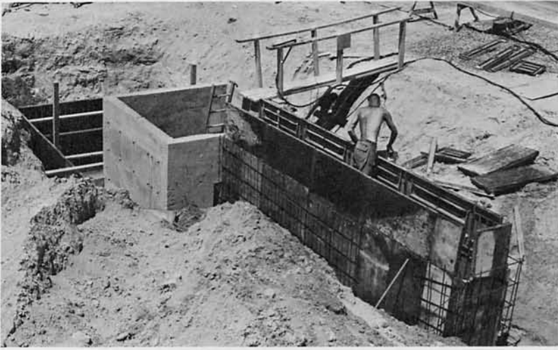
Placing steel forms for the spillway
