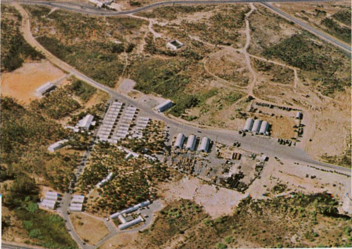
Silver City with the Acey Deucey (top) and office spaces (bottom)
