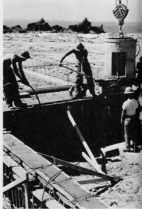
Pouring new foundations across the bay
