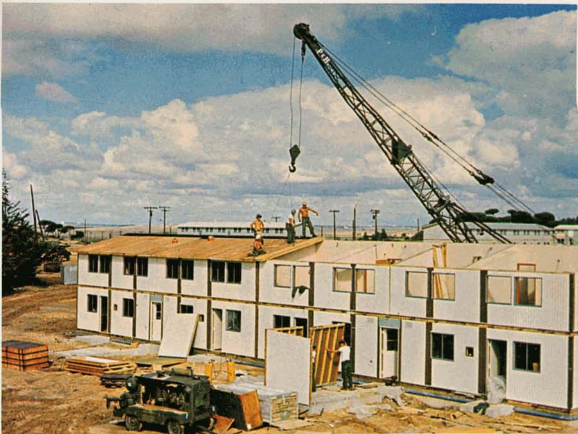
A typical fourplex is pieced together
