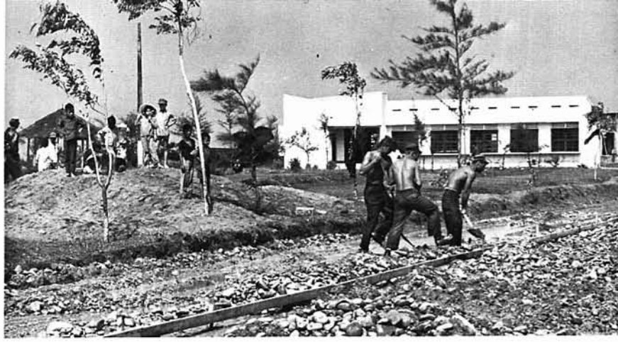
Builders place fill and pour concrete for Vietnamese housing job.
