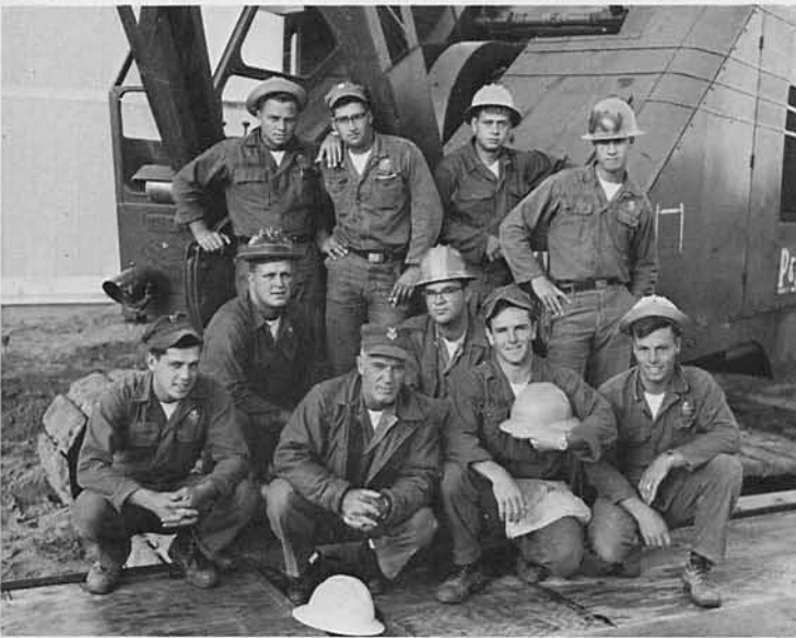
The first erection crew was under BU1 Carl Dube.
