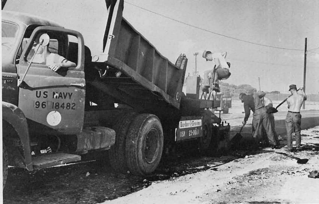
Paving the main road
