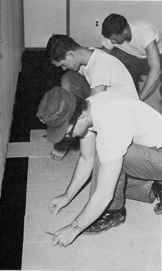
Measuring "cold cuts"
