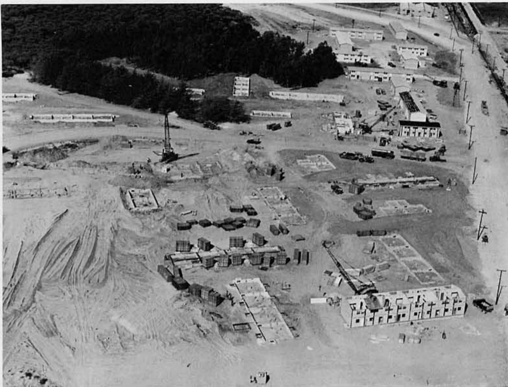
Area D reaches the erection stage.
