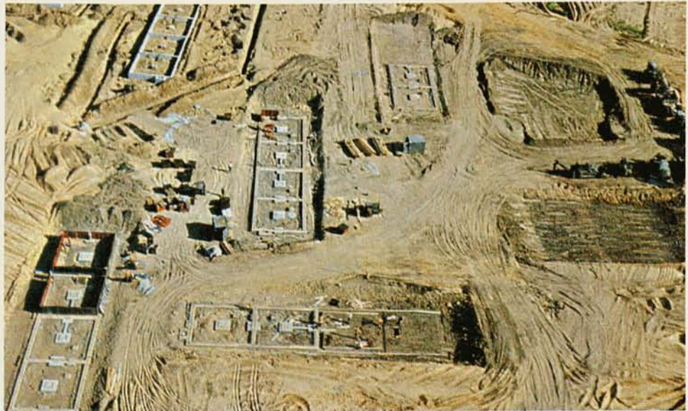
The Battalion completed the foundations in F&G areas.
