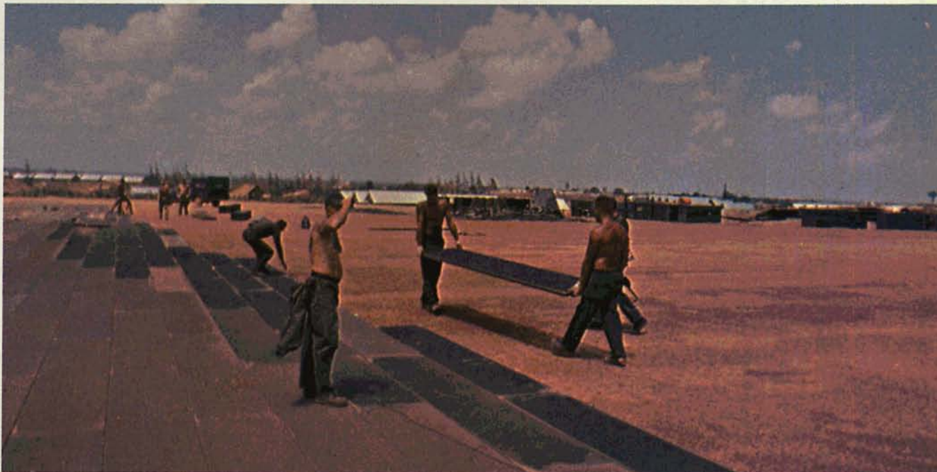
Dong Ha airstrip takes shape as interlocking AM-2 matting is laid down.
