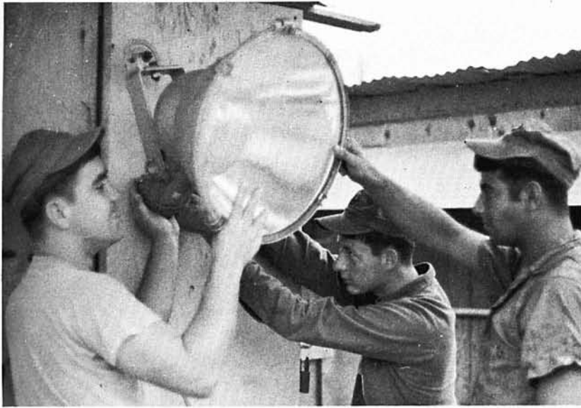
CONSTRUCTION ELECTRICIANS — CE2 D. C. Metell, CECN E. L. Scott, Jr., CE2 R. C. Fulcher.
