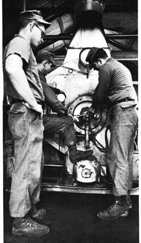
BOILER PLANT WATCH — CE3 L. A. Houman UTCN D. A. Russell, UT3 J. E. Connelly.
