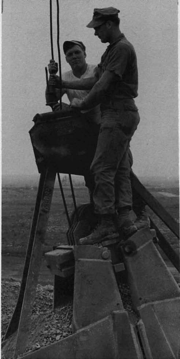
BATCH PLANT — SWCN R. H. Pitman, CN W. E. Leland.
