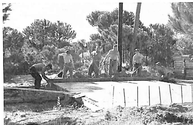
MEN OF OUR ADVANCE PARTY PUT FINISHING TOUCHES ON CHAPEL DECK...
