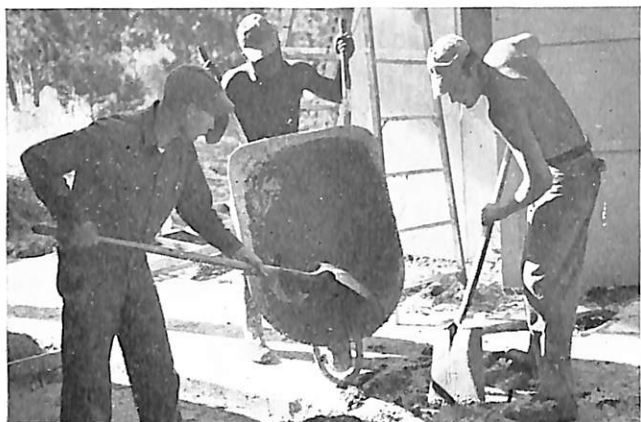
MEN OF ADVANCE PARTY WORK ON CHAPEL DECK
