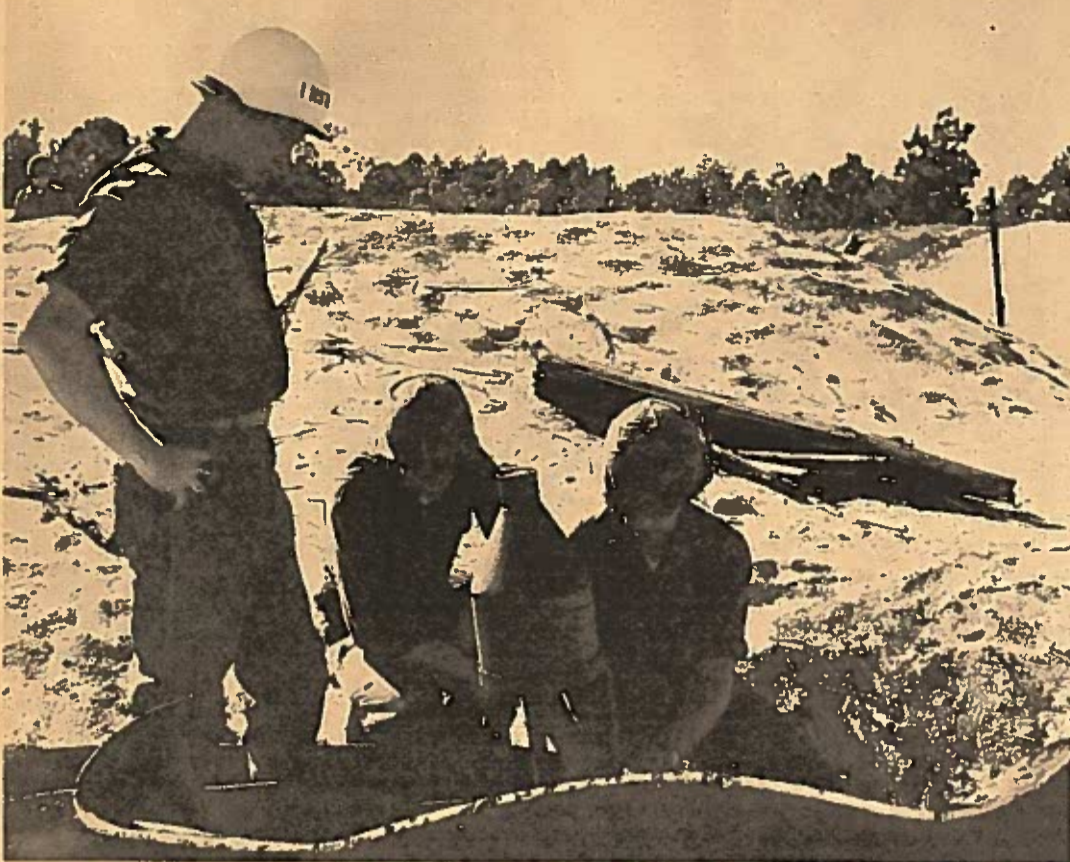
Under the justifiable close observation of their instructor, Constructionman James D. Flory, center, and Lt. Carl E. Christenson keep on as friendly terms as possible with 40 pounds of high explosive as they prepare to cut a steel beam the easy way.
