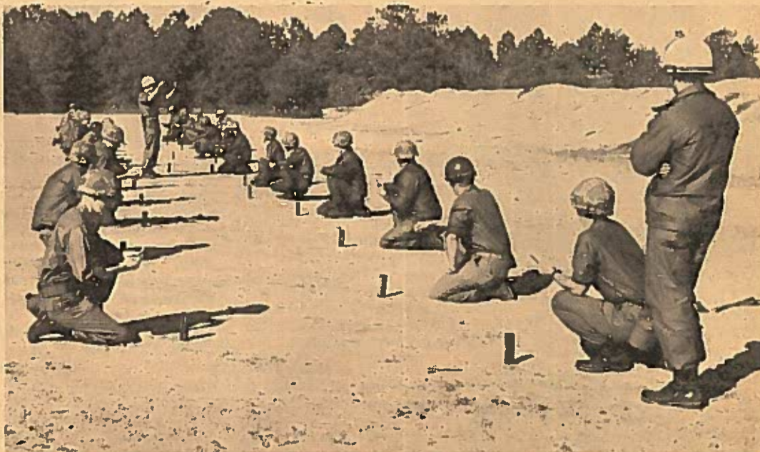
Seabee and Marine students learn together in the 2d Engineering Battalion Demolition and Mine Warfare School. Here, a "leapfrog" charge is prepared.
