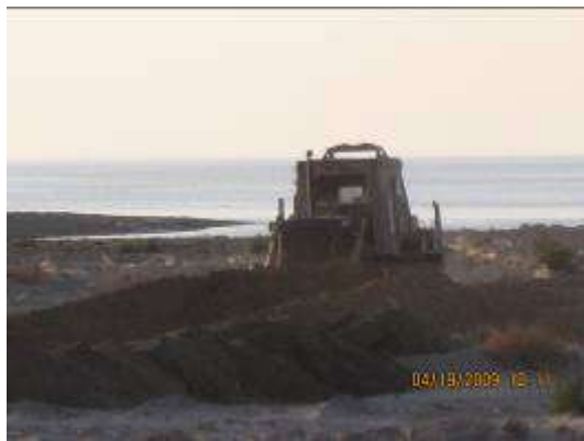
Dozer moves earth for roadway
