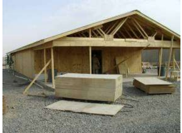
Exterior of one of the Buildings
