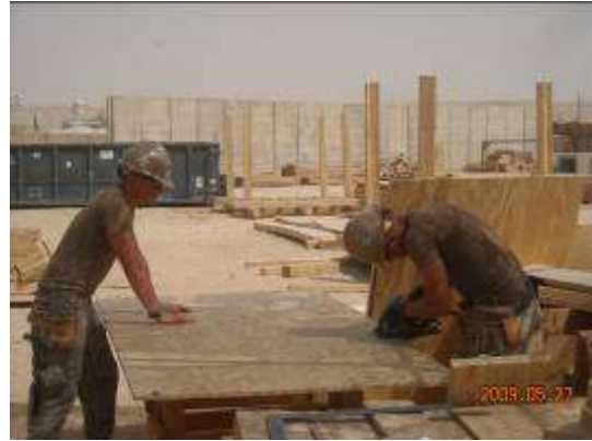
Prefab wall panel construction underway
