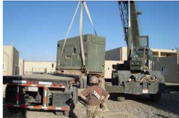
Generator emplacement underway
