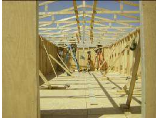
Seabees install trusses
