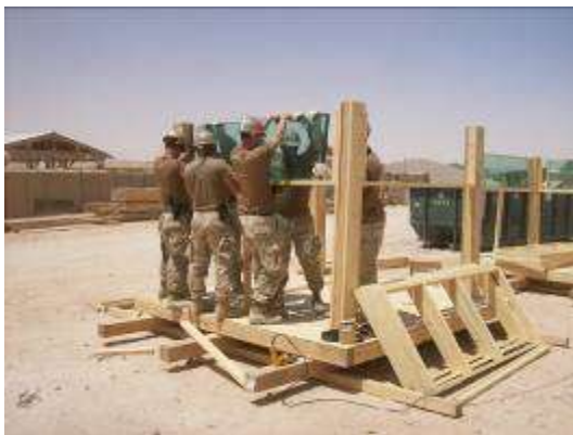
Bullet resistant glass install underway
