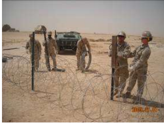
Concertina Wire installation continues
