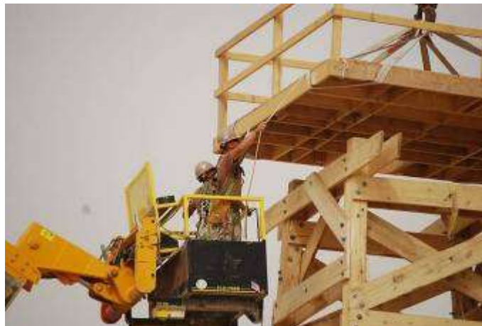
II MEF Fwd, JSTAR Timber Tower Erection
