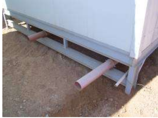
Piping installed at AB Unit
