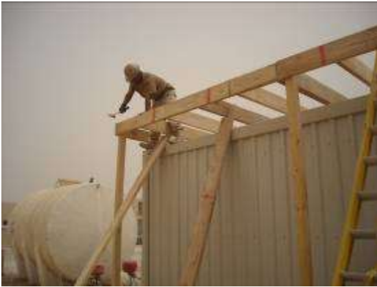
Shade shelter framing underway
