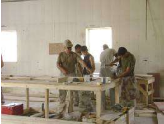
ISF learn floor truss prefab
