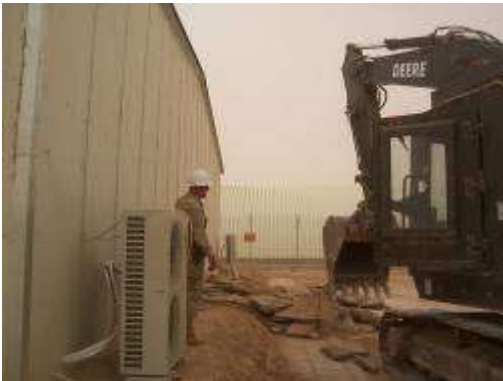
Demo existing walk for new loading pad
