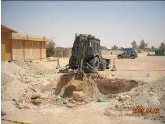
Backhoe digs foundation pit
