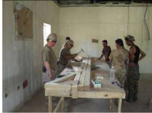
ISF learn floor truss prefab
