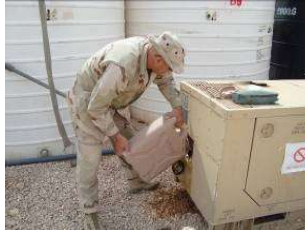
Seabee refills diesel generator
