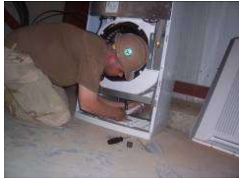
Air handler install underway
