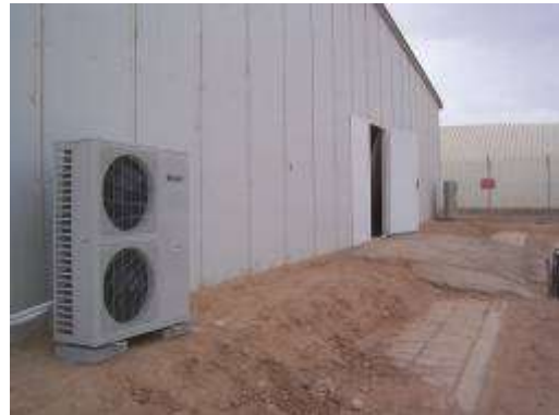
Concrete loading pad and A/C installed
