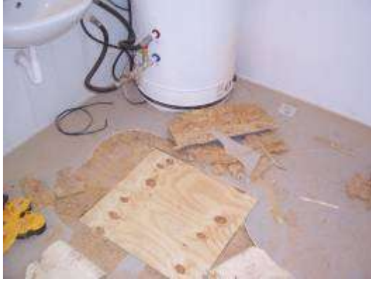
Repaired floor at water damaged area
