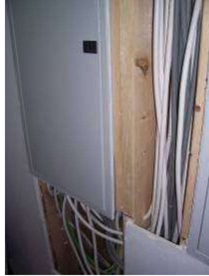
Wiring installed to panels
