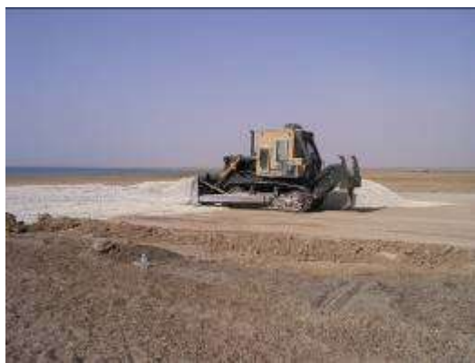
Dozer moves rock at equipment pad
