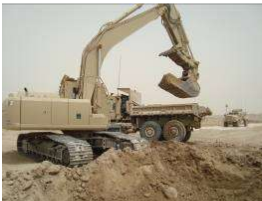
Excavator loads MTRV Dump
