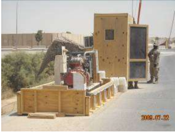
Generator and guard shack completed
