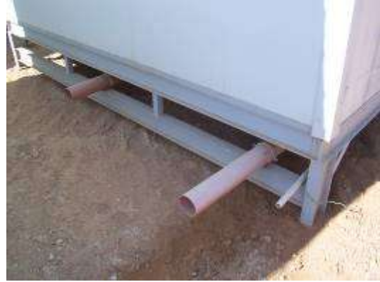
Drain piping installed
