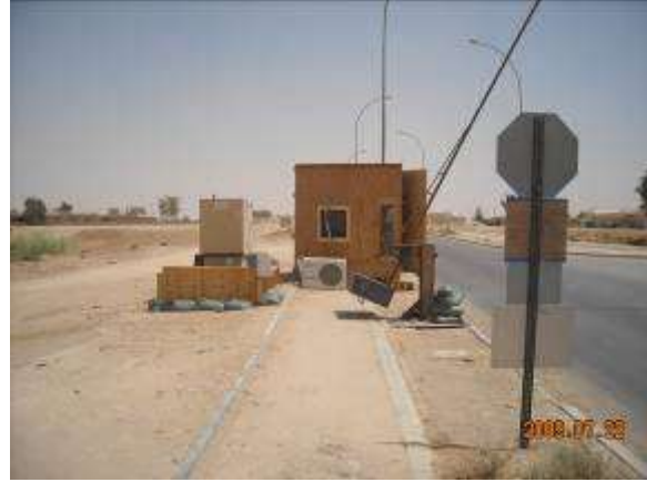
Guard shack, generator and gate
