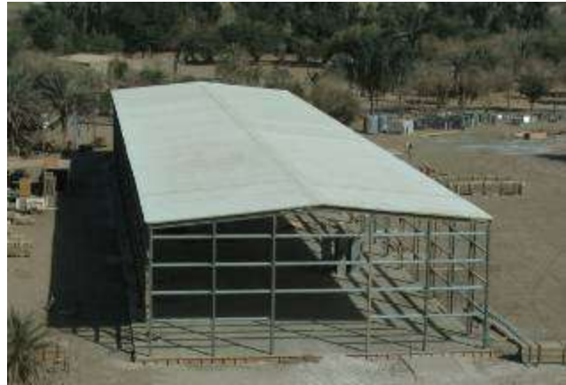
Steel Structure Erected
