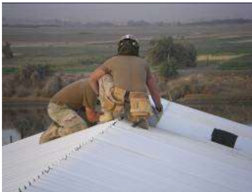
Metal Roof Panel installation
