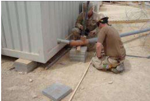
UT's install drain piping
