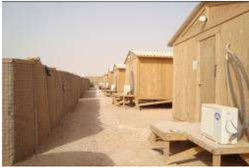
A/C Units and Steps installed at SWA Huts
