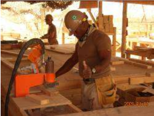
Gusset plate installation occurs
