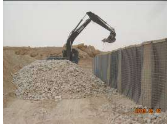
Excavator fills HESCOs with gravel
