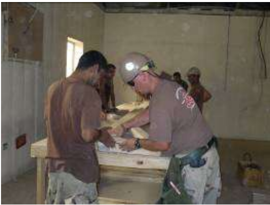
ISF learn floor truss prefab
