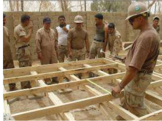
ISF view floor framing procedures
