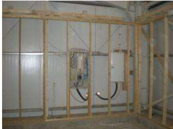
Interior electrical system roughed in
