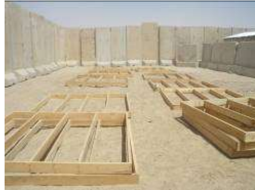
Prefabricated floor framing
