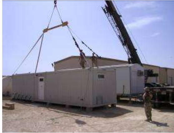
Ablution Unit being placed
