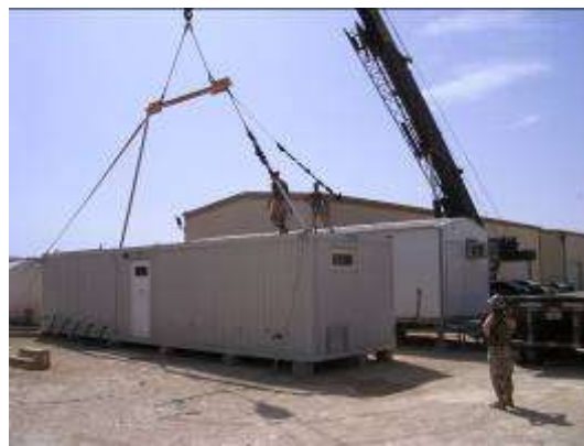
Ablution Unit emplacement underway
