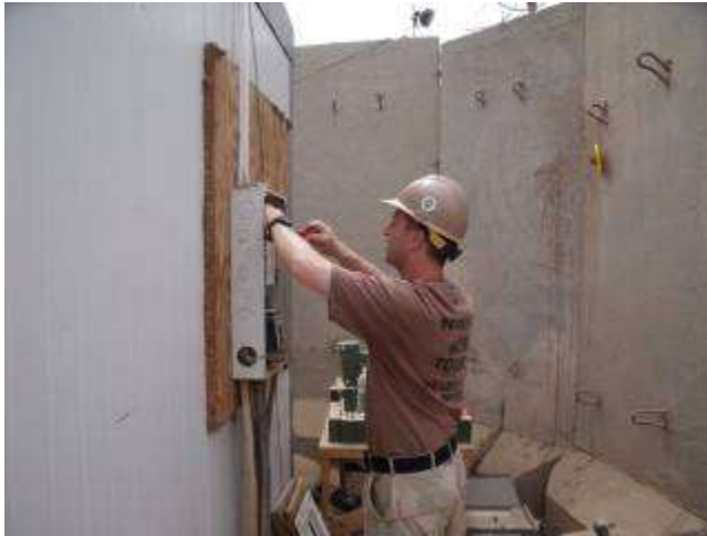
An existing panel is rewired correctly
