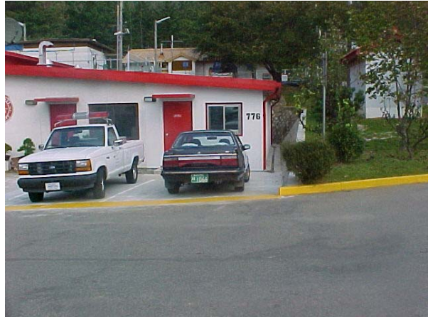
Front view of completed project.
