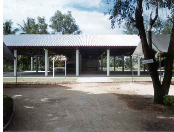
Left, completed canopy, Philippines. Below, completed school building project, Thailand.
