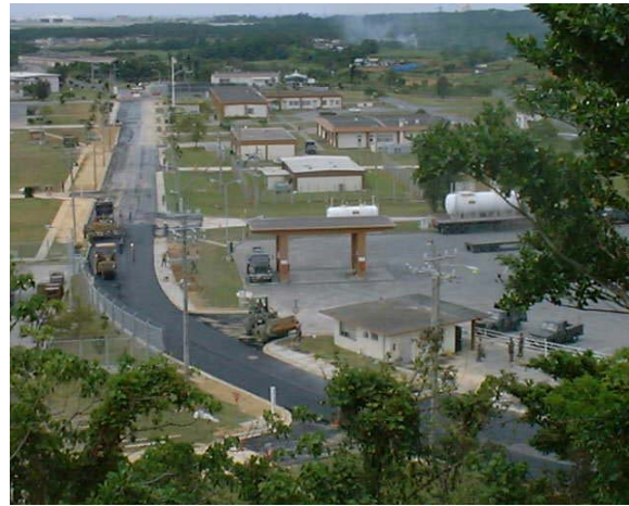
Right, spreading new asphalt onto existing road with asphalt paver.
