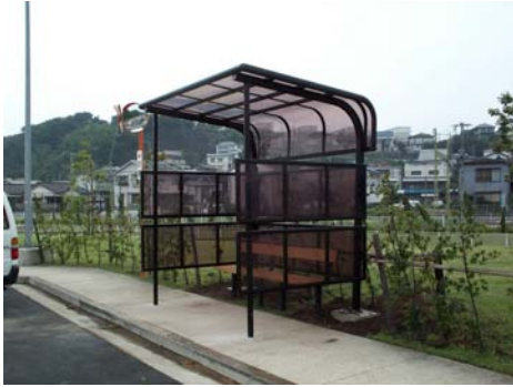
Above: Ikego Bus Stop, keeps school children and residents out of the weather
