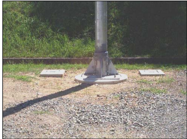
Left, installation of steel lightning mast. Close up of completed mast.
