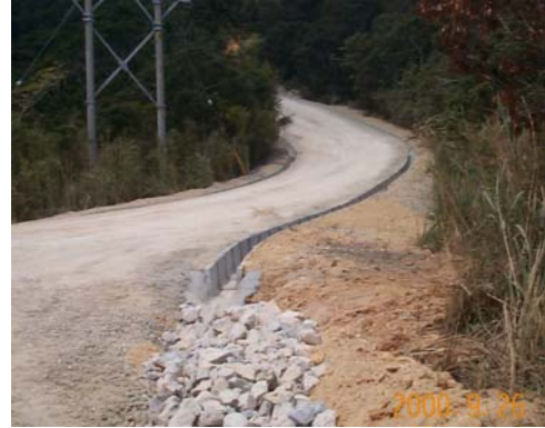
Above, Completed soil stabilization and installed U-ditching with gabion rock to divert runoff and prevent washout of roadway.
