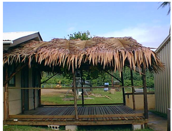
Above: Tropical patio constructed at Camp Combs.
