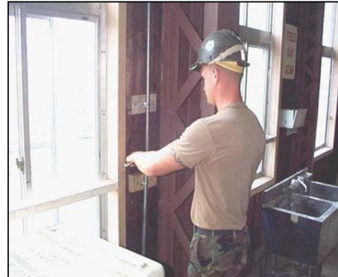
Putting the finishing touches on conduit for extension of LAN system
