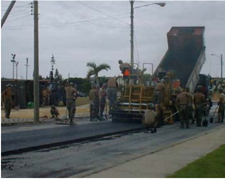
Right, spreading new asphalt onto existing road with asphalt paver.
