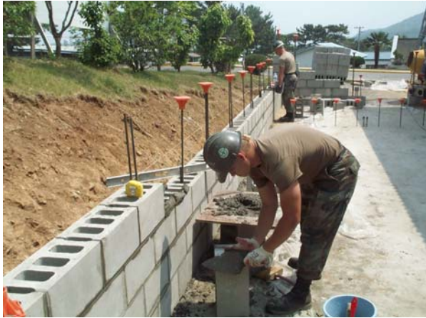
EO3(SCW) Matthew Johnson and BU3(SCW) Justin Smoyer, Laying CMU exterior walls.
