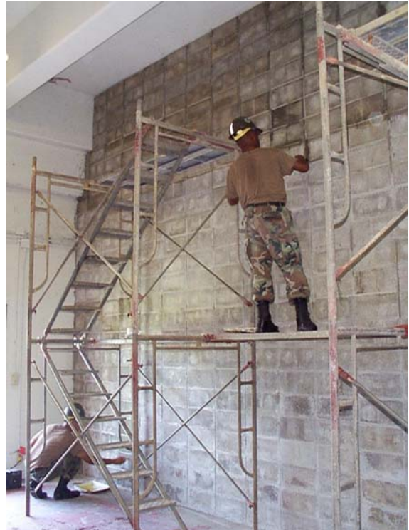
Install Concrete Masonry Wall at Building 7205 galley.
