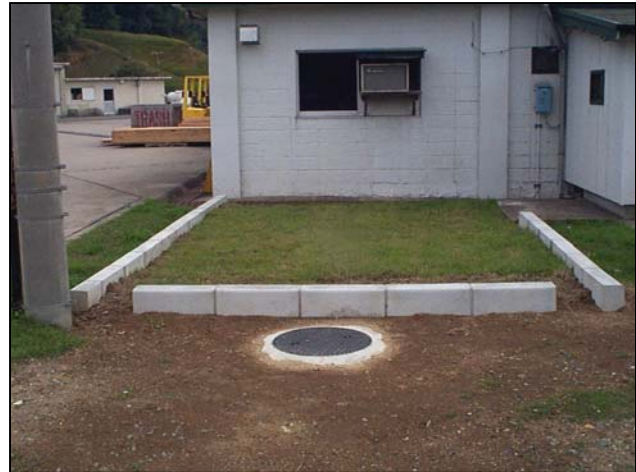
Left, perforated PVC piping for leach field. Below, completed leach field.
