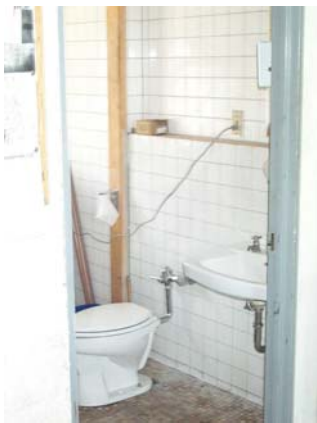
Above: Repaired and relocated commode, tiled the walls, and installed a washer in the CM shop.
