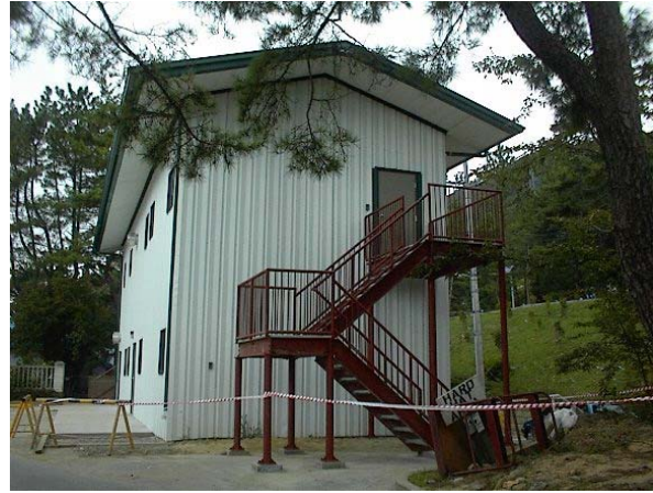
Northeast project view.
