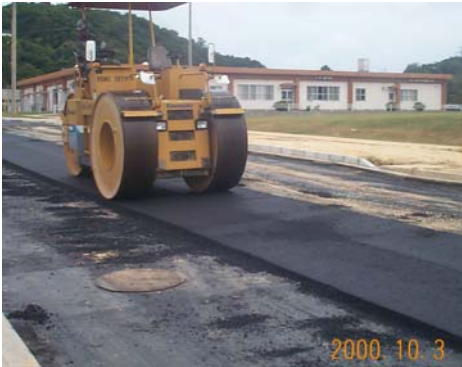
Above, rolling new asphalt onto existing road.
