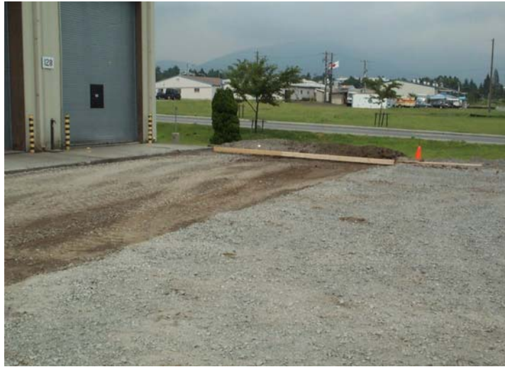
At top left, the existing site. Bottom left, formed up for the 3 rd pad. Below, formed up for the 4 th pad.
