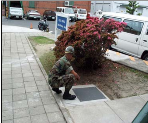
Inspecting pad prior to installation of mailbox.
