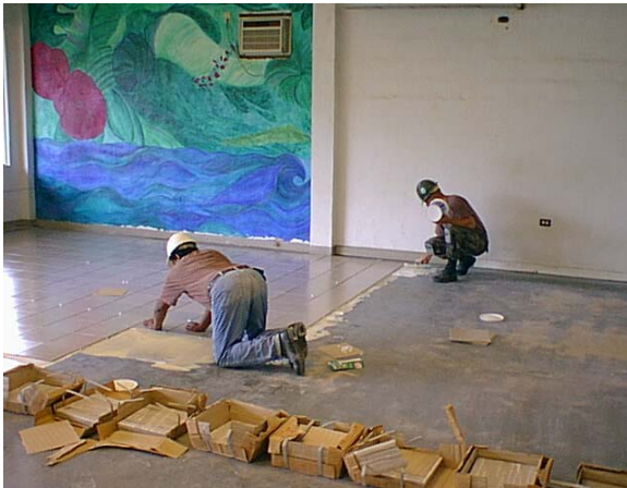
Above: Seabees and apprentices laying ceramic tile at Pohnpei State library.
