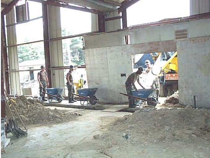
Detail Pohang Seabees place concrete in Messhall interior.
