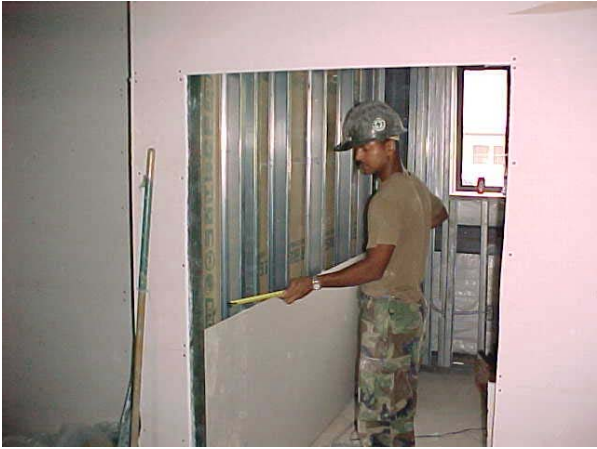
Measuring for drywall.
