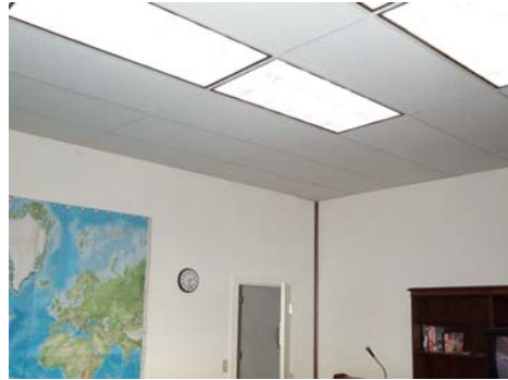
Above: COMDESRON 15 lounge Upgrade, provides a private conference area and a separate kitchen area to minimize noise and personnel traffic
