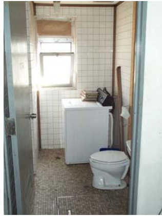
Above: Repaired and relocated commode, tiled the walls, and installed a washer in the CM shop.
