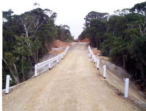
Above and right, completed soil stabilization and shotcrete of washout area, guardrails in place.
