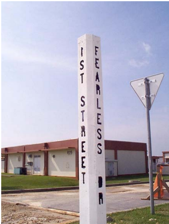
Construct Road Signs for Fearless Drive.
