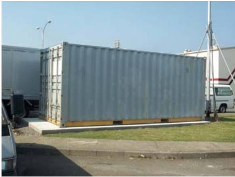
Above: Post Office Concrete Pad, prevents water damage to the storage container needed for additional capacity for the Post Office
