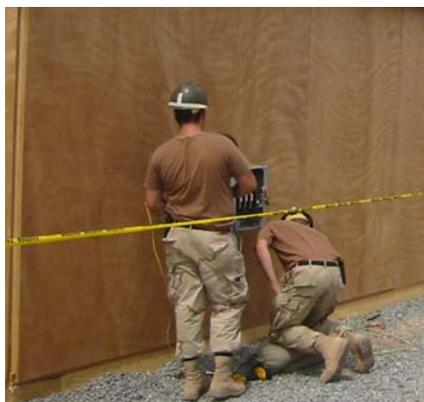
*Figure 2: NMCB 74 Seabees installing Electrical Panel For New Gym*
