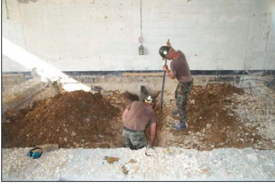
LEFT: Bravo Co. crewmembers excavating for grade beam and footer forms. BOTTOM: Bravo Co. Crewmembers compacting after grade beam, footer and under slab utility placement.
