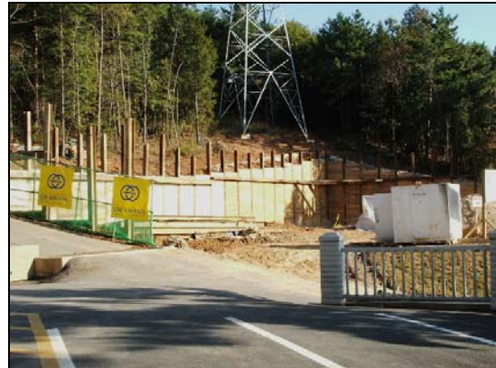
LEFT: Site prior to construction, SEP 05. BOTTOM: Site at turnover, DEC 05
