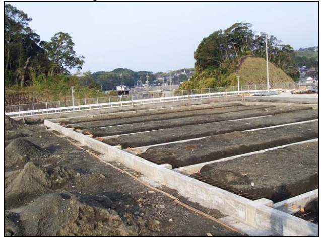
BOTTOM: Completed concrete foundation.
