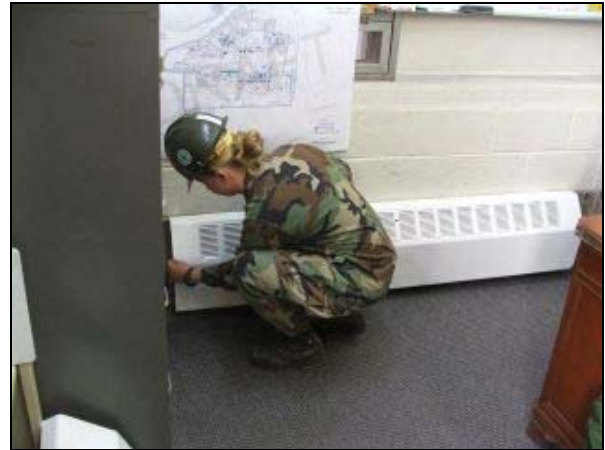
A Seabee places a rehabilitated radiator cover in the OIC's office.
