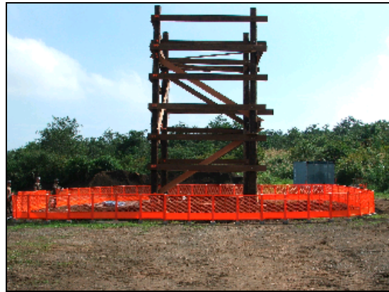
LEFT: Crew setting top poles in place as tower is being constructed on its side. BOTTOM: Tower erected in place.
