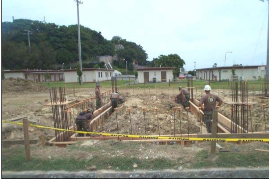
LEFT: Crew is forming and placing RST for building grade beams. BOTTOM: Windows and doors installed, roof poured and waiting for exterior painting.
