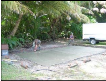
Finishing concrete pad for pavilion.
