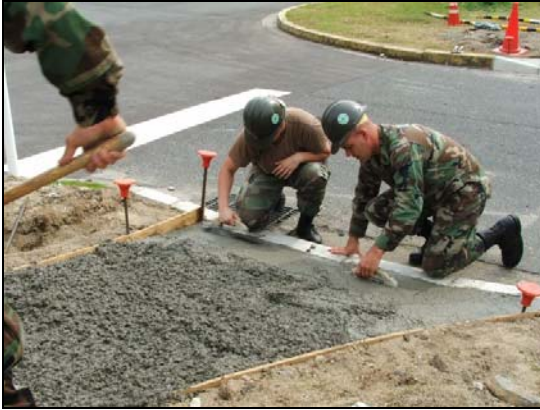
LEFT: Seabees finish concrete handicap ramps with magnesium floats. BOTTOM: Evidence of the completed project.
