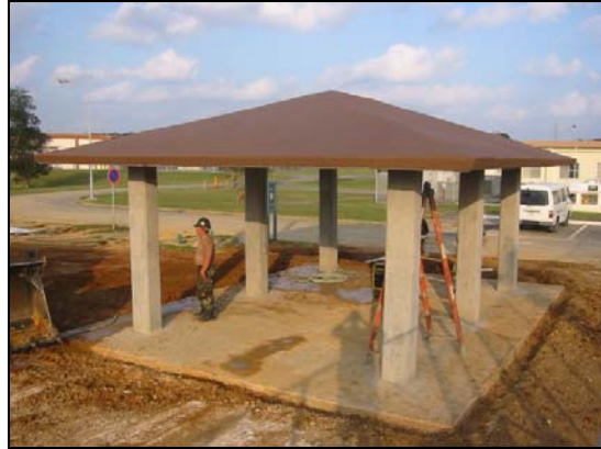
BOTTOM: Pavilion A – Completed. Contractor completed exterior paint.
