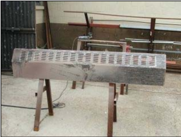
The camp facility's radiator covers were stripped and repainted.
