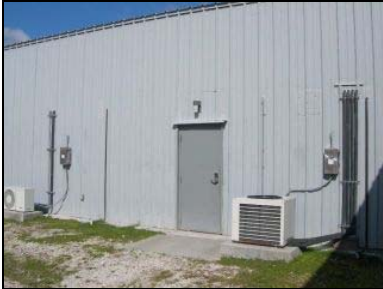
Rear entrance prior to canopy placement
