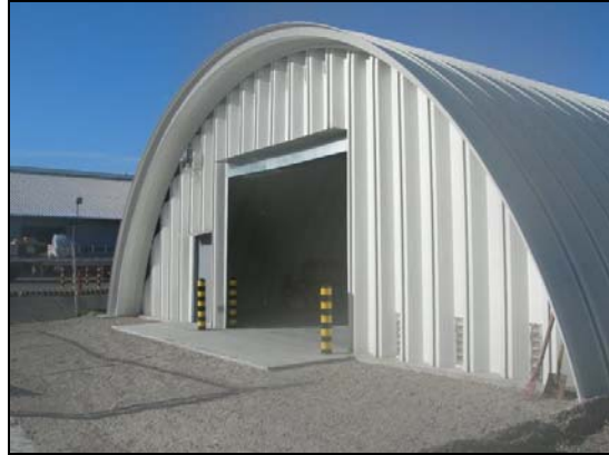
BOTTOM: View from front overhead door of completed K-Span #2
