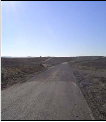
Section One of Ridge Road Repair. (after)
