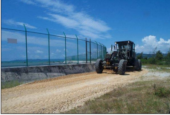
LEFT: Initial grading of the road. BOTTOM: Completed road.
