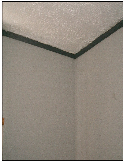
Finished trim work for BEQ room.
