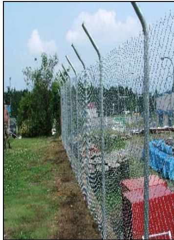
Installation of chain link fencing.
