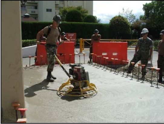
LEFT: The entire crew received whirly-bird operator training as they finished the concrete floor slab. BOTTOM: The completed project.
