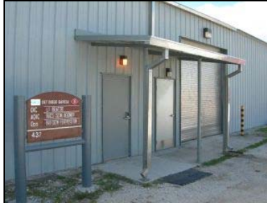
Front entrance with new canopy and guttering
