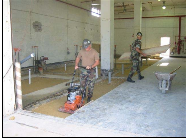
LEFT: Bravo Co. crewmembers excavating for grade beam and footer forms. BOTTOM: Bravo Co. Crewmembers compacting after grade beam, footer and under slab utility placement.
