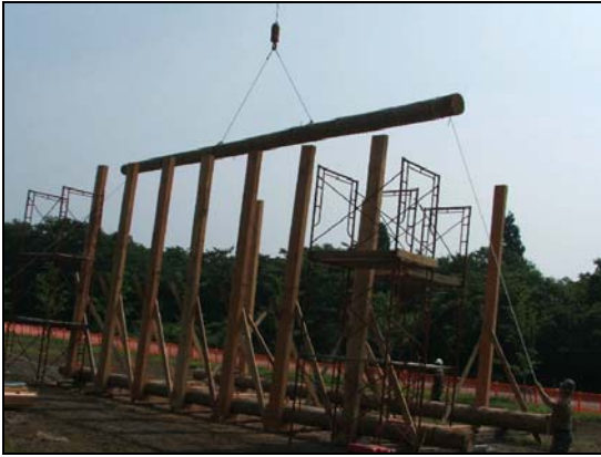
LEFT: Crew setting top poles in place as tower is being constructed on its side. BOTTOM: Tower erected in place.
