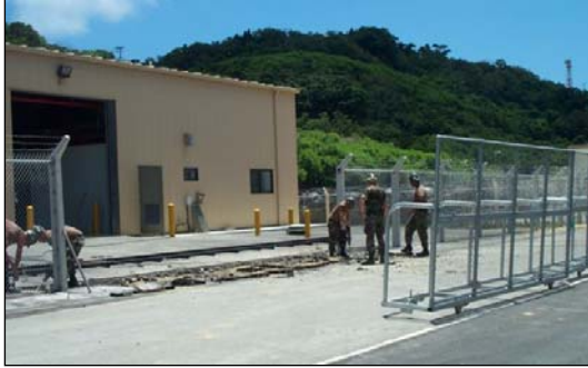
LEFT: Crew prepares the asphalt to install the fence rails. BOTTOM: Completed project.
