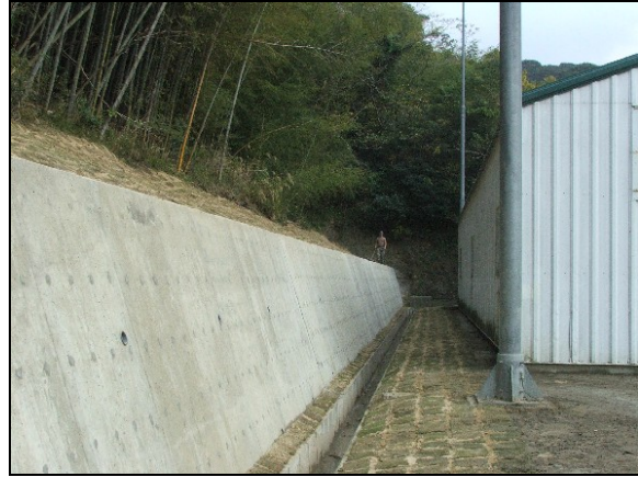
BOTTOM: Finished retaining wall.
