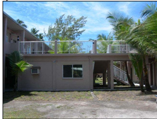
LEFT: Crew placing concrete for stairwell leading to sundeck. BOTTOM: Side view of completed CPO Lounge project.
