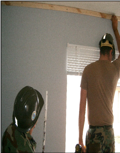
Placing trim work for BEQ room.
