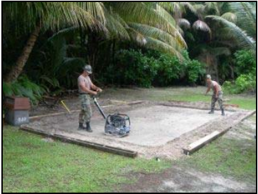
Compaction of sub-base for pavilion pad.
