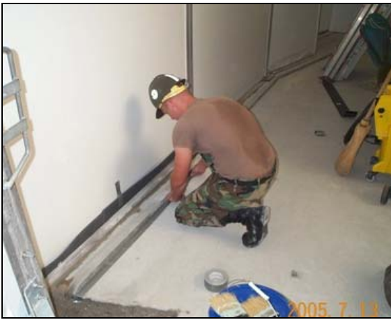
Crew Member prepares concrete channel for sealant. Completed exterior TFS sealant repairs.
