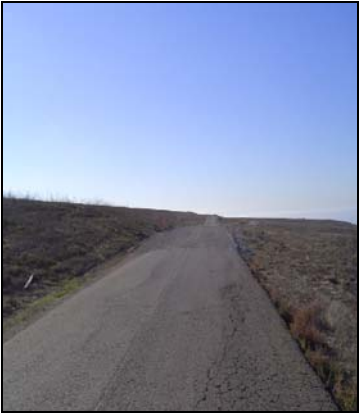
Section Two of Ridge Road Repair. (after)
