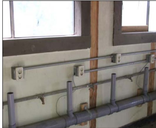
BOTTOM: New utility work in the laundry facility.
