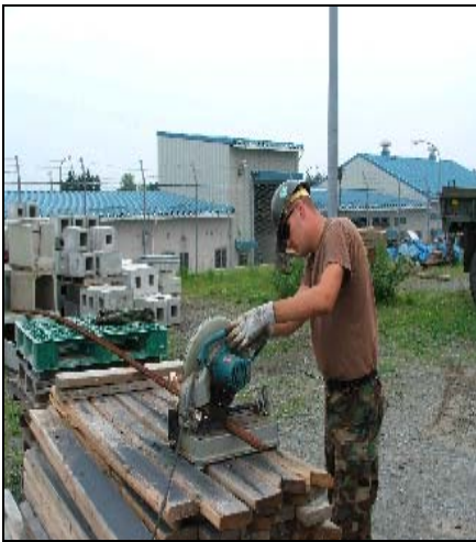
Crewmember cutting rebar for the loading ramp.
