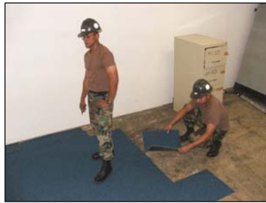
Installing carpet for Conference Room
