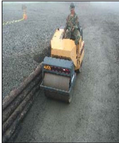
Crewmember rolling the loading ramp.
