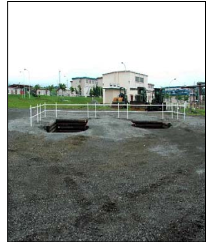
Completed loading ramps.
