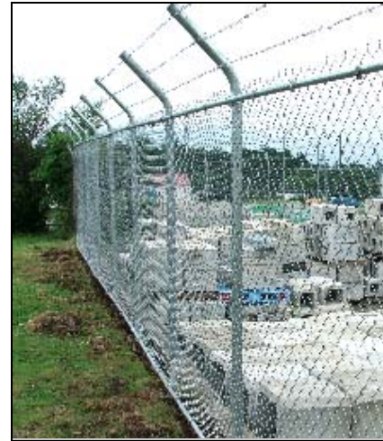
Completed fence with barbed wire.
