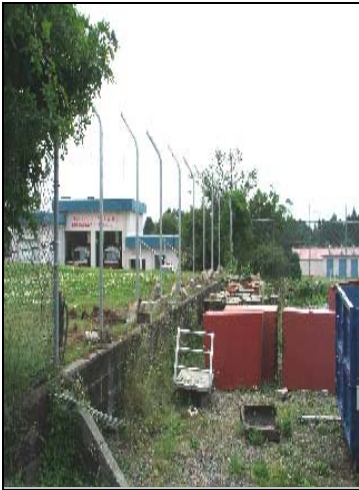
Installation of the fence posts
