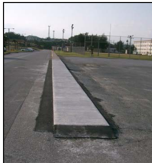
Completed grinder sidewalk
