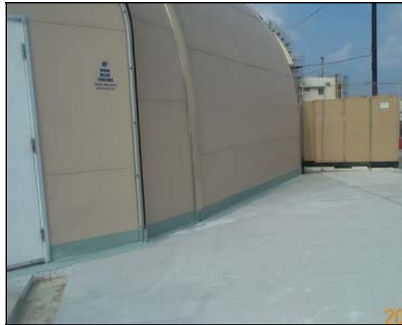
Crew Member prepares concrete channel for sealant. Completed exterior TFS sealant repairs.
