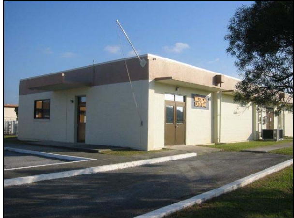
LEFT: Completed Dental room. BOTTOM: Project is complete less contracted work for the fire alarm system.
