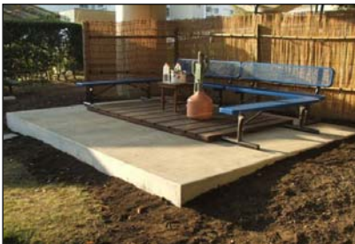
Ikego Patio project after.
