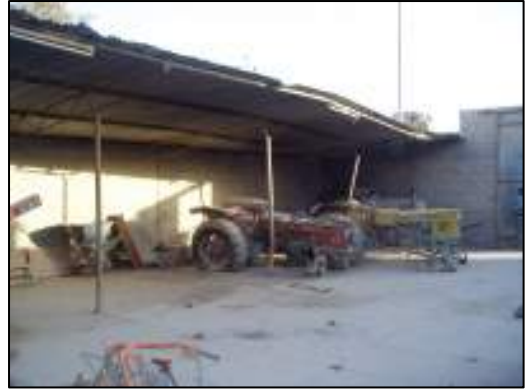
Condition of an existing structure.
