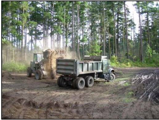
Fig. 53 – Detail Whidbey Island clears an area for future projects.
