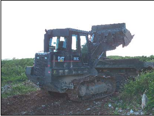
Cleaning up the quarry roads.
