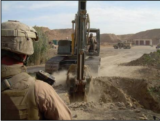
Excavation for culvert.
