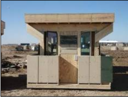
Completed "Crow's Nest" in pre-fab yard.
