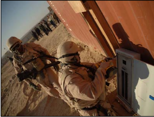
CEs install electric service to a berthing container.
