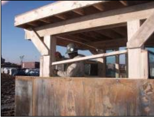
Framing for the ballistic glass.
