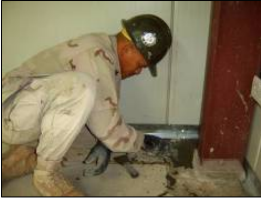
Seabee places non-shrink grout beneath column.
