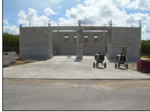
Orote Point Mechanic Shop.
