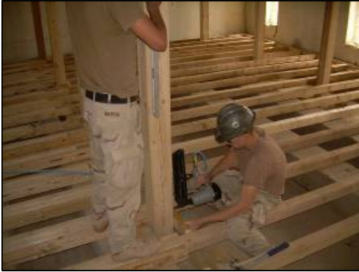
Installation of one of the posts for the overhead protection.
