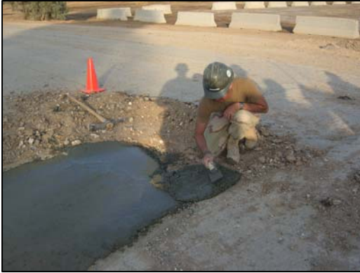
Seabee makes repairs to damaged roadways on camp.
