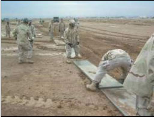
Seabees install AM2 matting for runway.
