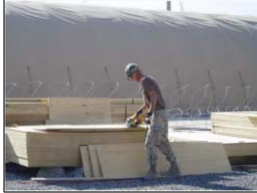
Seabee cuts wood for tent base.
