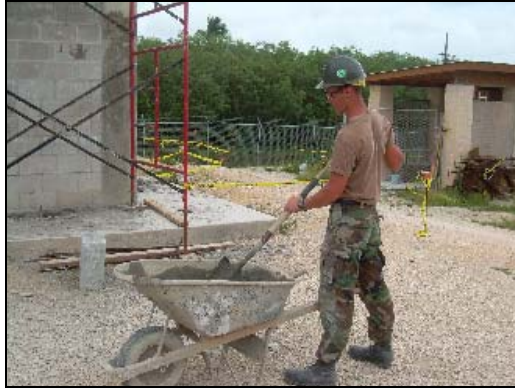
Mixing Mortar for CMU block.
