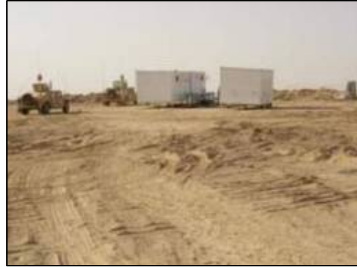
Completed installation of berthing units.
