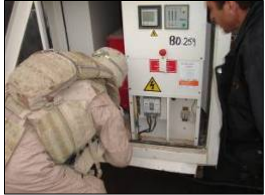
Final connections to the new generator.
