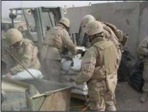
Mixing Quickrete using the 11s mixer.
