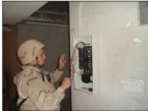
Installation of the facility's breaker panel.
