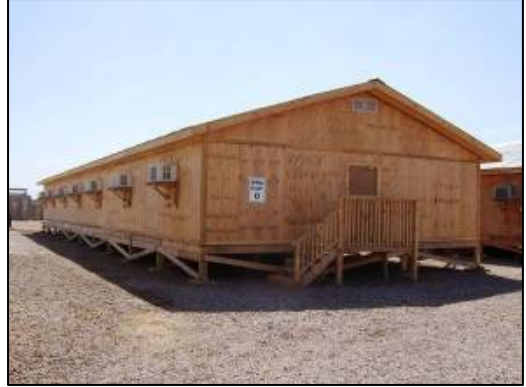
Completed SWA hut.
