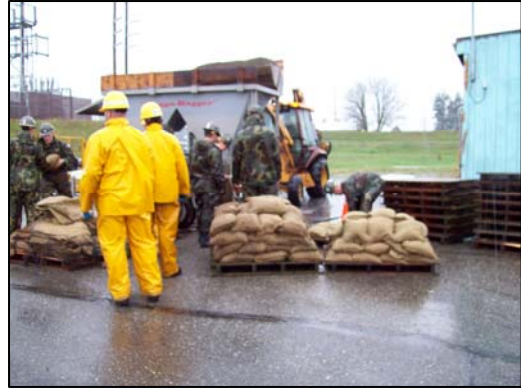
Skagit Valley Sand Levee re-enforcement.
