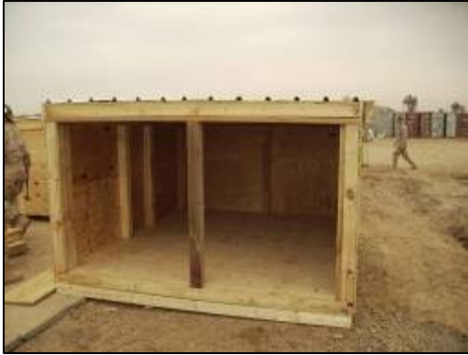
Pre-fabricated pre-detonation roof section at Delta Co. fabrication yard.
