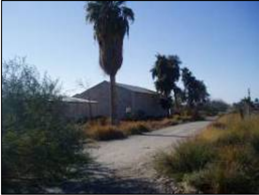
Building and roadway at the proposed site.
