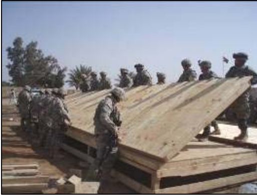
Installation of the pre-fabricated wall section.
