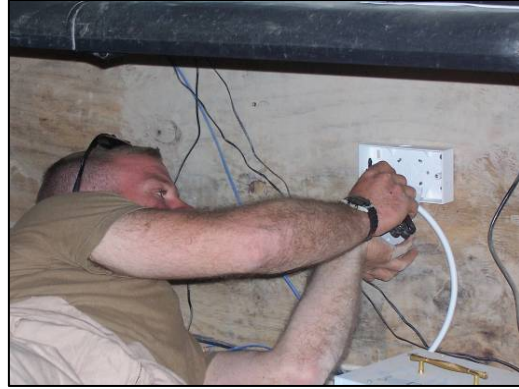
Upgraded Electrical at OP Dunlap.
