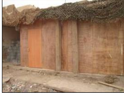
Completed wall section.
