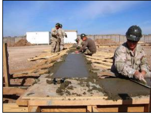
Crew finishes concrete grade beams.
