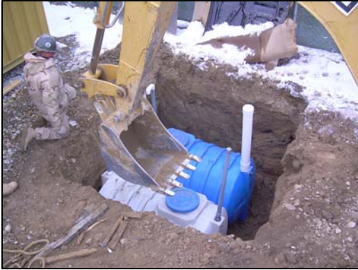
Seabees excavate for a septic tank.
