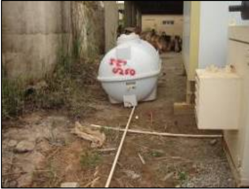
Water storage tank and shower trailer at the Gov't Center.
