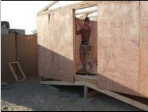
Constructing the deck of a SWA hut.
