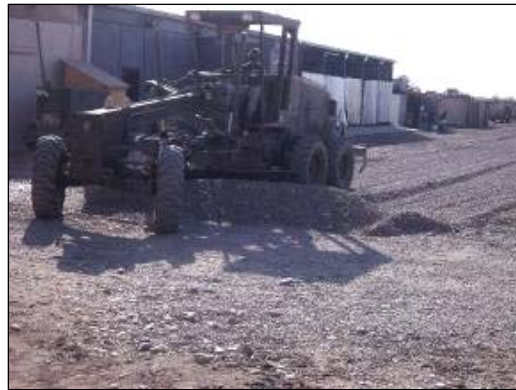
Road repairs at DET-ONE.
