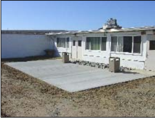
Completed concrete patio at the Islander Club.
