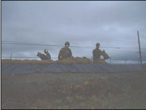
Seabees position sandbags to reinforce levee.
