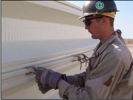
Seabee sets clamps on metal for K-Span.
