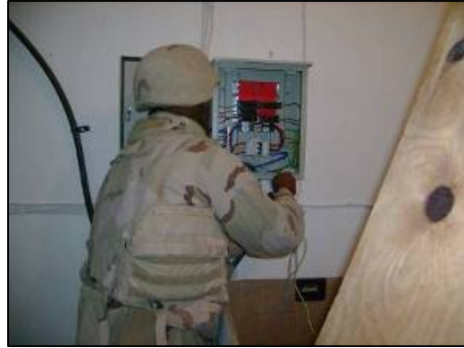
Installation of the facility’s breaker panel.
