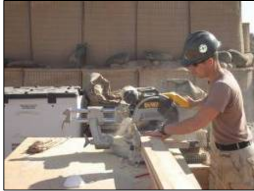
Construction of one of the walkways in the Delta Company yard.
