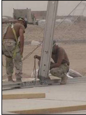
Crew preparing to stretch fabric through rails.
