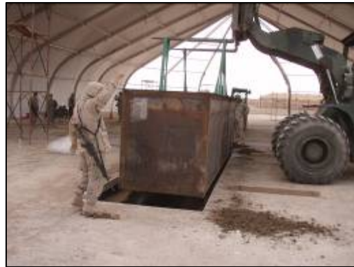
Completed maintenance pit with concrete bond beam placed.
