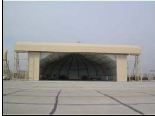
Completed Sprung Structure.
