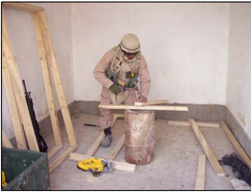
Seabees frames a wall at PB Firecracker.
