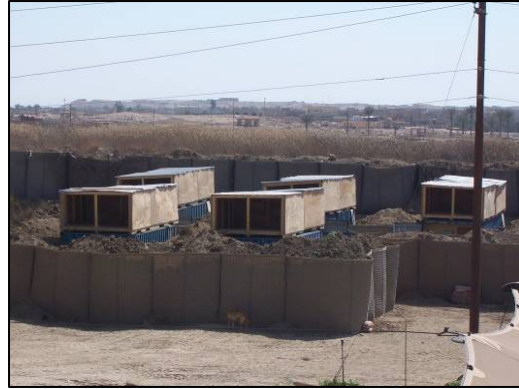
ISO Berthing containers set in place.
