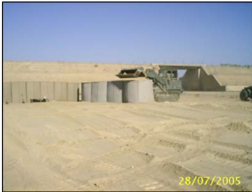
Construction of the HESCO structure.
