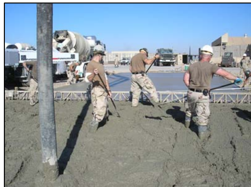
Fig. 37 – Seabees place concrete on airfield at TFS Main Body.
