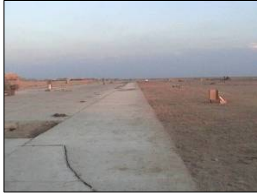
Grading the earth subbase in preparation for forming and concrete placement.
