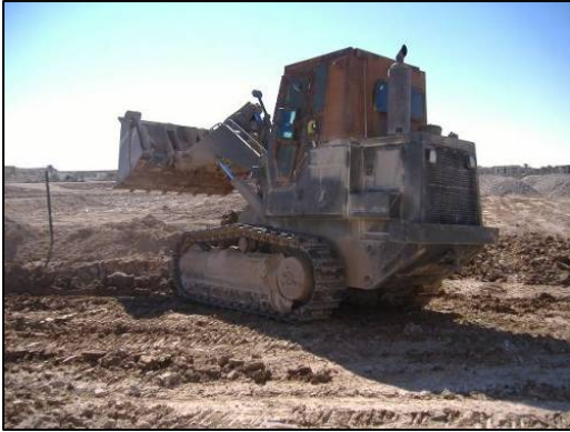
Removing ruts from OP Cubs parking area.
