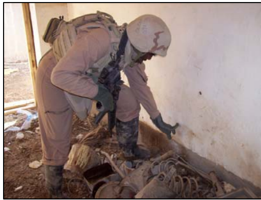
Fig. 25 – Seabee investigates work site at a Combat Outpost in Ar Ramadi.
