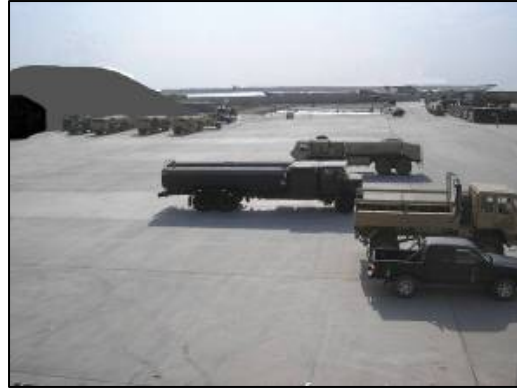
Overhead view of airfield concrete pads.
