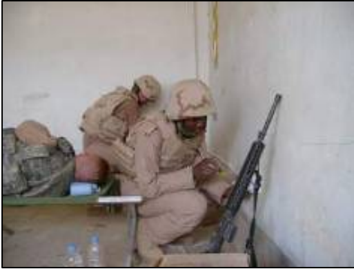
Installation of the electrical wiring.
