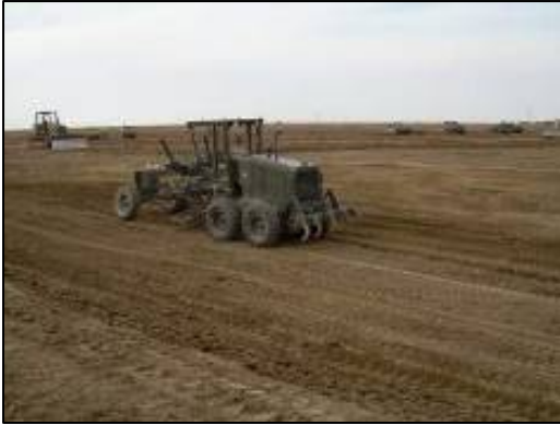
Grading operations on Phase II.
