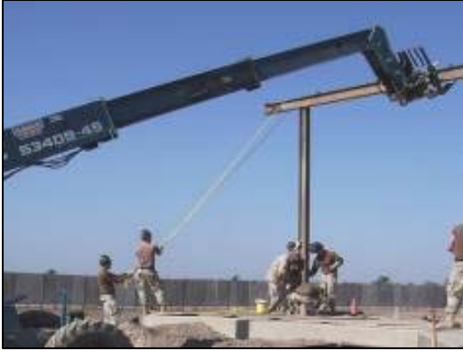
Steel members being lifted into place.
