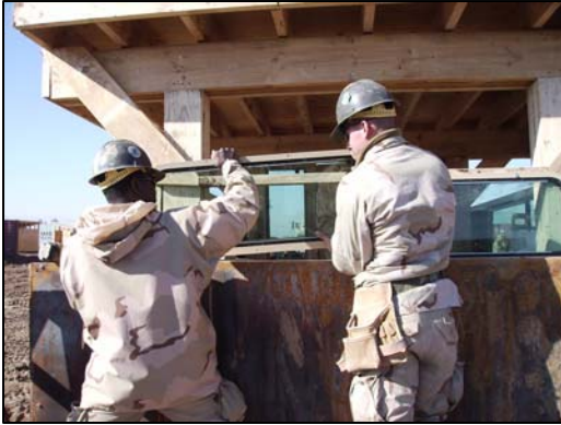
Seabees install ballistic glass for “Crow’s Nest”.
