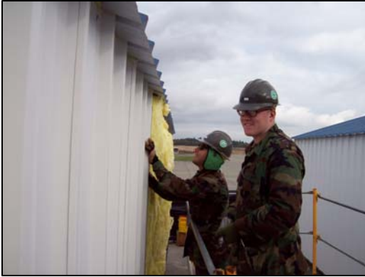
Seabees attach siding to exterior of PEB.
