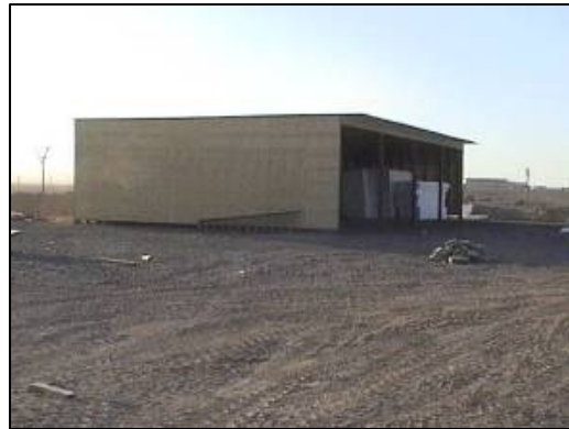
Class IV Yard Pole Barn completed.
