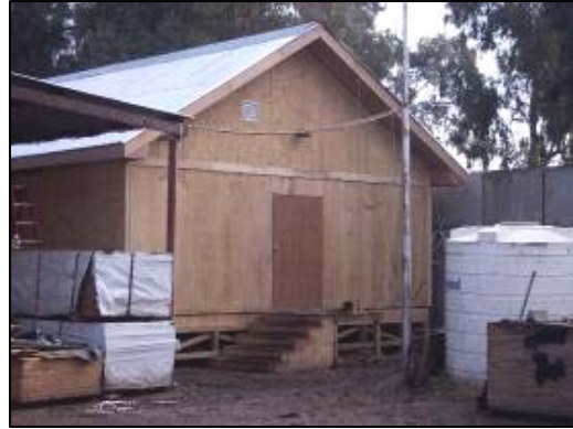
Completed SWA hut.
