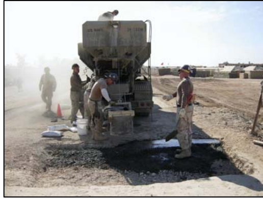
Seabees make repairs to roadway damaged on camp.
