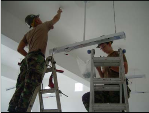
Seabees hanging lighting inside facility.
