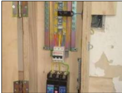
Installation of a circuit to one of the guard posts.
