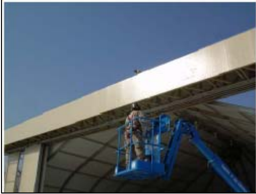
Seabee finishes door installation.
