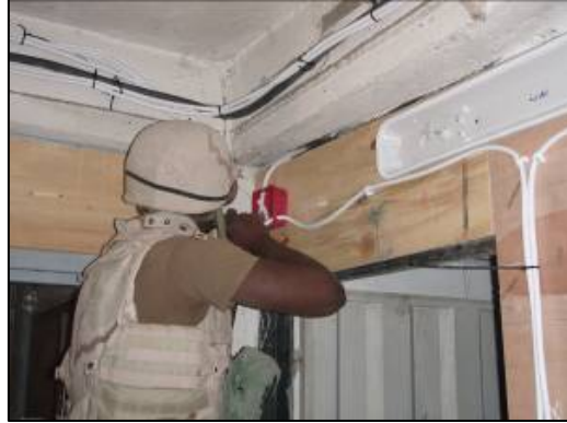
Installation of a lighting circuit on site.
