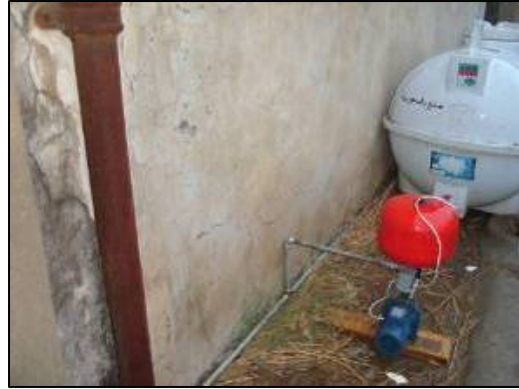
Completed installation of water pump.
