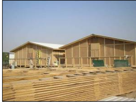
SWA Huts under construction.
