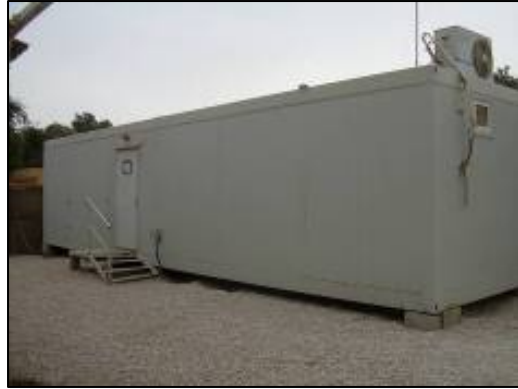
Shower trailer in place and operational.
