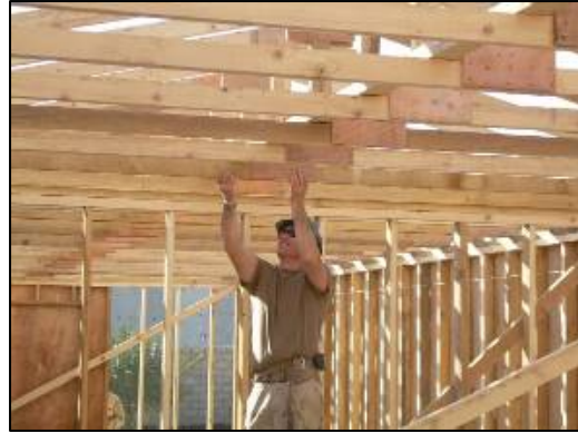
SWA hut construction in progress.
