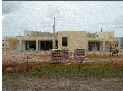
Laundry Facility with paint in progress.
