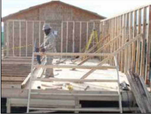
Seabee frames walls for laundry facility.
