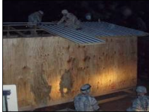
Completing the roof panel installation.
