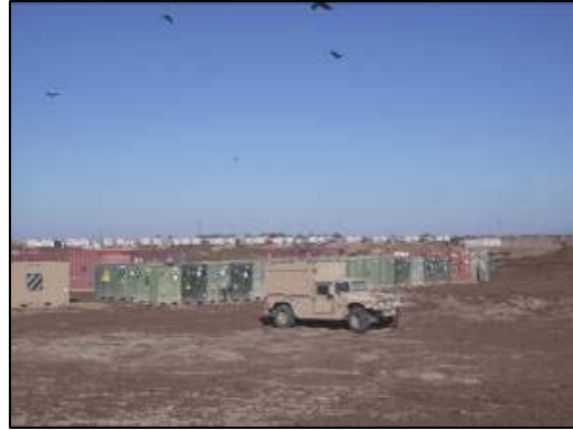
Completed laydown area.
