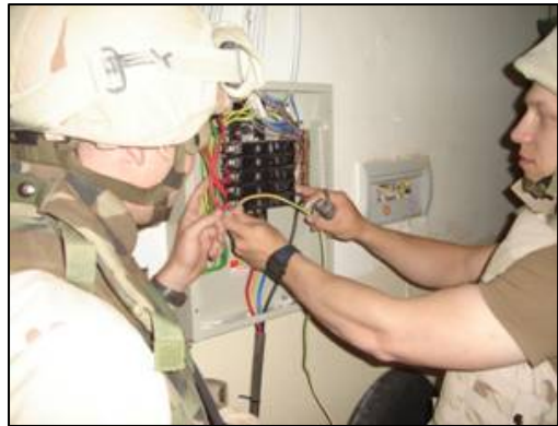
Seabee provides electrical support to COP North.
