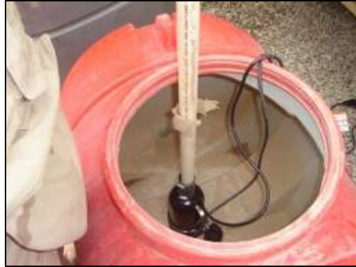
Installation of a sump pump for a gray water tank.
