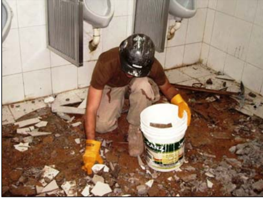
Seabee removing floor tile.
