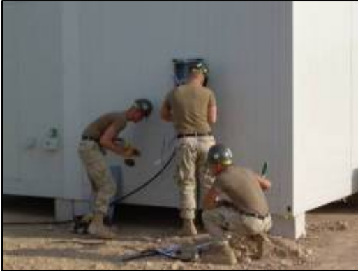
Electrical wiring for new POD trailer.
