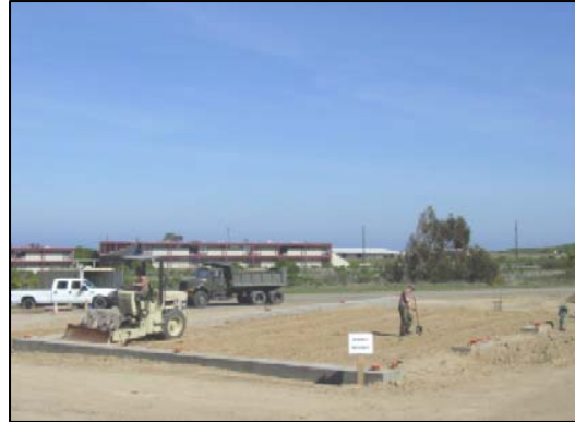
Backfill placed.
