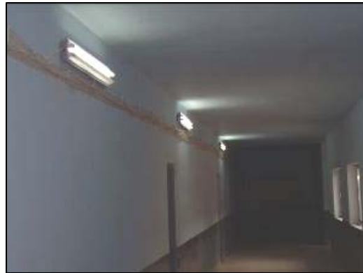
Completed rewiring of lighting in hallway.
