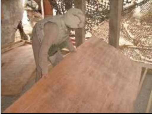
Securing plywood to a wall frame.
