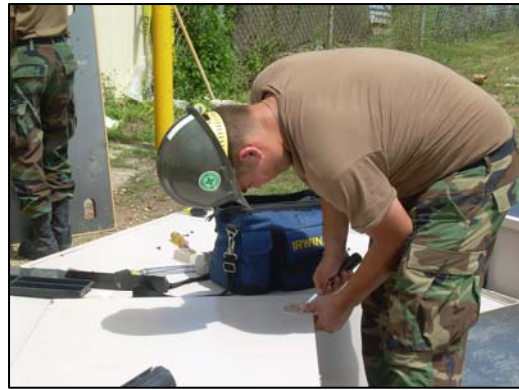
Fig. 35 - Seabee constructs a door.
