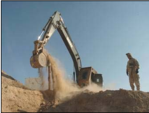
Fig. 51– Excavating at OP Viking.
