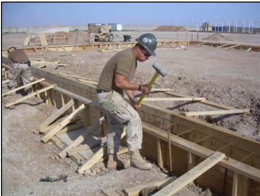
Fig. 36 – Seabee setting forms for concrete placement at DET-ONE.
