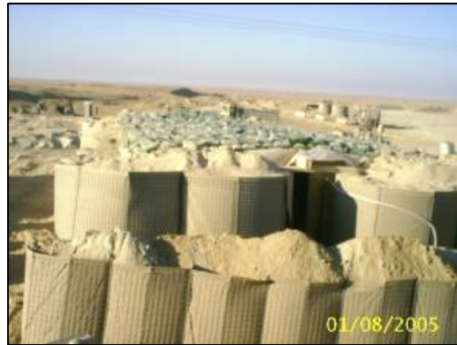
Completed Outpost structure.
