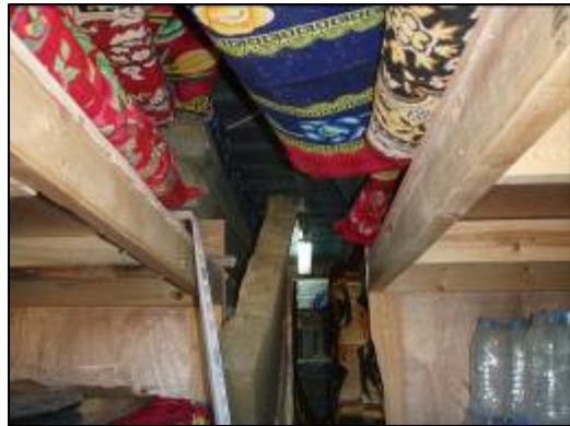
Lighting installed inside an ISO berthing unit.
