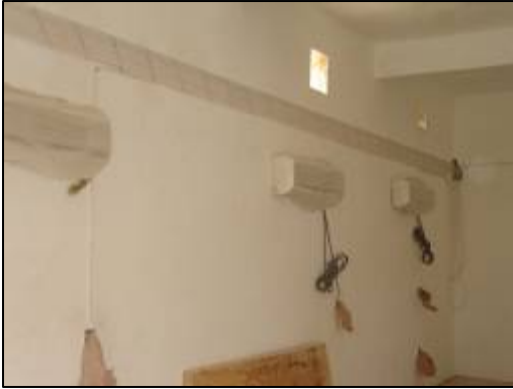
Installation of A/C units by the contractor.
