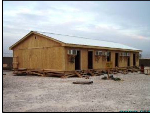
Completed SWA hut.
