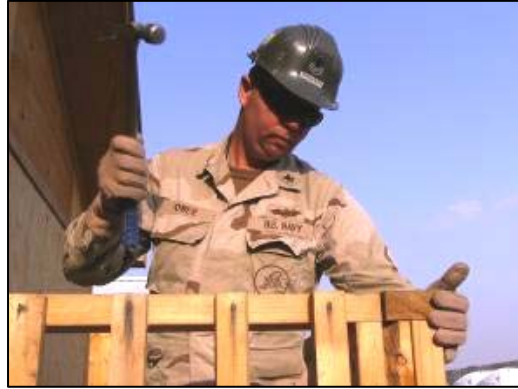
Seabee fixes a guardrail.
