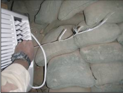
Operational check of an installed A/C unit.
