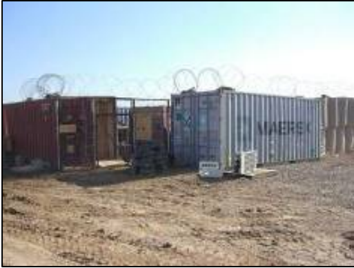
Construction of the temporary armory.
