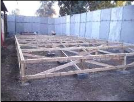
Floor joists are set on SWA hut.
