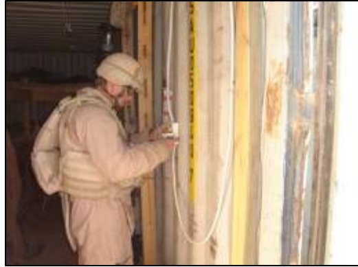
Making the final electrical connections inside a berthing area.
