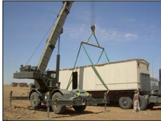
Fig. 27 – Crane is used to off-load a trailer.
