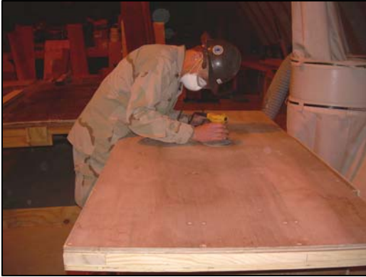
Seabee prepares to router a door.
