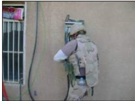
Installation of an electrical panel.
