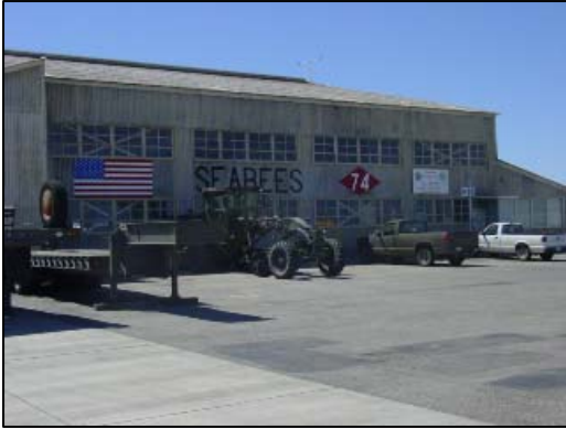
Exterior of Detail Office Space.
