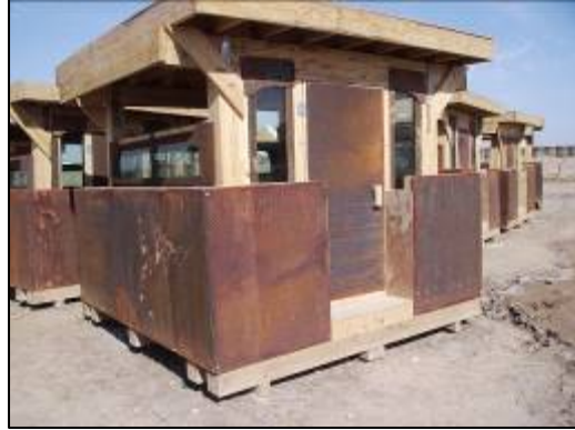
Completed “Crow’s Nests” ready for installation.
