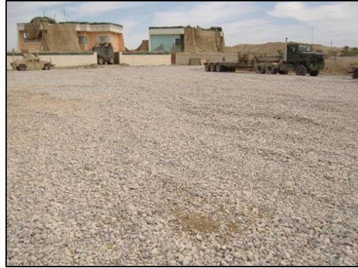
Completed gravel work at OP 573
