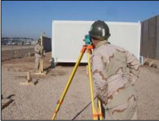
EAs set piers to grade.
