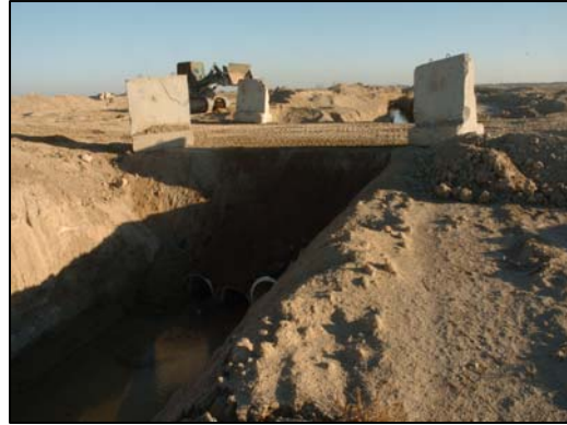
Completed culvert crossing.
