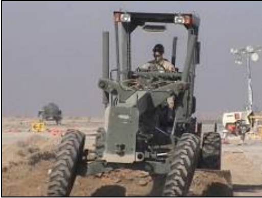
Completed V22 expansion of SW side of Kilo taxiway.
