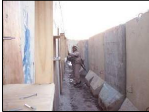
A/C installation on the COP.
