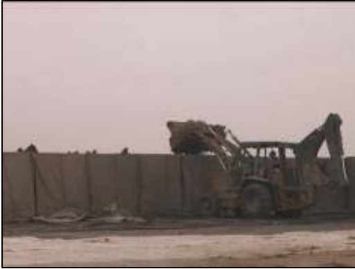
Filling of HESCO barriers.
