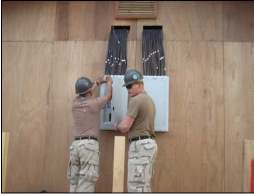
Seabees wire up circuit panel for SWA hut.
