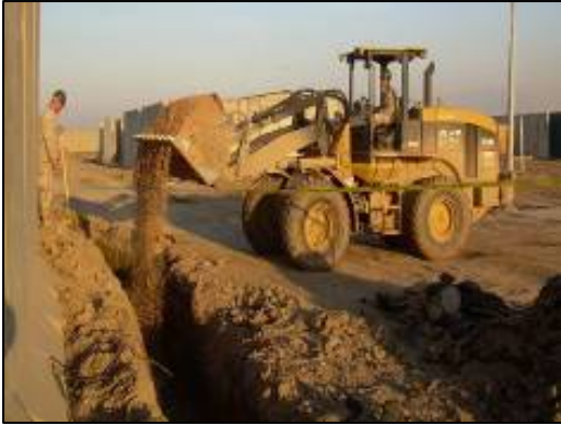
Fiber optic trenching operations.
