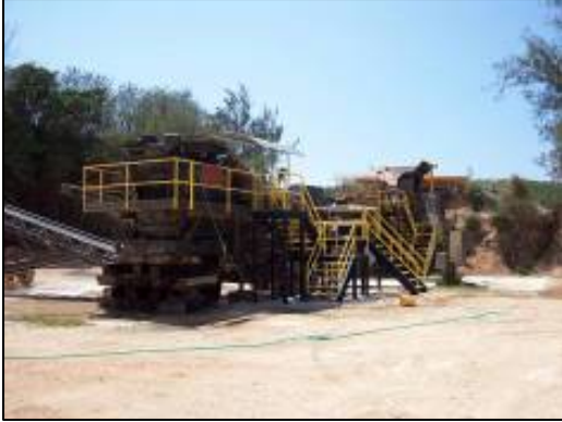
The crusher with new stairs.
