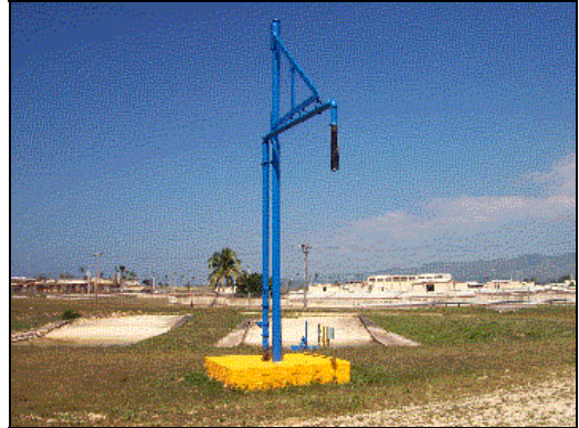
A new coat of paint on water distribution point.
