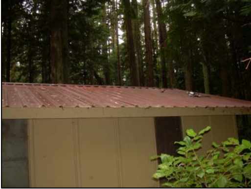
Re-roofed Cabin on Whidbey Island.
