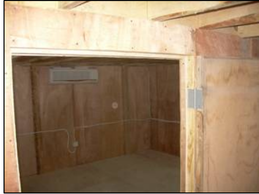
Completed berthing area with overhead protection in place.
