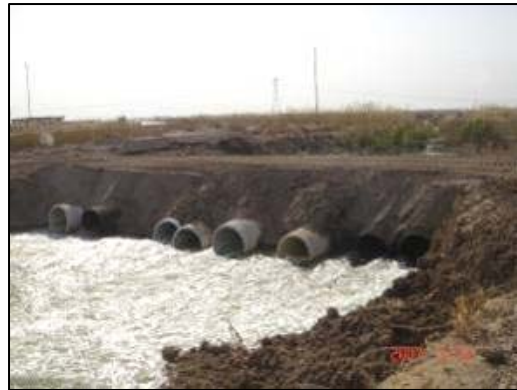
Completed roadway with eight culverts in place.
