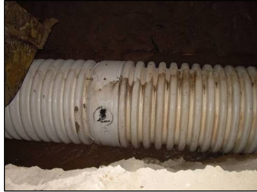
Culvert placed in trench.
