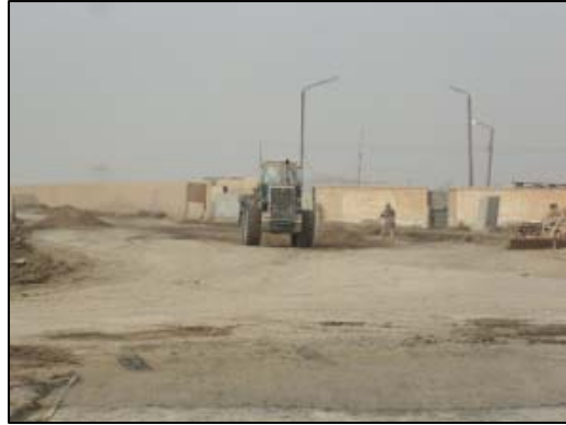
Completed roadway looking SE.
