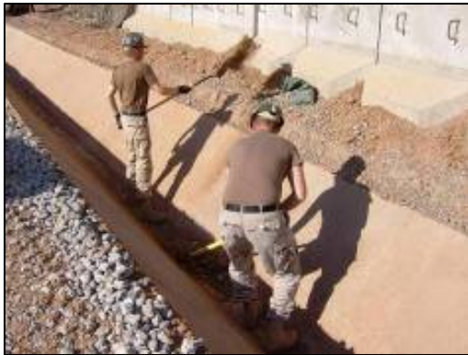
Seabees keep drainage ditch clear of debris.
