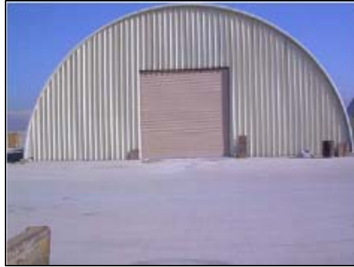
Completed K-Span structure.
