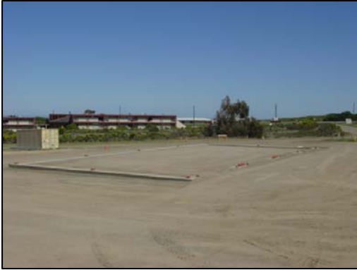
Grade beams and Backfill completed.
