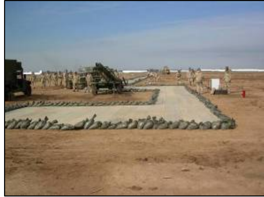
Install temporary UAV runway.
