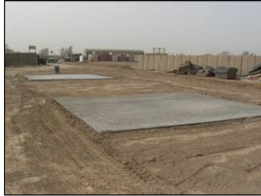
Install temporary UAV runway.
