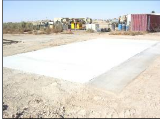
Completed pad with ramps constructed.
