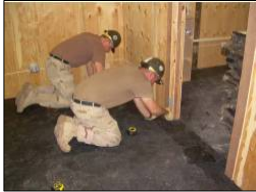
Seabees lay floor matting.
