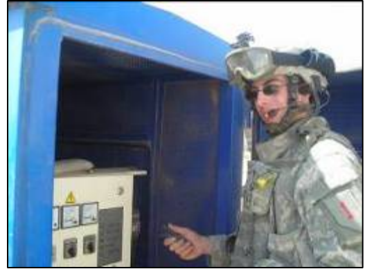
Completed generator installation.
