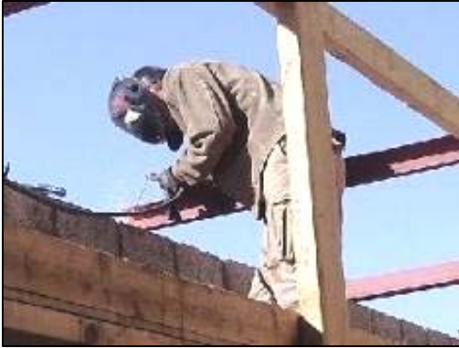
Seabee welds steel roof.
