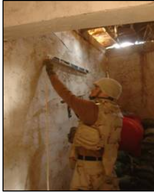
Seabee installs lighting at COP.
