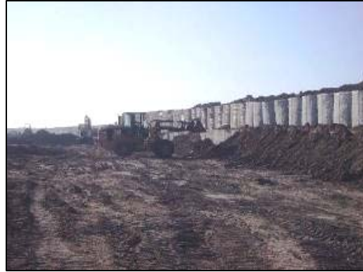
An earthen berm is pushed up around Hesco barriers.
