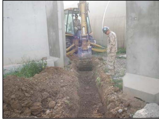
Trenching for new fiber optic installation.
