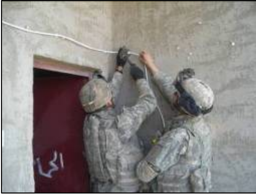
Installation of wiring by Army engineers.
