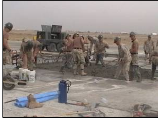
Concrete placement on runway.
