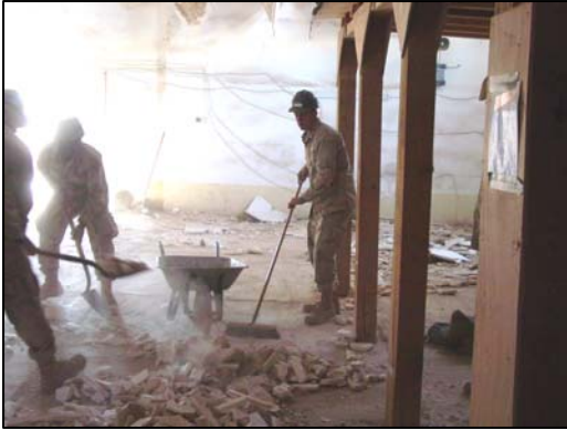
Seabees demolish existing facility.
