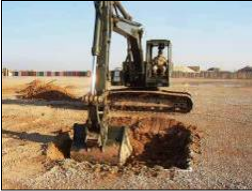
Breaking ground on footers.
