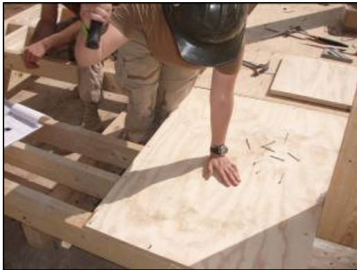
Prefabrication of decking for a “Crow’s Nests” in Ar Ramadi.
