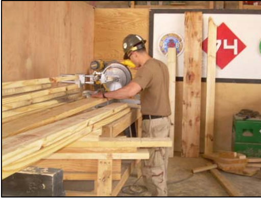
Lumber being cut to fulfill a project BOM.
