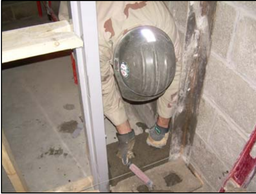
Seabee lays CMU block.
