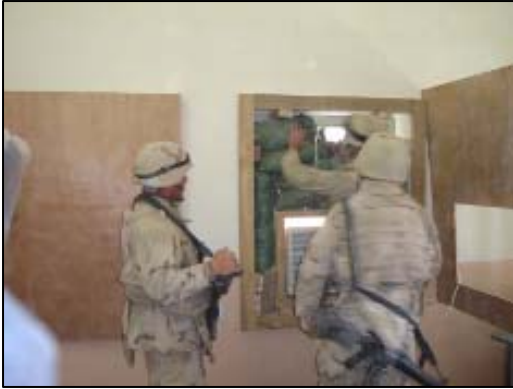
Installation of a window A/C unit and sandbags.
