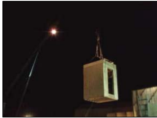
Night crane operations.
