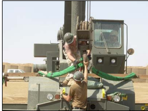
Fig. 52 – Rigging for a crane lift.
