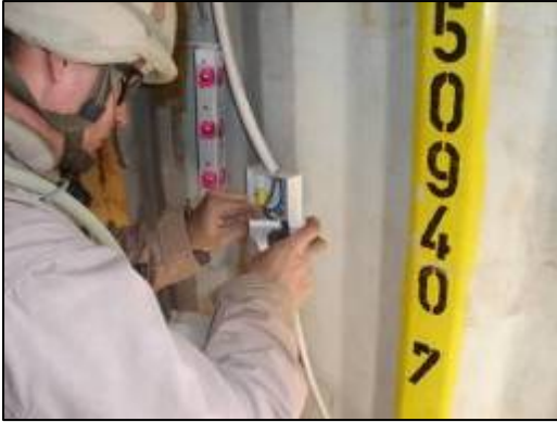
Electrical installation of a switch.
