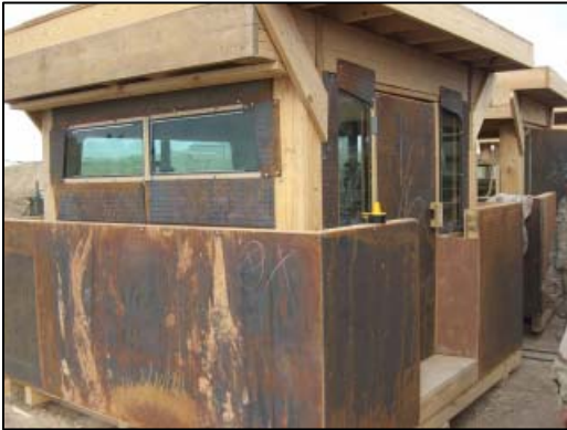
Fig. 26 – “Crow’s Nest” under construction.
