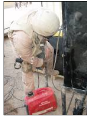
Installing the grounding rod for the generator.
