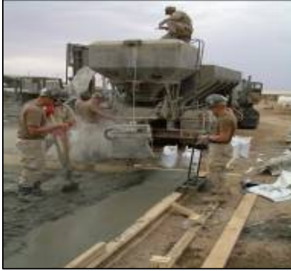
Concrete placement using the Cretemobile.
