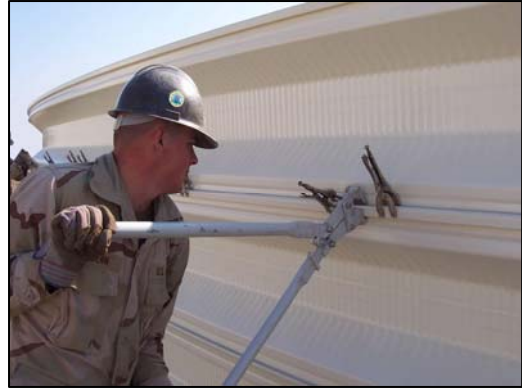
Seabee bends K-Span reinforcement into place.
