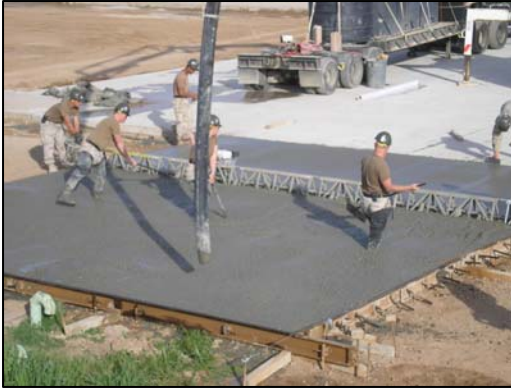
Seabees place a section of concrete pad.
