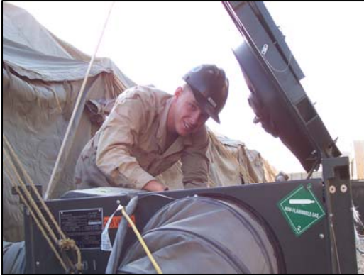
Seabee provides repairs to HVAC.
