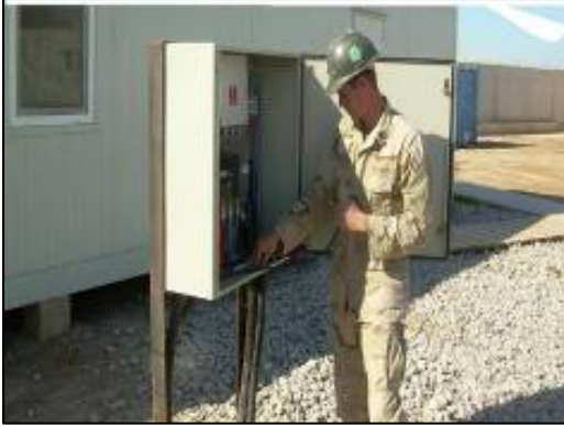
Low voltage breaker and cable repair.
