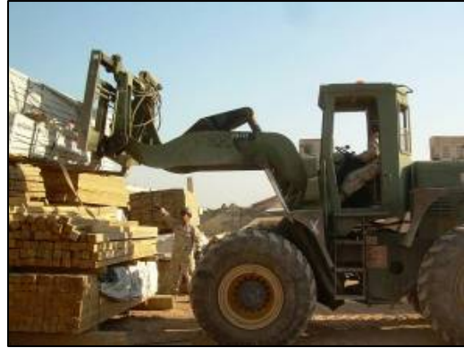
Material movement for staging to FOB locations.
