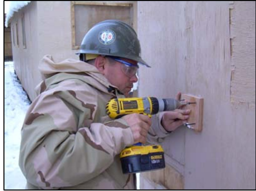
Seabee makes repairs to facilities.
