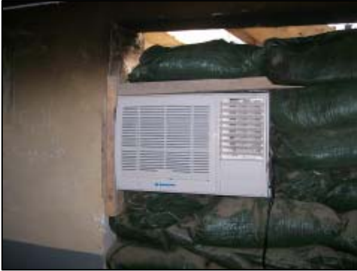
Completed A/C unit installed with force protection.
