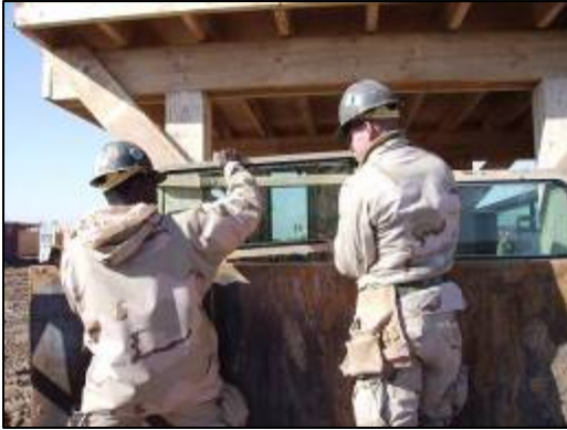
Installing ballistic glass on a “Crow’s Nest.”
