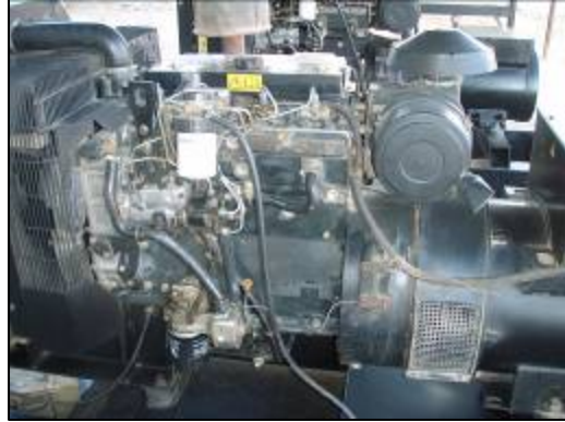
Completed repairs to generator.
