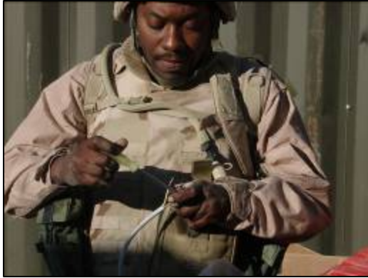
Splicing wires to complete electrical connections.
