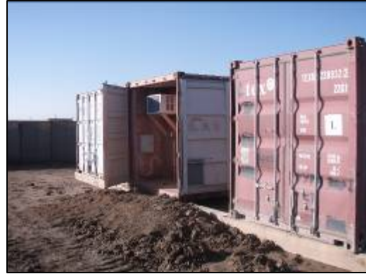
Installed ISO berthing units before the pre-detonation roofs are installed.
