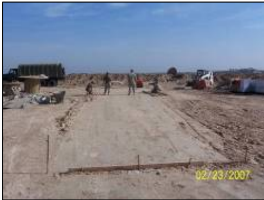
Crew placing forms for IED Trainer Road.
