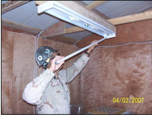
Seabee changing light bulb in Camp Maintenance Shop.
