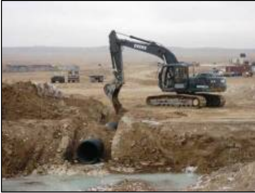
Excavating retention pond for Water Well operations.
