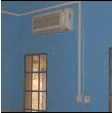
Completed installation of A/C unit in barracks.
