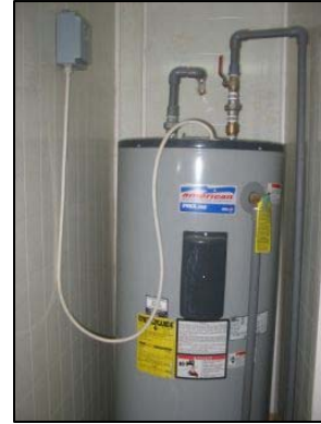
Newly installed water heater.
