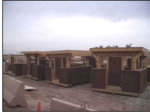
Completed "Crow's Nests" awaiting installation at COPs.
