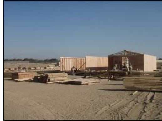
Class IV staged for SWA hut construction.
