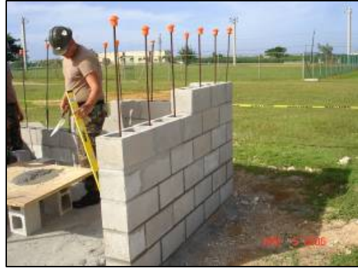
Seabees laying block.
