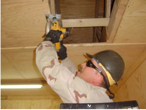
Builders cutting access hole into ceiling.
