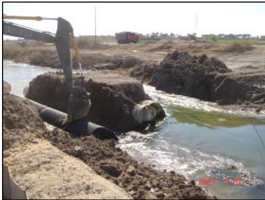
Placement of one pipe after breaching the previous crossing.
