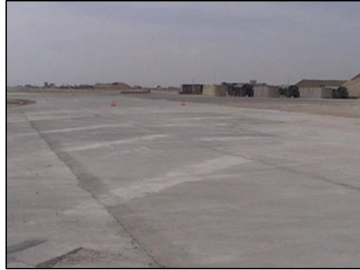
Taxiway Kilo and Delta intersection.
