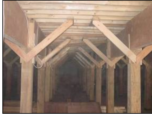
Completed framing of the pre-detonation layer.
