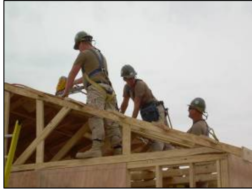
Sheathing roof of new SWA hut.
