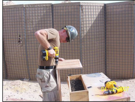
Seabee constructing boxes for TOA weapons shipment.
