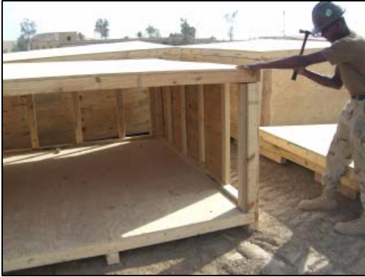
Construction of a pre-detonation roof for an ISO berthing container.
