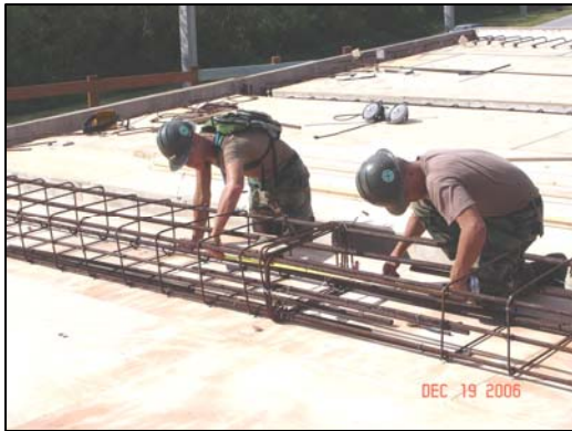
Fig. 34 – Seabees tie steel for overhead placement in Guam.
