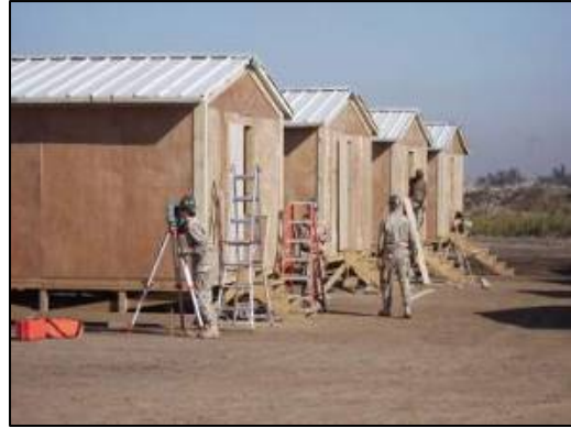
Elevation of Row 8 under construction.
