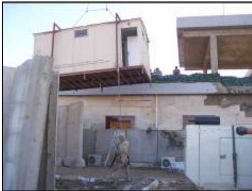
Crane lowers shower trailer into position.
