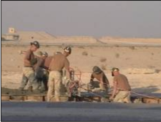
Seabees place and finish concrete on runway.
