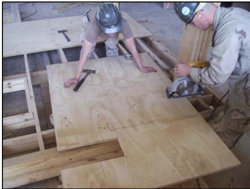
Seabees rip plywood for floor decking.
