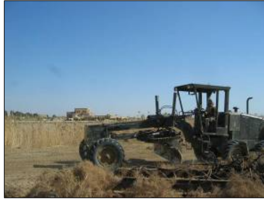
Grading operations to level area for new HESCO barriers.
