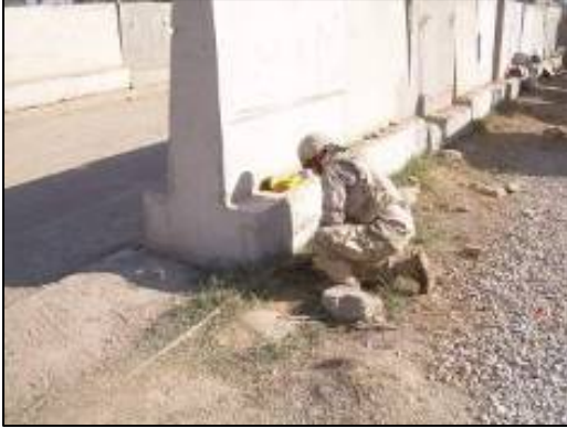
Installation of a 1" waterline to the barracks.
