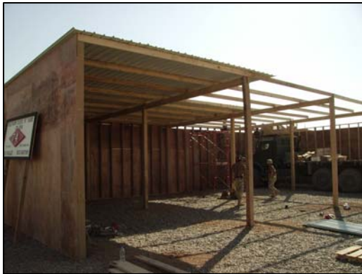
Front elevation of the completed Pole Barn.
