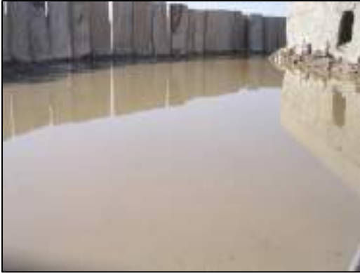
Flooding at COP Qatana prior to fill and walkways being placed.
