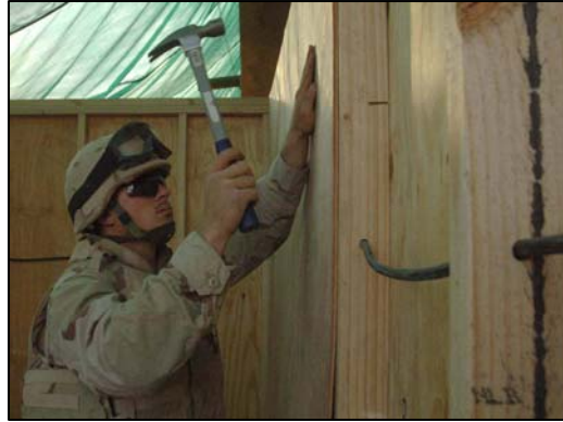
Repair an office space.
