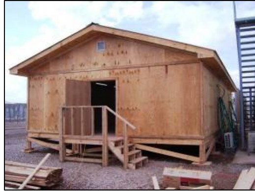
Completed SWA hut.
