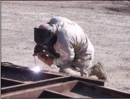
Steelworker places a bead of rod on a steel member.
