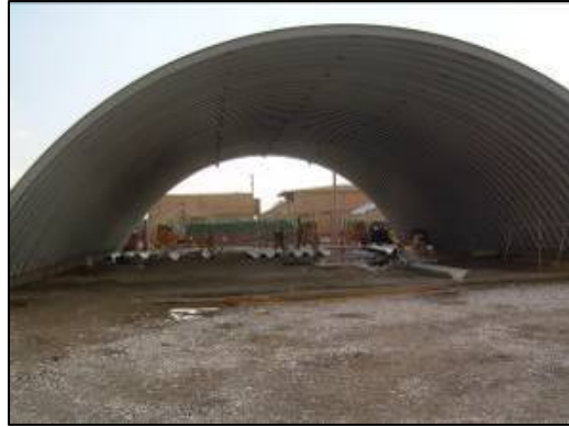
K-Span Arches erected and seamed.
