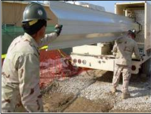
Seabees form K-Span metal with an ABM.
