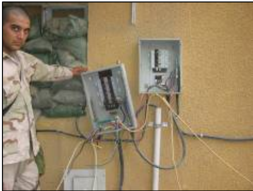
Crew Leader preparing to remove old panel box.
