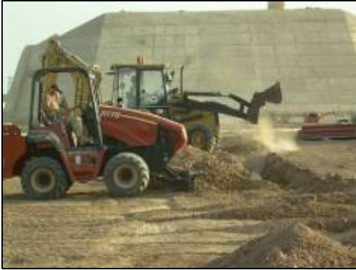
Backfilling fiber optic trenches.
