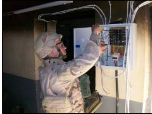
Installation of an electrical panel on site.
