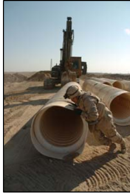
Seabee moves culvert piping into position.
