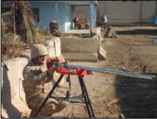
Seabee threads water pipe for installation.
