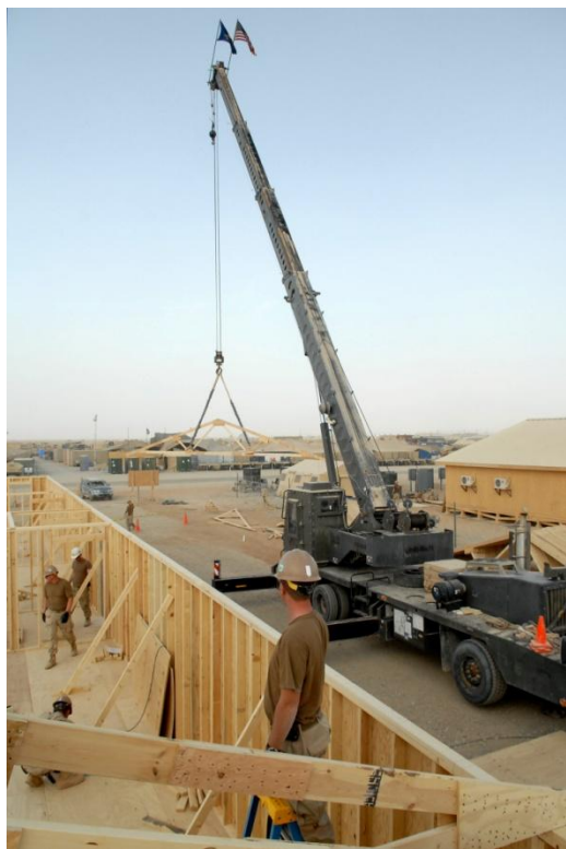
NMCB 74 Crane Crew Lifting Trusses
