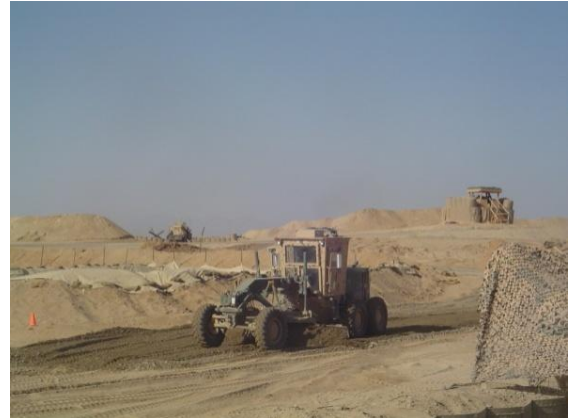
Spreading gravel on road
