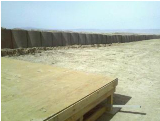
Project site photo where Det4 began construction of seven B-huts with 8 rooms each.
