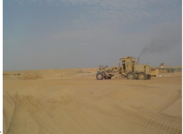
Grading area for the COC Pad
