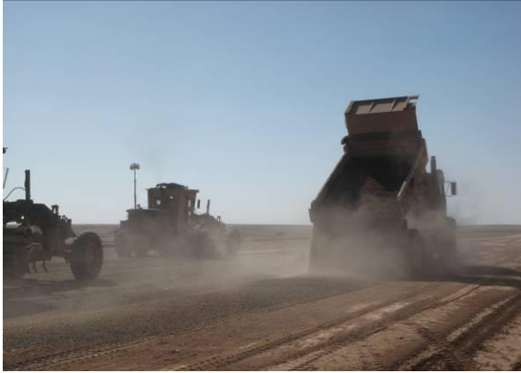
Equipment Operators laying and spreading gravel
