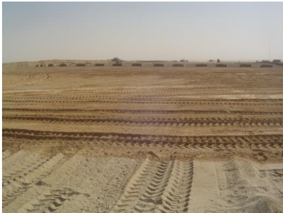
Pad leveled and rough graded
