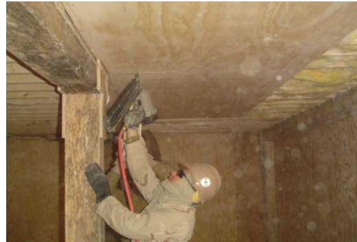
Crew member sheathing ceiling in Hardened COC
