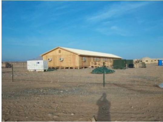
Completed TOC at Delaram
