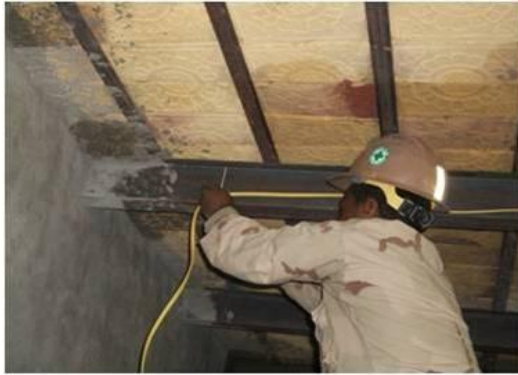
Running Romex on I-beam
