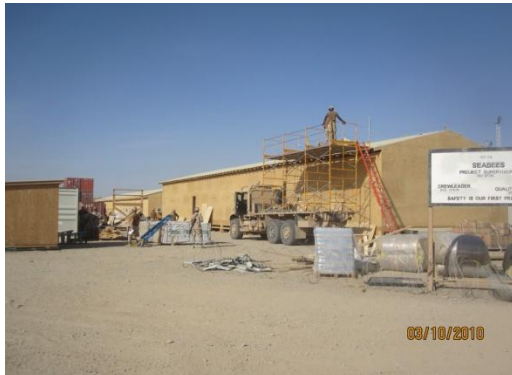
SWA Hut Construction
