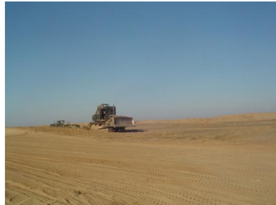
Leveling ground for new HLZ Pad
