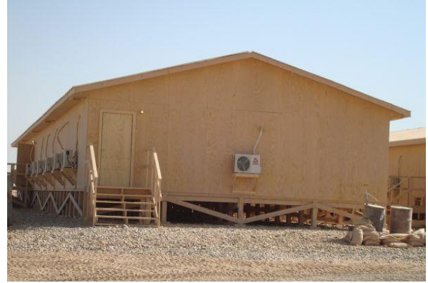
RCT TOC 1 Complete
