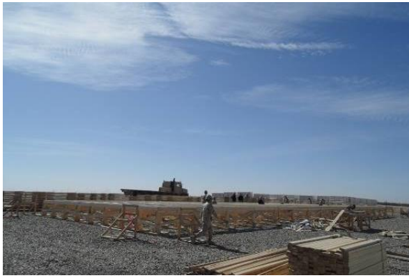
Fire Station under construction
