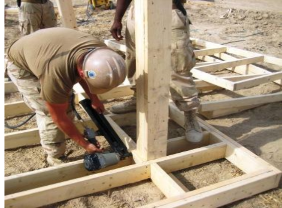
Installing wall studs
