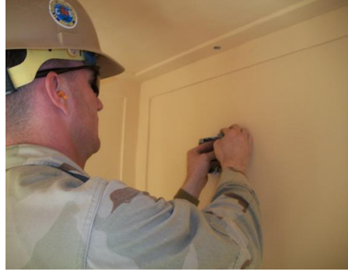
Crew member installing junction box in B-hut.
