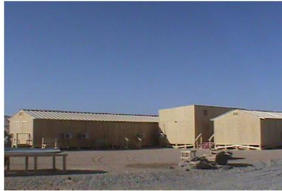
COC pad at project completion
