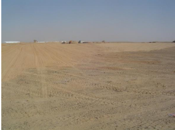
FRSS Pad leveled and rough graded
