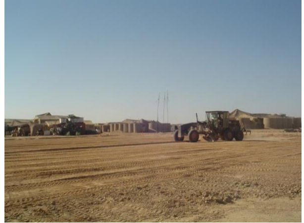
Rough Grading Pad
