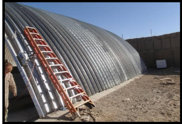
Length of K-Span in place.
