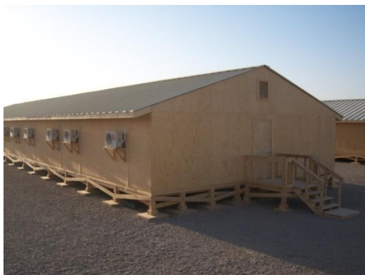
Completed SWA Hut
