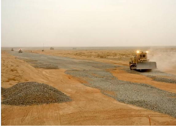
Armored D7 Dozers spreading Gravel.
