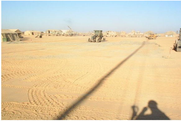
FOB Geronimo at start of site work
