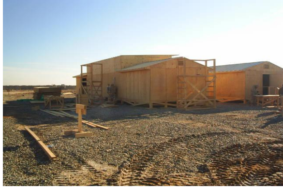
SWA Huts 3 & 4 Nearly Complete
