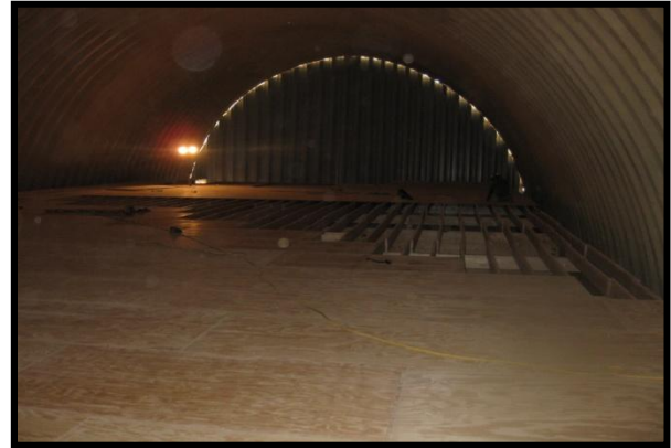
Interior build out.
