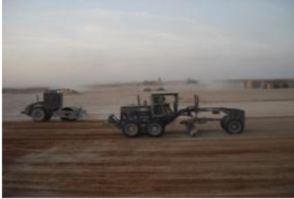
First cuts on Fiddler's Green COC pad
