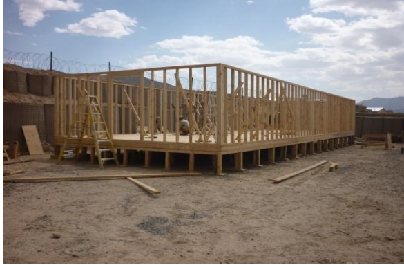
Crew standing the exterior walls of a B-Hut.
