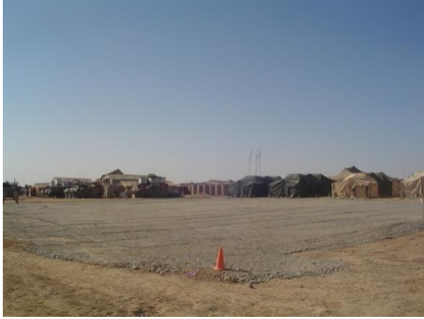
Maintenance Pad Complete
