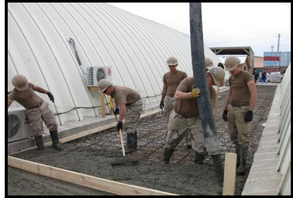
Placement concrete.
