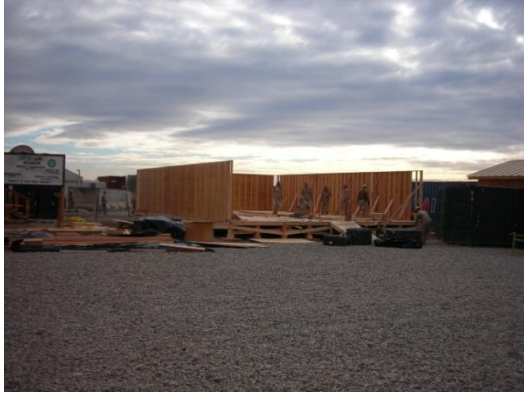
G6 Building inside the 2 nd MEB compound
