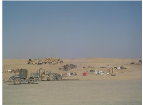
Spreading and compacting gravel on Pad
