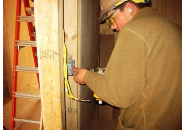
Installing Electrical in SWA Hut
