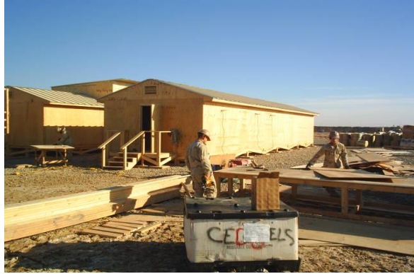
SWA Huts 1 & 2 at Completion
