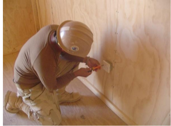
Installing wiring for ANA SWA Hut
