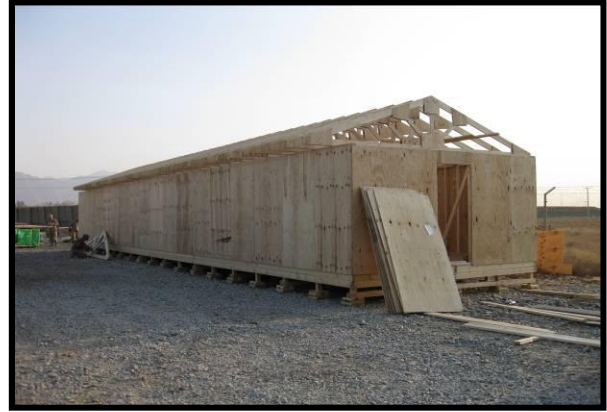
All trusses set.
