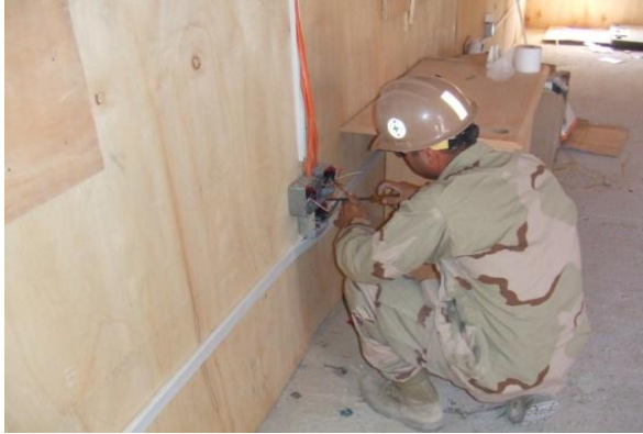
Tying B-Hut into sub panel.
