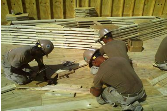
Crew constructing trusses for three B-Huts.
