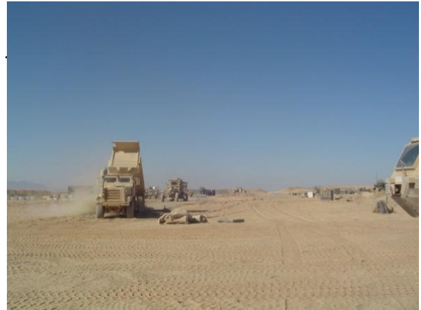
Constructing Main Interior Road
