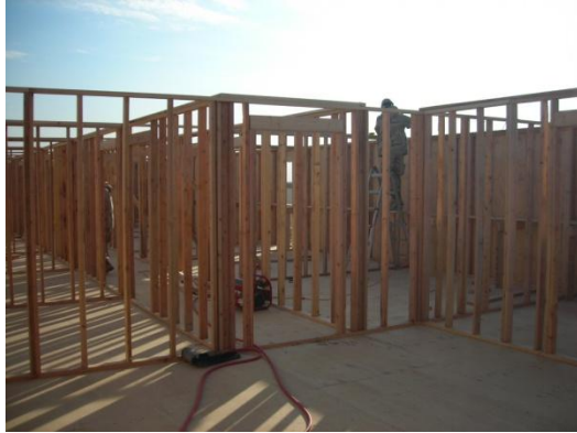
Himar building at the 50%.
