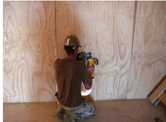
Cutting out door for DG SWA Hut #2
