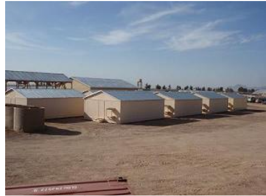
Photo of project site after all B-huts completed, after conducting final BOD.
