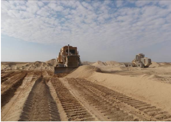
D7 Clearing 4' of sand to find hard surface for road. Grader ripping road to mix gravel for cohesion.
