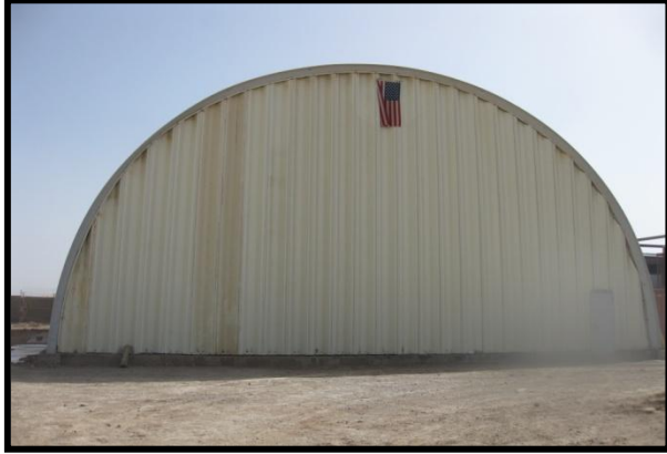
All steel and doors in place.
