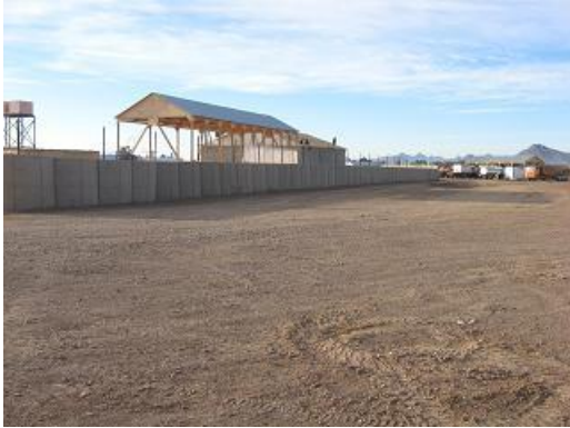
Project site photo where Det4 constructed nine open bay standard B-huts.
