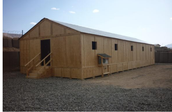
20'x60' B-Hut with 9 rooms completed.
