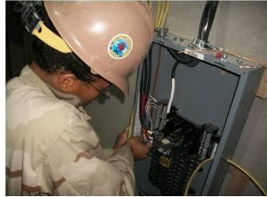
Making connections in panel.
