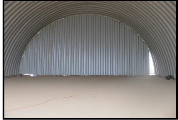
Interior view of Gym K-Span.
