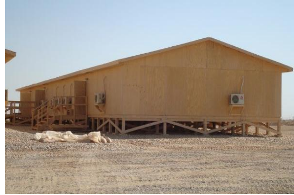
RCT TOC 2 Complete
