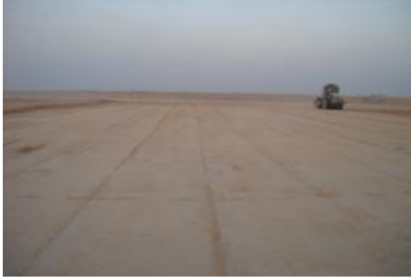
COC pad prior to construction
