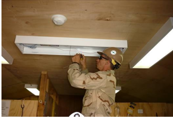
Crew installing interior lighting.
