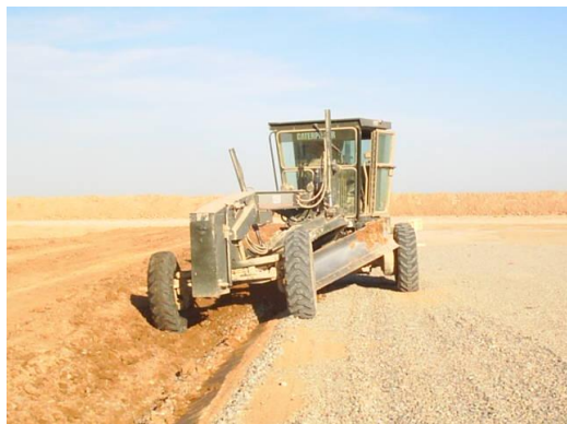
Grading Surface Course
