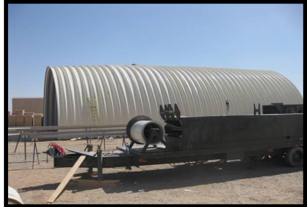
K-Span length complete.
