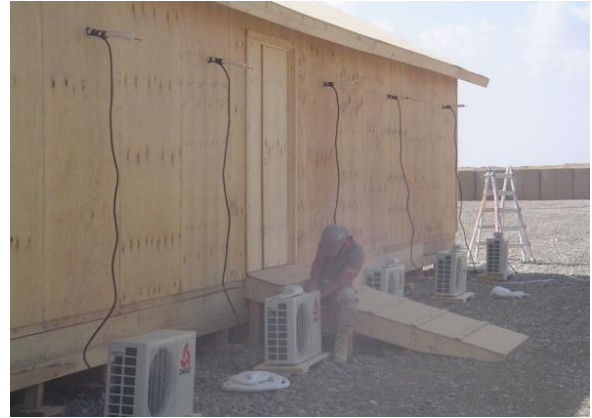
Installing CHIGO split type A/C units
