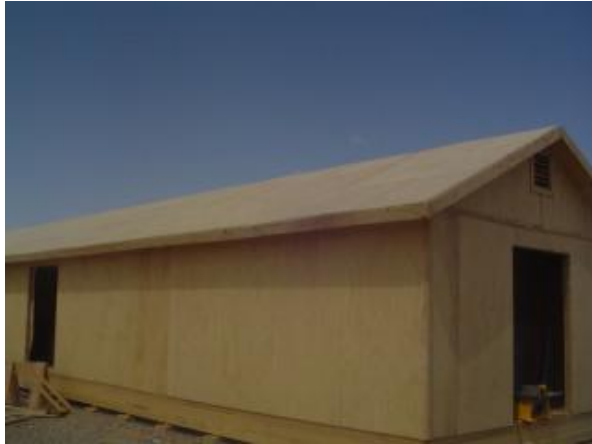
SWA Hut near completion
