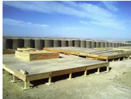
Photo of B-hut #5 prior to conducting BOD.
