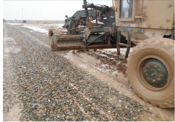
D7 Clearing 4' of sand to find hard surface for road. Grader ripping road to mix gravel for cohesion.
