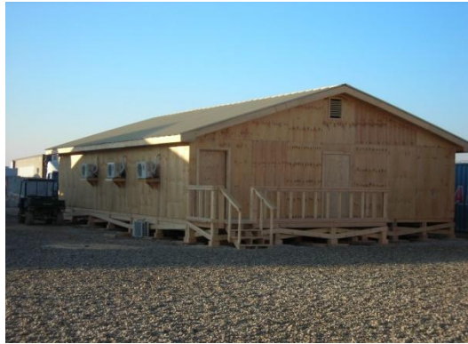
G6 Building inside the 2 nd MEB compound
