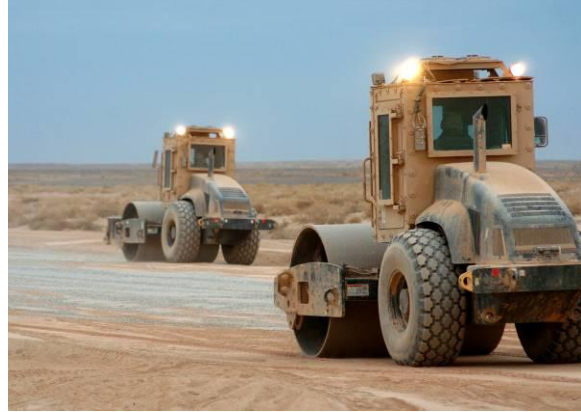
Armored Rollers compacting the road.
