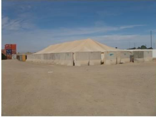
GCE-1 BUILDING AT PROJECT START
