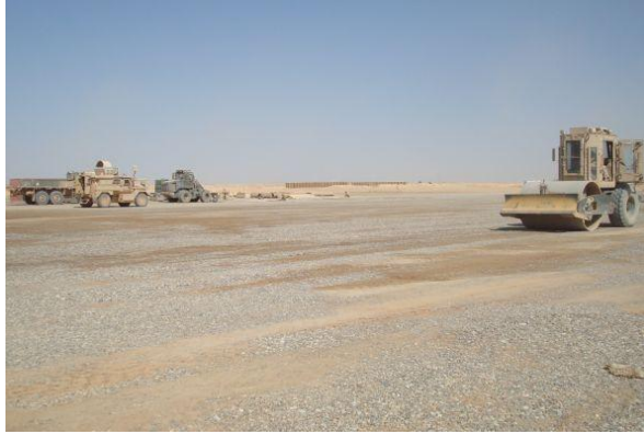
CLB TOC during Site Prep
