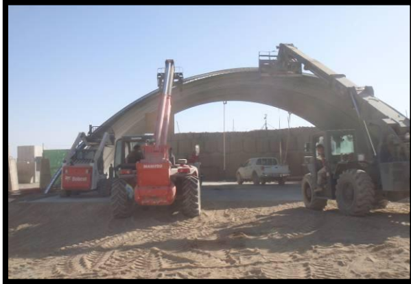
Lifting section in place with extend a boom forklift.
