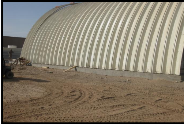
Completing the standing of steel.
