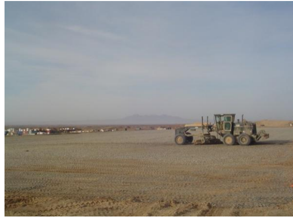
Grading LSA Pad
