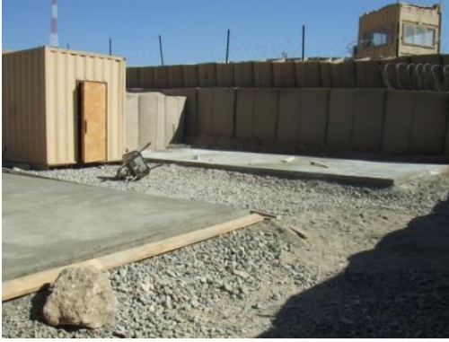
Project site photo where Det4 constructed three standard B-huts.
