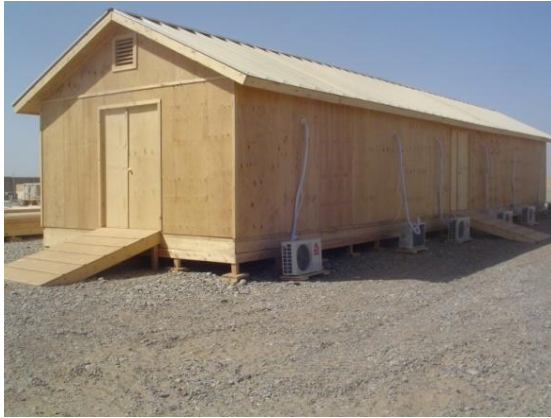
BAS/STP SWA Hut Complete
