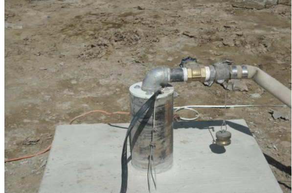
Water Well #1 Complete
