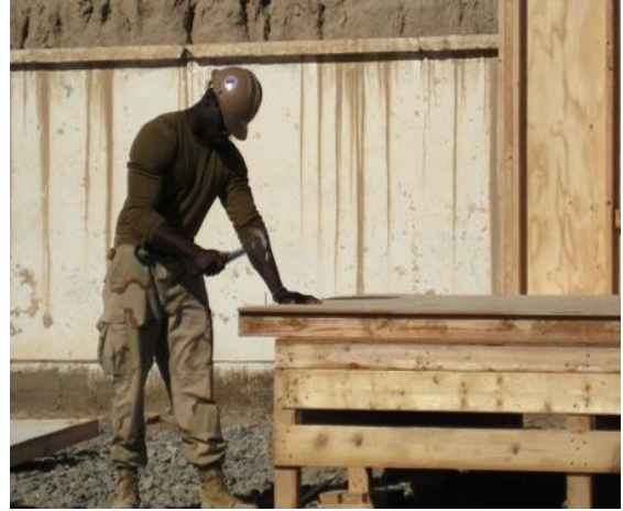
Working on wall section for SWA Hut
