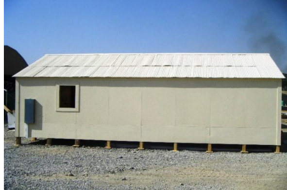
Completed 20'x32' B-Hut #3 with window.
