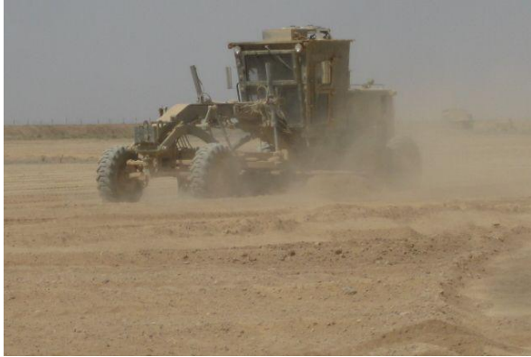
A/DACG Pads – typical initial condition
