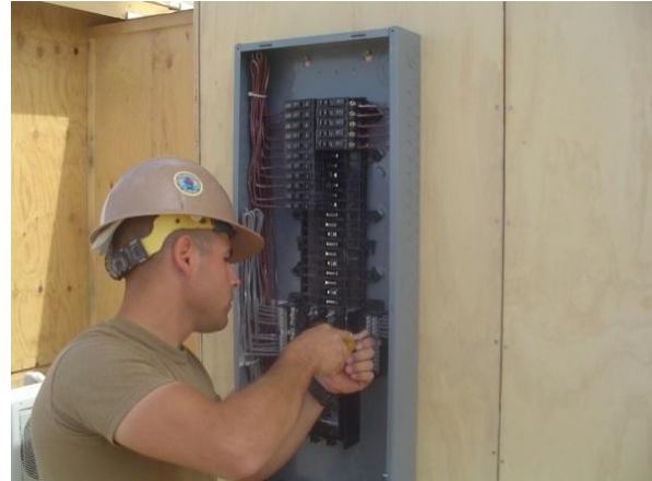
Crew wiring Main Panel
