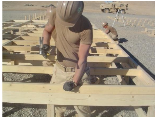
Crew members constructing subfloor
