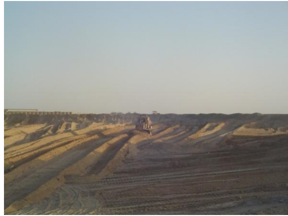
Leveling ground for HLZ Fuel Farm Bladder
