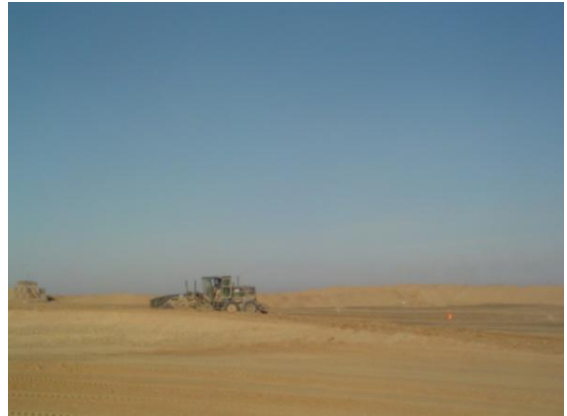
Rough grading FRSS pad
