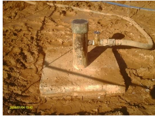
Water Well #1 Complete
