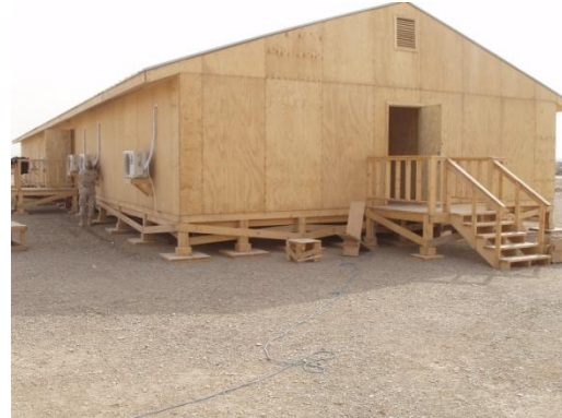
COMMS BUILDING AT COMPLETION
