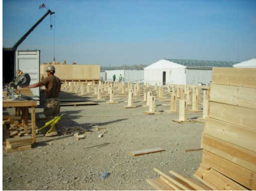
GCE HQ building at 5 %
