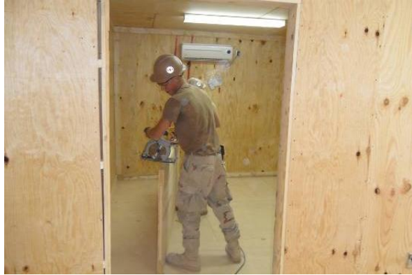
Seabees preparing to hang doors
