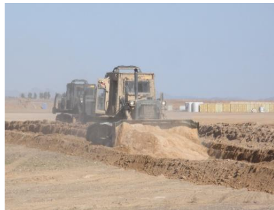
Moving Dirt at Delaram
