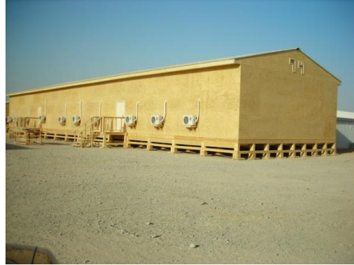
GCE HQ after move out.
