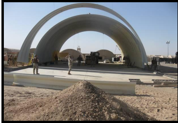
Crane bringing section into place.
