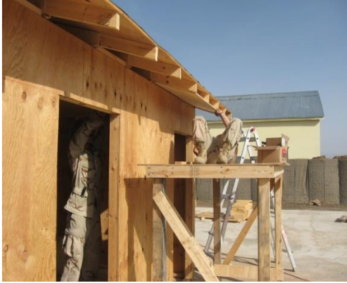
Project site photo where Det4 constructed One 7 room 20'X32' B-hut.
