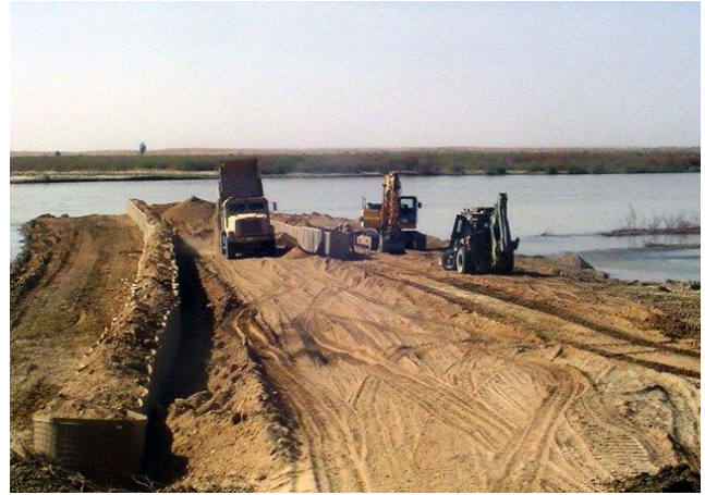
Placing fill as sub-base for Causeway
