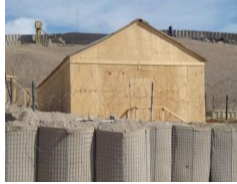
Photo of B-hut #3 prior to conducting BOD.
