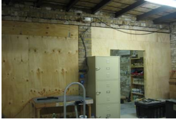
Completed Armory walls.
