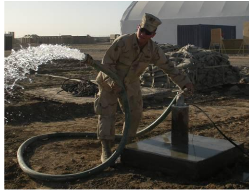
Water Well #2 Complete
