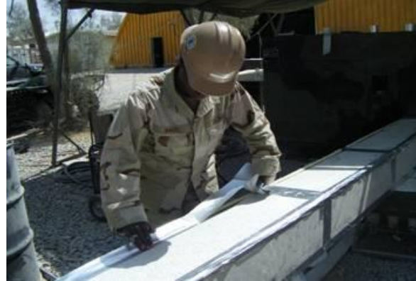
UT assembling main stack for AC for SCIF.
