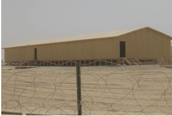
RCT TOC 1 at Turnover
