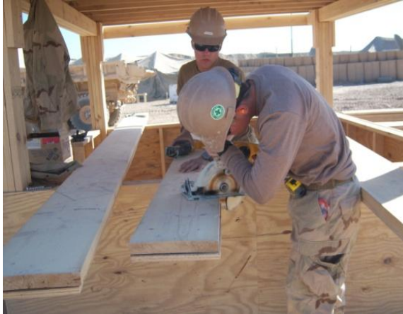
Crew members working on cutting stairs for Crow's Nest
