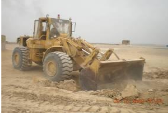
Crew clearing and grading for expansion.
