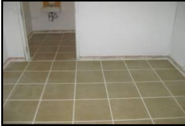
Project Overview: Bunk Room and Head Renovation
