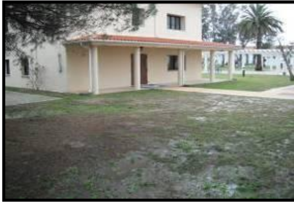
Project Overview: Prior To Construction
