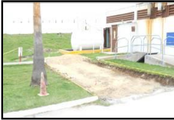
Project Overview: Prior to Construction
