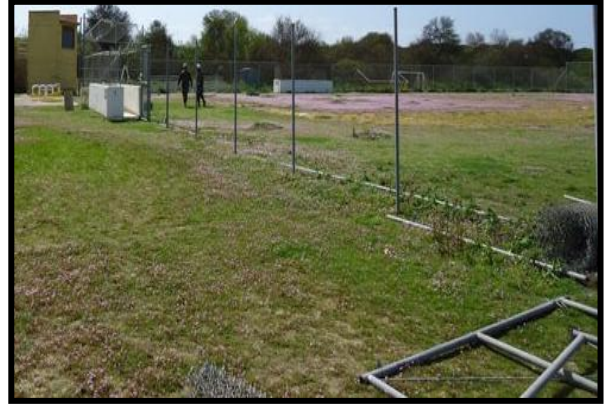
Project Overview: Clearing Fence for Project Finish
