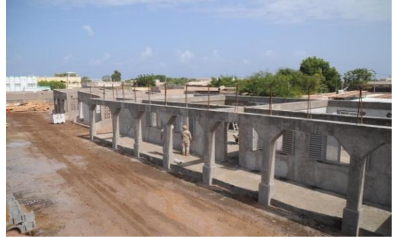
Ecole 5 School Construction in Camp Lemonnier
