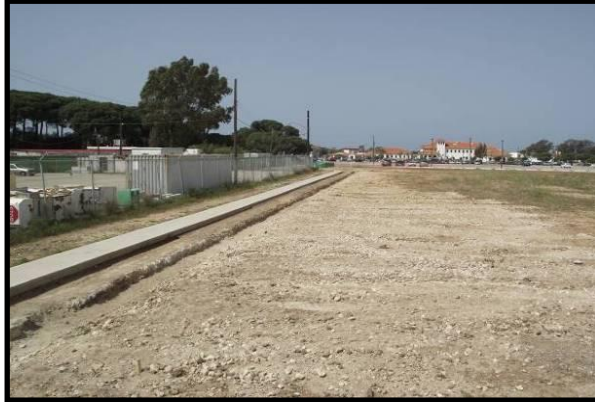
Project Overview: Prior to construction
