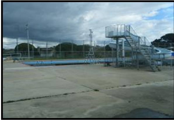
Project Overview: Prior to construction
