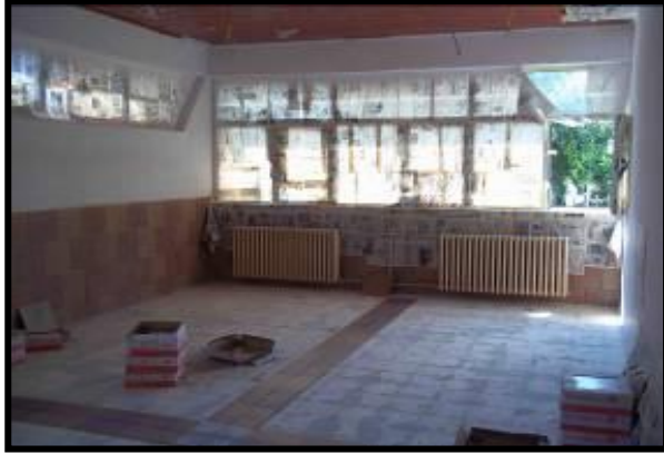
Project Overview: Demolishing Interior Tile
