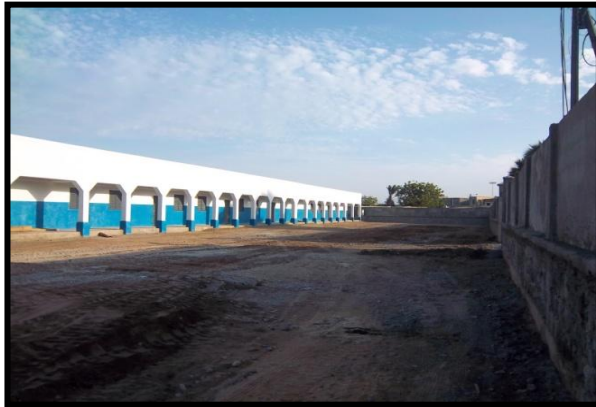
Project Overview: Project Site Facility
