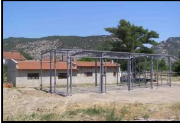
Project Overview: Project Steel Structure
