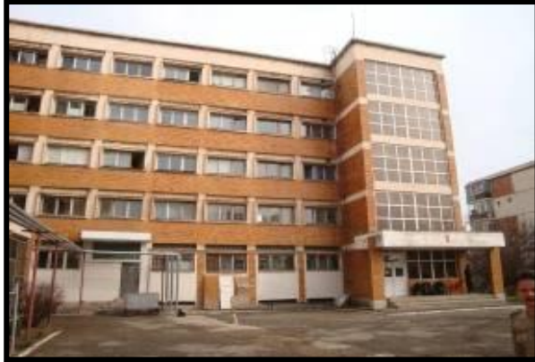
Project Overview: Exterior Prior to Construction
