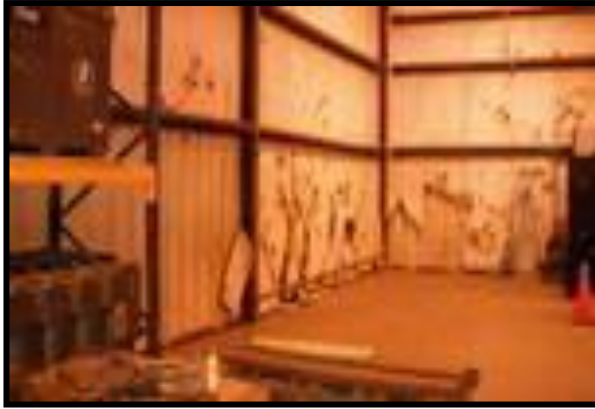
Project Overview: Prior to Construction
