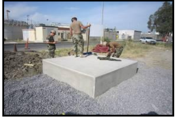
Project Overview: Prior to Construction
