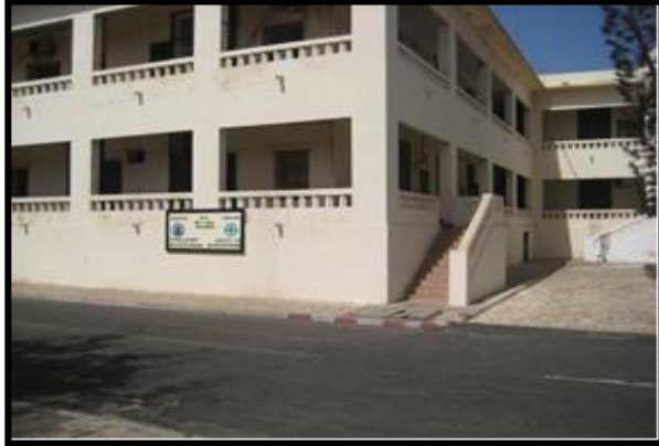
Project Overview: Exterior Prior to Construction
