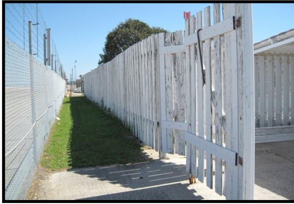
Project Overview: Prior to Construction
