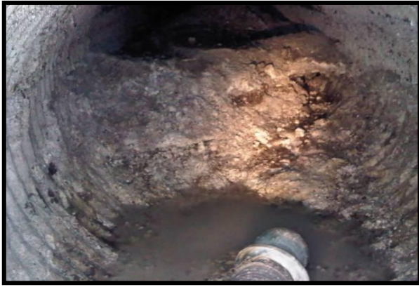
Project Overview: Prior to Removal of Sediment
