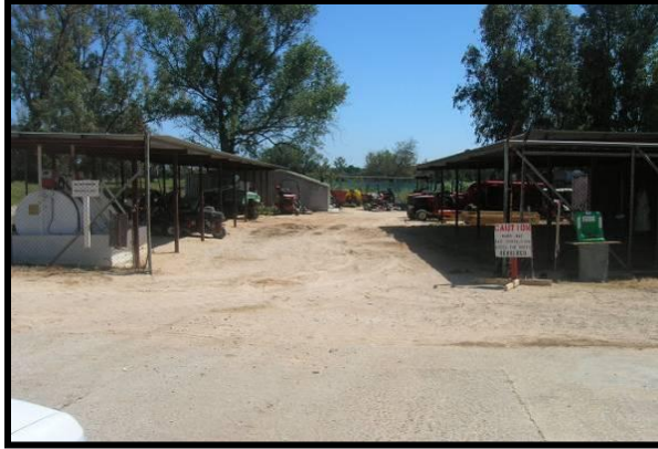
Project Overview: Prior to Construction
