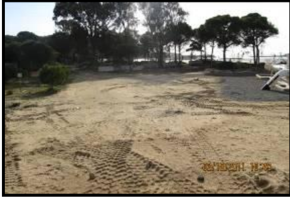
Project Overview: Prior to Paving
