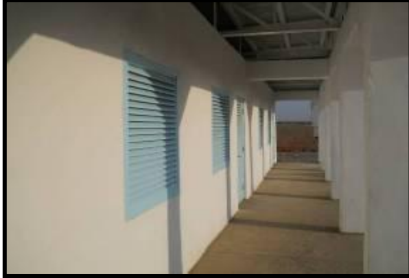
Project Overview: Project Site Facility
