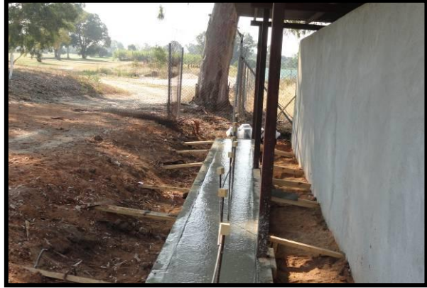
Project Overview: Poured Footers
