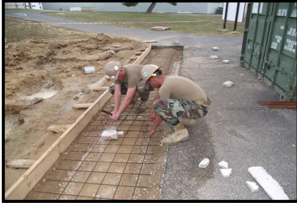
Project Overview: Form Work
