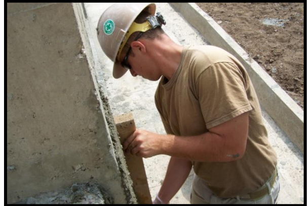
Project Overview: Stucco Is Applied to Walls
