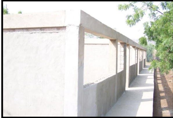
Project Overview: Project Site Facility
