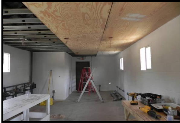
Project Overview: Early Phase of Construction
