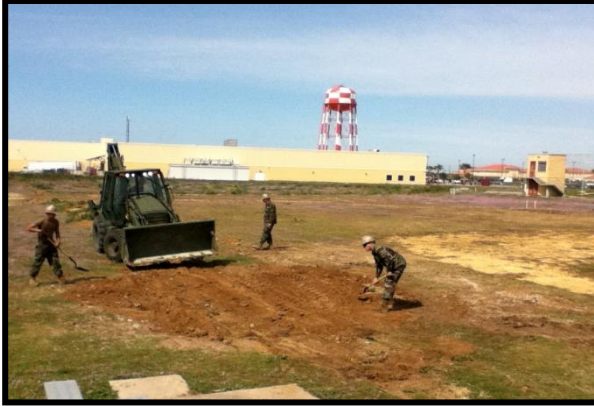
Project Overview: Demolition Operations
