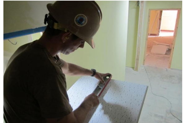
Renovation of Ops Center (Dakar, Senegal)
