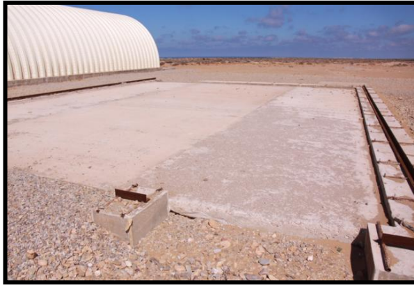
Project Overview: Prior to Construction
