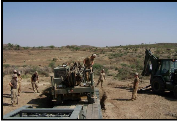
Project Overview: Prior to Construction
