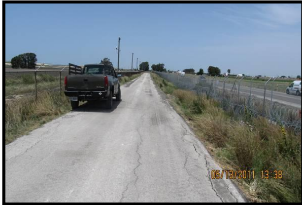
Project Overview: Prior to Paving
