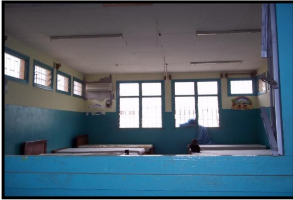
Project Overview: Existing Room
