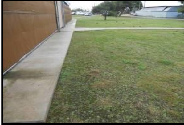
Project Overview: Prior to Construction
