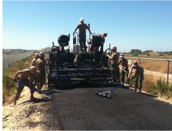
Perimeter Road Paving Operations
