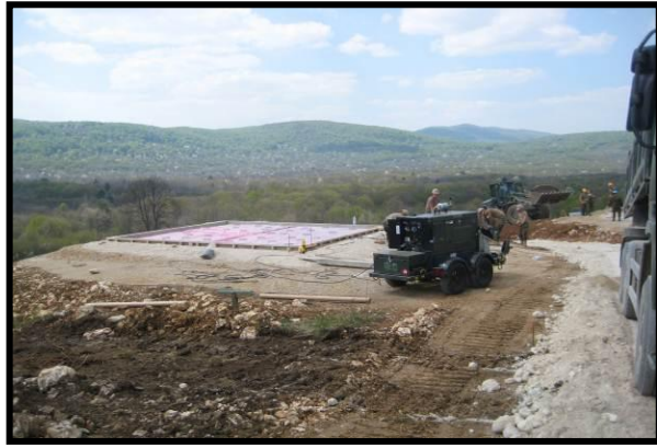
Project Overview: Formwork for pad Slunj, Croatia
