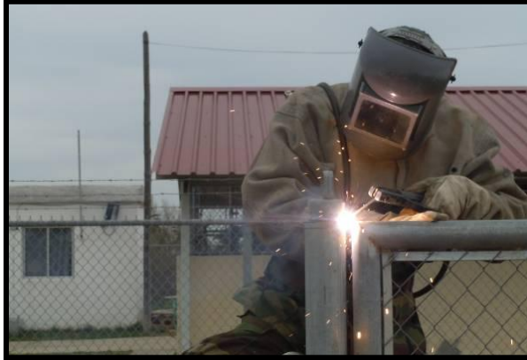
Project Overview: Fence Construction
