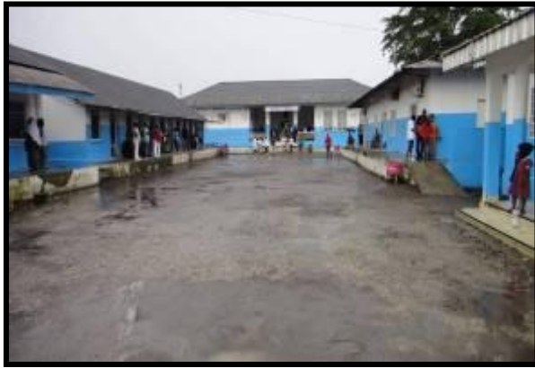
Project Overview: Prior to Construction
