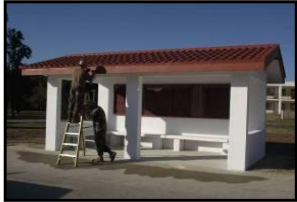
Project Overview: Project Ready for Turn-Over
