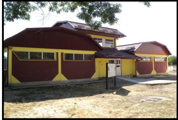
Project Overview: Renovation Project Complete
