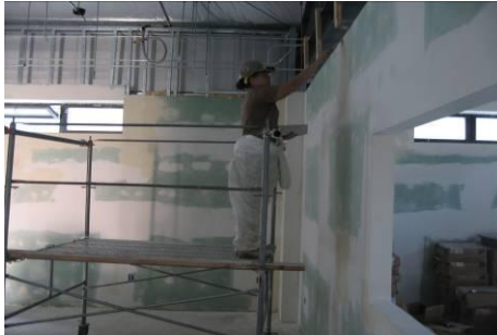
CN Rech applying joint compound
