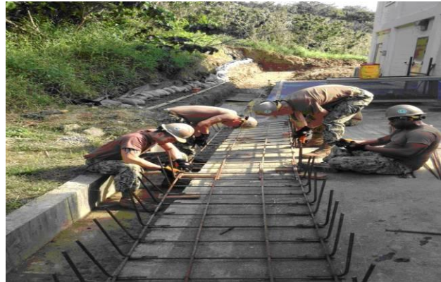
Project at Turnover
