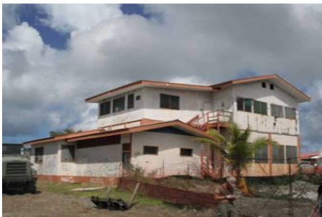
Initial Site Conditions
