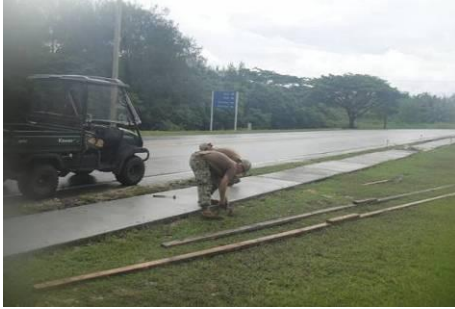
Initial Site Conditions
