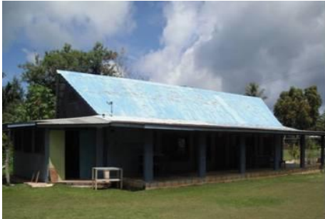
Initial Site Conditions
