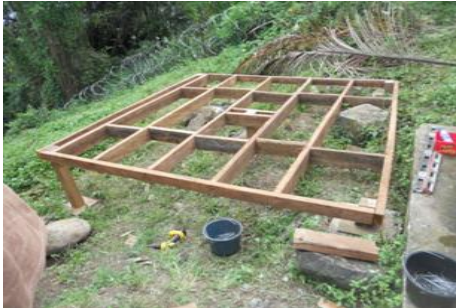
Initial Site Conditions
