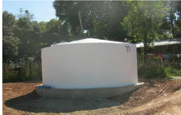
Project at Turnover
