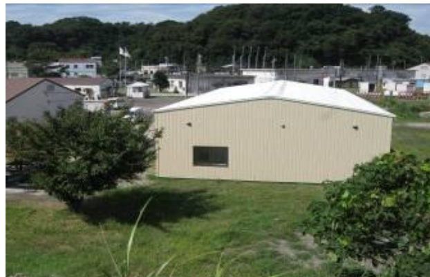
Building at turnover with NMCB 5
