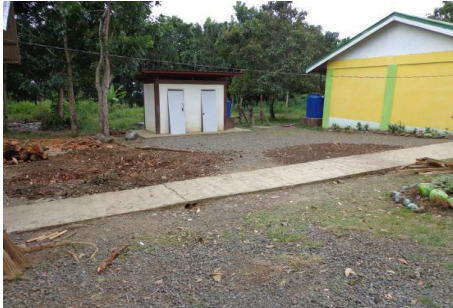
Initial Site Conditions
