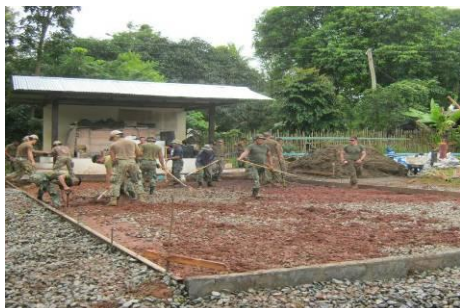
Initial Site Conditions
