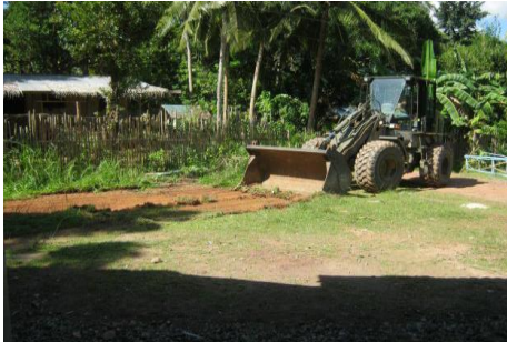
Initial Site Conditions
