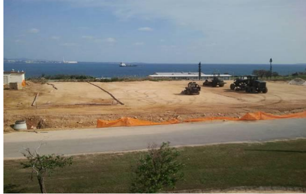
Project at Turnover with NMCB 5
