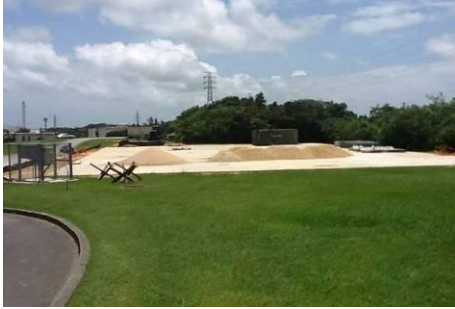
Project at turnover with NMCB 40
