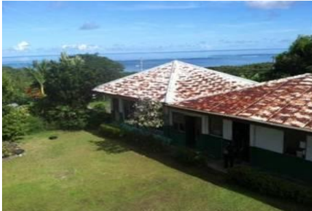
Initial Site Conditions
