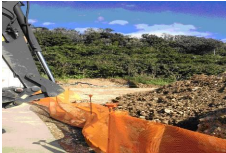
Initial Site Conditions
