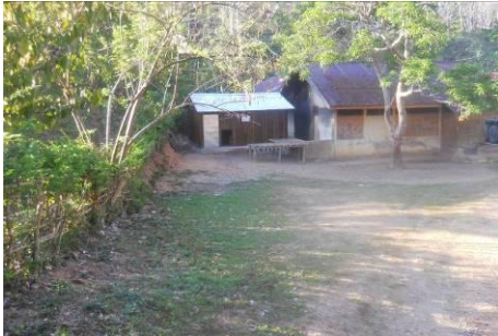
Initial Site Conditions
