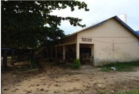
Initial Site Conditions
