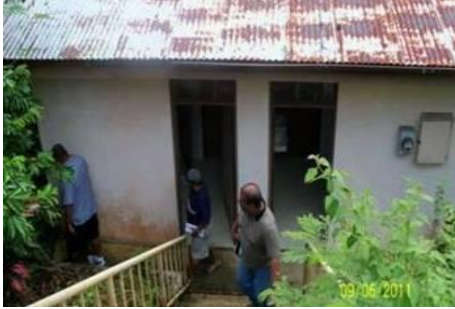
Initial Site Conditions
