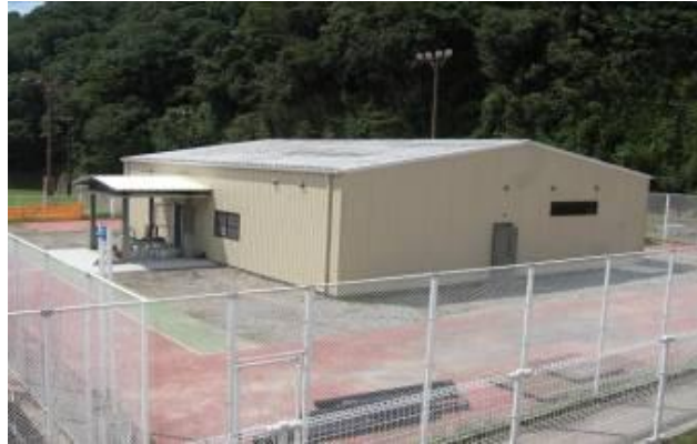
Building at turnover with NMCB 5
