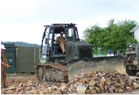
Spreading base course
