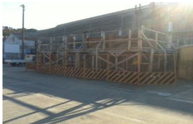
Project at turnover with NMCB 5
