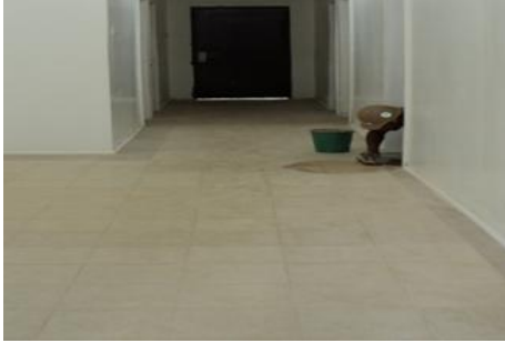
Initial Site Conditions
