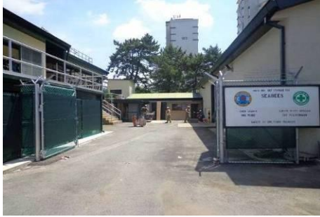
Initial Site Conditions
