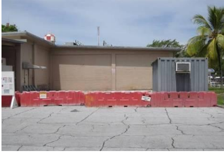
Initial Site Conditions
