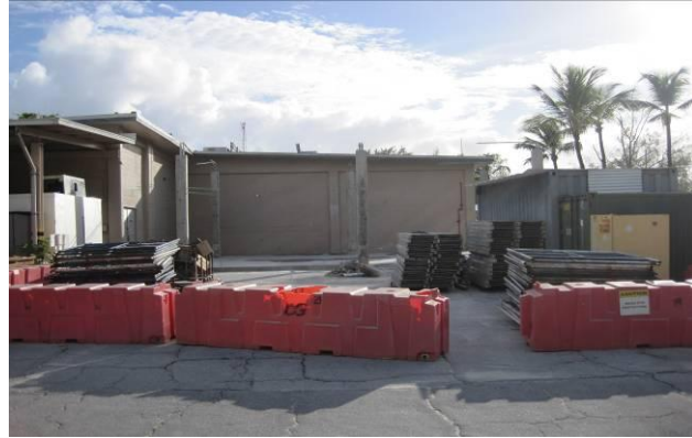
Site Conditions at turnover with NMCB 5
