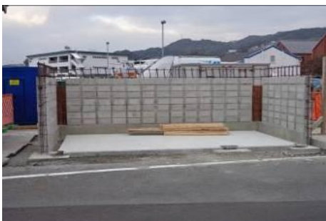
Initial Site Conditions
