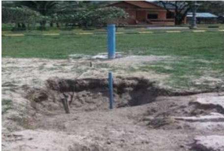
Initial Site Conditions
