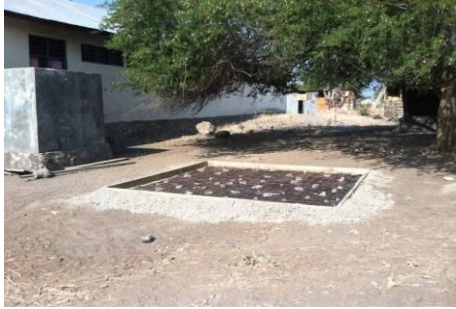
Initial Site Conditions
