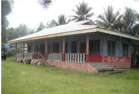
Initial Site Conditions
