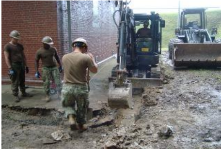
Excavation of existing drainage ditches.
