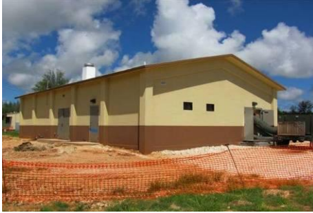
Initial Site Conditions
