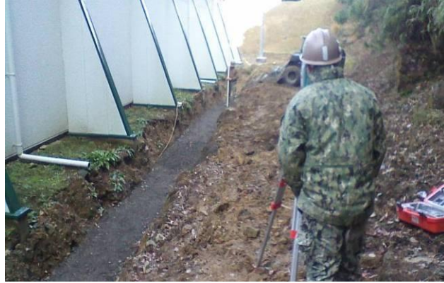
Project at Turnover
