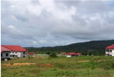
Initial Site Conditions
