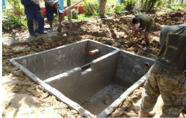
Tagbueros Septic Tank prior to fitting top
