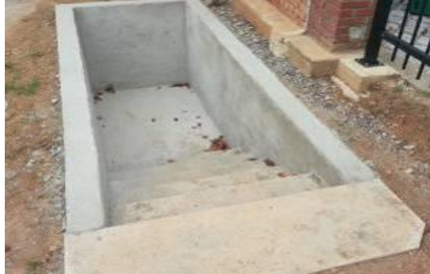
Completed Hardened Bunker
