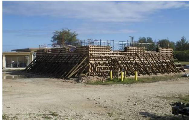
Project at Turnover
