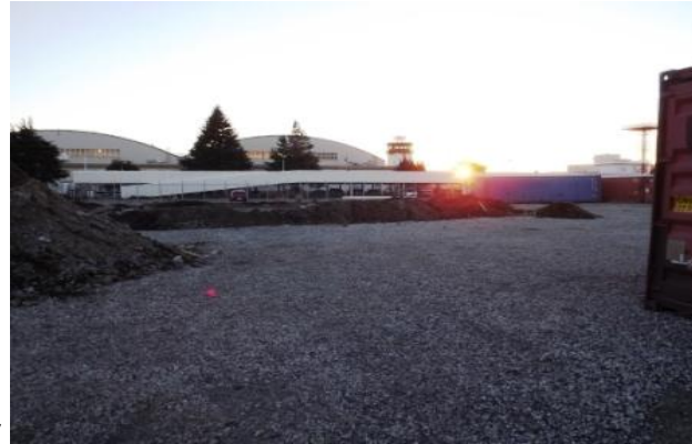
Site Condition at Turnover
