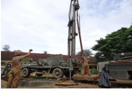
Adding another piece of drill steel
