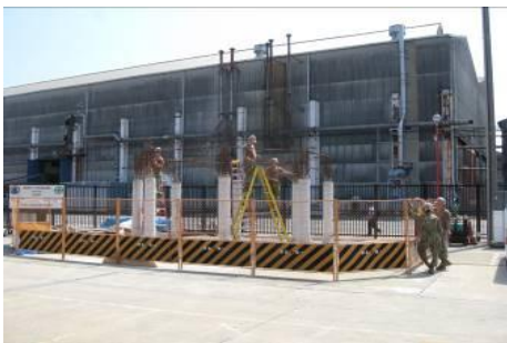
Initial Site Conditions
