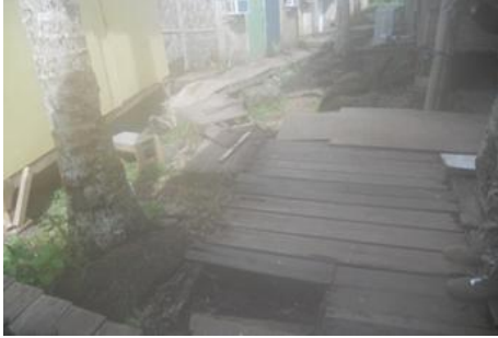
Initial Site Conditions
