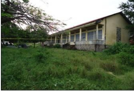
Initial Site Conditions
