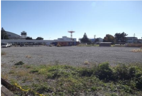
Initial Site Conditions
