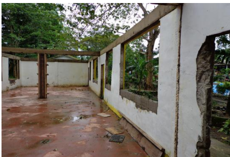
Initial Site Conditions
