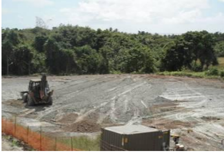
Initial Site Conditions
