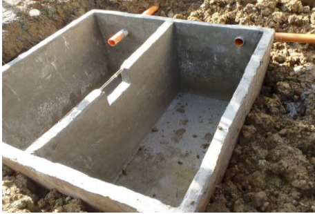
Septic tank after initial placement
