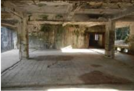
Empty Second Floor of Building
