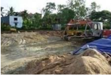
Initial Site Conditions
