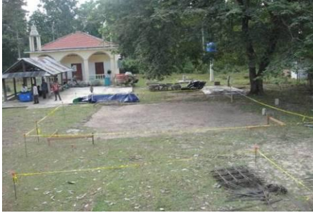
Initial Site Conditions
