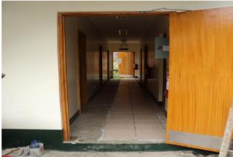
Initial Site Conditions
