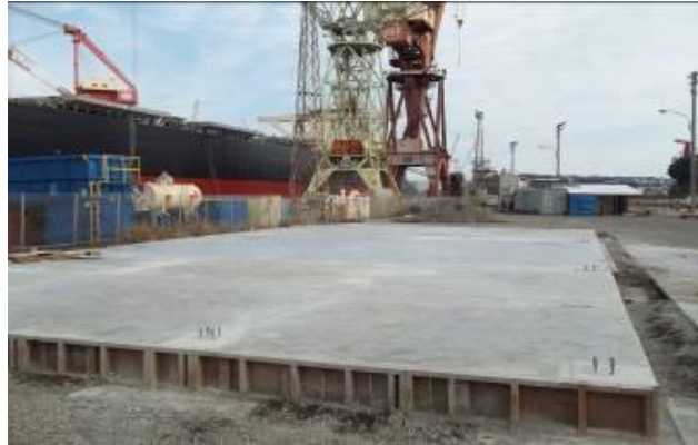
Project at Turnover
