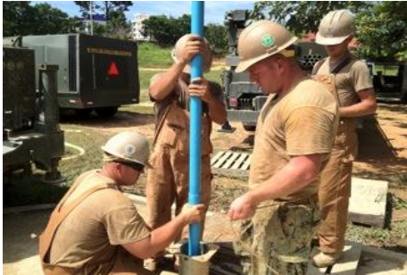
Water well team installs new PVC pipe
