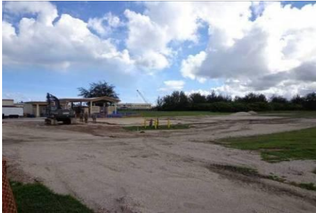
Initial Site Conditions
