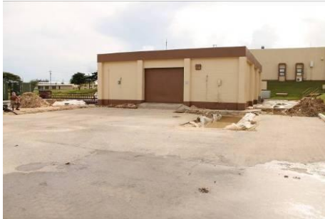
Initial Site Conditions
