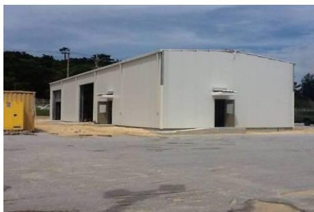
Initial Site Conditions
