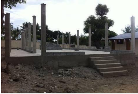
Initial Site Conditions
