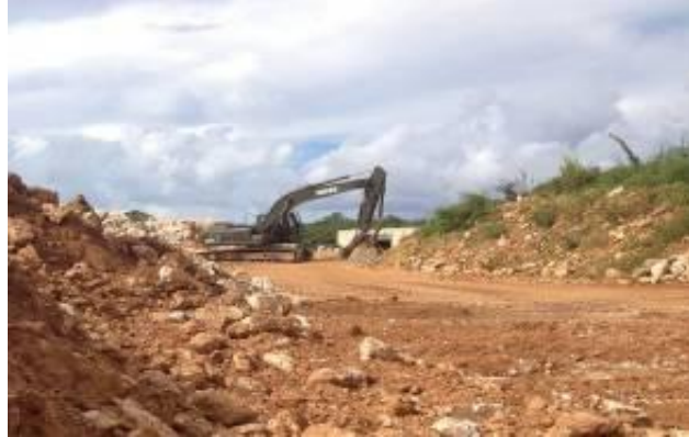
EO3 Lawrence operating an excavator
