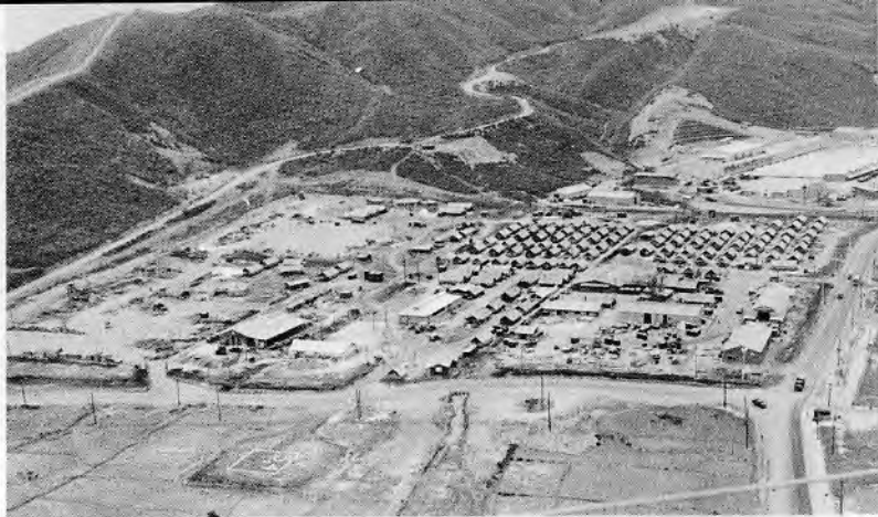
Camp Hoover, Danang Main, (above) was base camp for NMCB 9's third consecutive deployment to the Republic of Vietnam. It was from this location that a detail deployed to Phu Loc to construct and develop the Seabees largest quarry-crusher site in the Republic at Phu Loc, north of Hai Van Pass.
