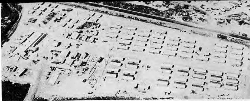
Cantonments were the "order" of the day during NMCB 11's Quang Tri deployment. Above is ELEVEN's camp while below center is a new cantonment being built under the MER Program.
