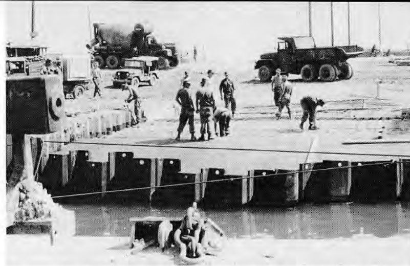
Seabees from NMCB-3 prepare the concrete ramps at the Danang harbor Bridge Ramp project. In the two photographs below, Seabees participate in the MER program in the northern I Corps where prefabricated construction is the word of the day. In the bottom photograph, Seabees erect the prefabricated SEA huts at a new MER cantonment somewhere north of Hue City.
