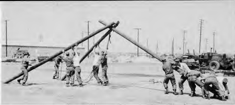
Seabee Team 0913 (above) erects a tripod as part of the rigging phase of their training.
