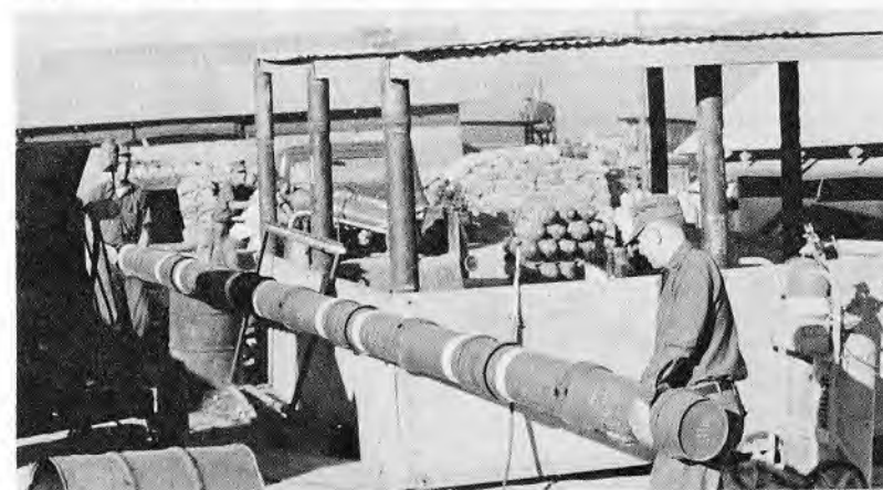
Seabees from Detail ALFA at An Hoa carry a power line pole fabricated by welding used ammunition cannisters end to end. Back at Dong Ha (bottom), Seabee "muscle power" is used to relocate a quonset hut.
