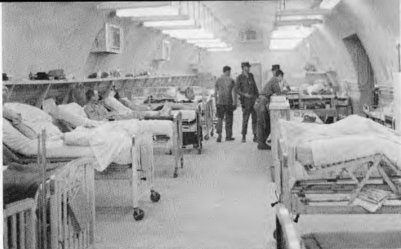
While upgrading the Second Surgical Hospital at Chu Lai, the Seabees hardly had time to remove their tools before the wards were occupied. Shown here is the just completed intensive care ward built by NMCB 40.
