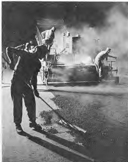
Seabees laid asphalt on highways in the I Corps at night to avoid heavy traffic congestion in the daytime hours.
