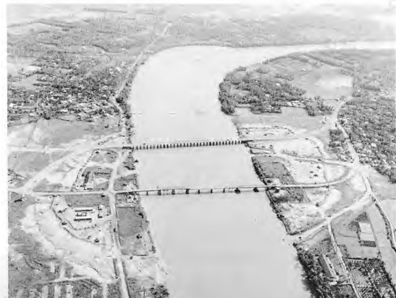
The completed 780-foot An Lo Bridge (below) is a vital link to combat forces in the I Corps. The bridge it replaced is in the foreground of the photograph.
