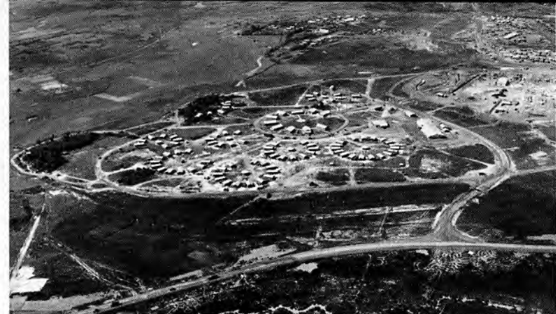
This is an aerial view of NMCB 4's Camp Haines' administrative and berthing areas on the edge of the huge Camp Evans Combat Base north of Hue.
