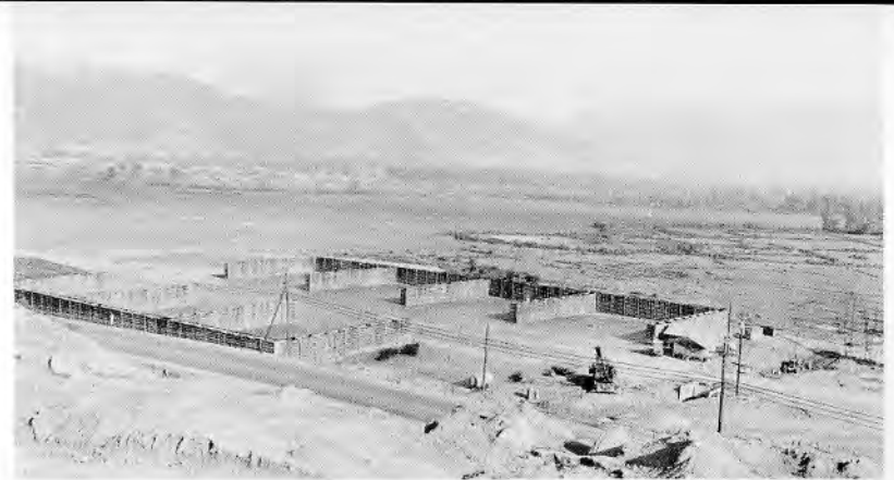
Above is a reveted helo pad built to house CH-54 "Flying Cranes" for the 478th Aviation Company of the U. S. Army.
