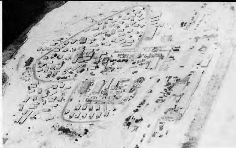
NMCB 128 made Camp Faulkner, Danang East (above) its home from October 1967 until July 1968. A few months after the battalion departed Vietnam the Camp was decommissioned by NMCB 3.
