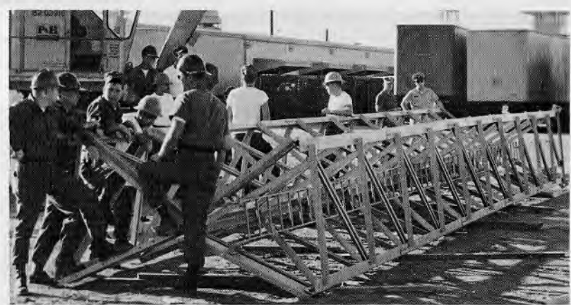
Homeport training is also a time for experimenting with new products. Here an Ammi-Tower is utilized for the first time by a Seabee crew.
