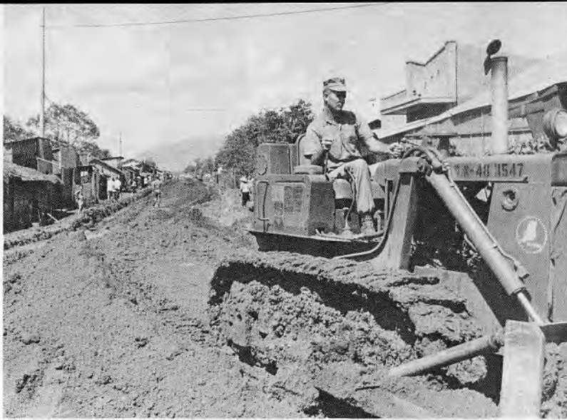
EO1 C. R. Webb from Seabee Team 0912 spreads fill for the Hoang Dieu Street project at Xuan Loc City above. In the photograph below, Seabees from 7101 constructed this 280-foot cable suspension bridge at Phu My Village across the Ba Bao Canal for pedestrian traffic.
