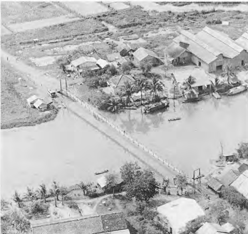
EO1 C. R. Webb from Seabee Team 0912 spreads fill for the Hoang Dieu Street project at Xuan Loc City above. In the photograph below, Seabees from 7101 constructed this 280-foot cable suspension bridge at Phu My Village across the Ba Bao Canal for pedestrian traffic.
