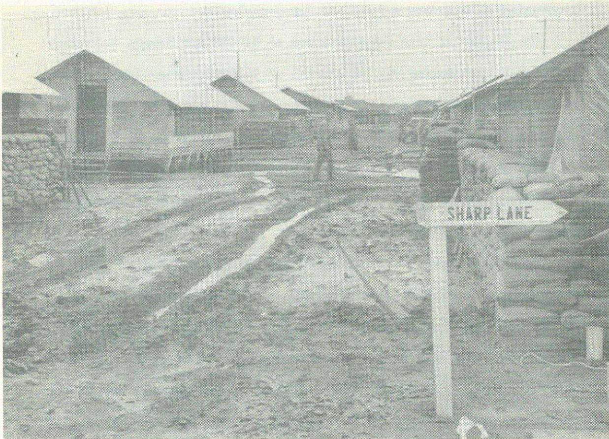
Navy berthing facilities at Dong Tam.
