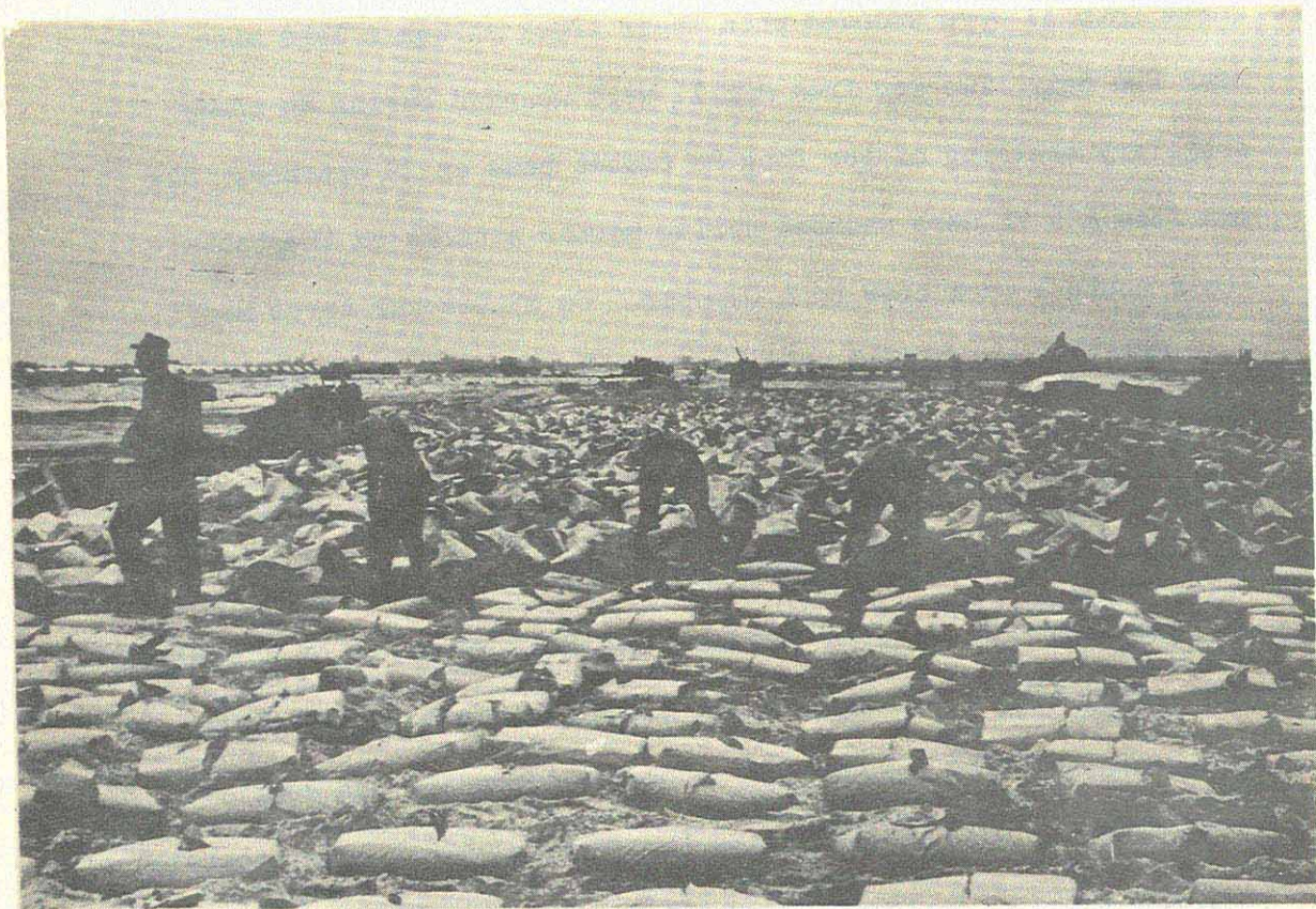
Seabees spread cement used to produce a soil base for the new airstrip at Dong Ha.
