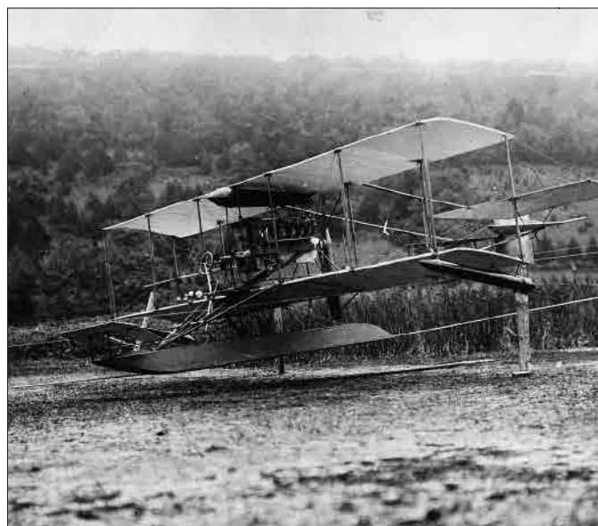
Preparing A-1 for a launch from an inclined wire rigged from the beach down to the water at Hammondsport, N.Y.
