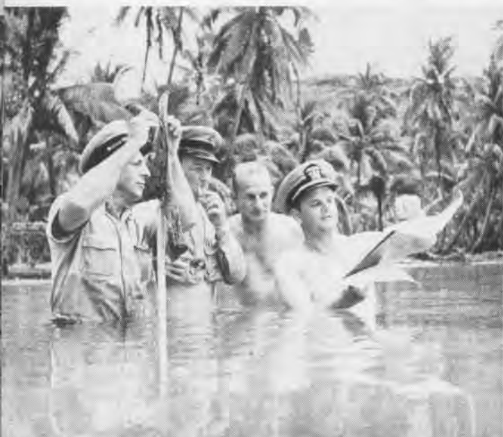
DAMP conditions fail to slow up these men laying out plane runway ramp on South Seas island
