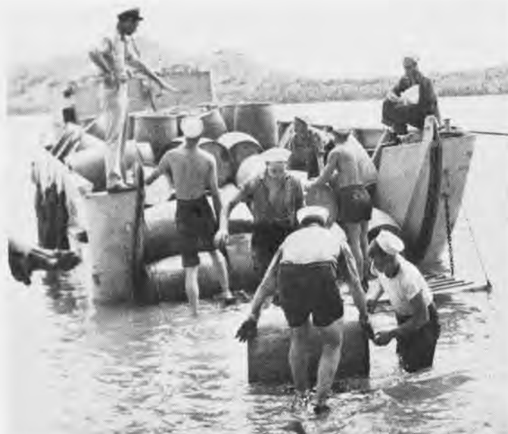
STEVEDORE work, unloading gas for Navy's planes, one of many tasks done by the Seabees
