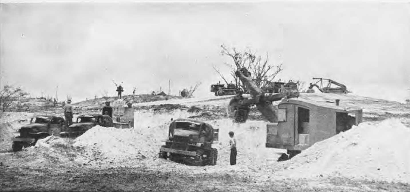
◆ Seabees, using coral for surfacing, started rebuilding bomb-blasted field after capture August 5 ◆ Nine days later Marine pilot landed Corsair on strip and Munda Point became advanced Allied base
