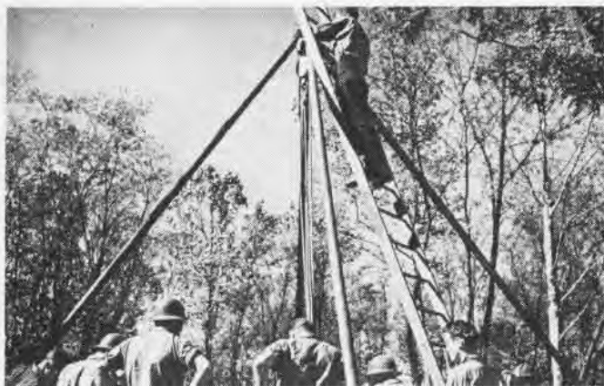
1 DEEP SHAFT , sometimes 35 feet down, needed to reach and neutralize dud projectiles or bombs
