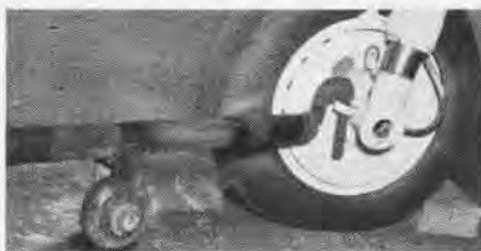
BAR ENABLES ONE MAN TO DO PLANE TOWING JOB
