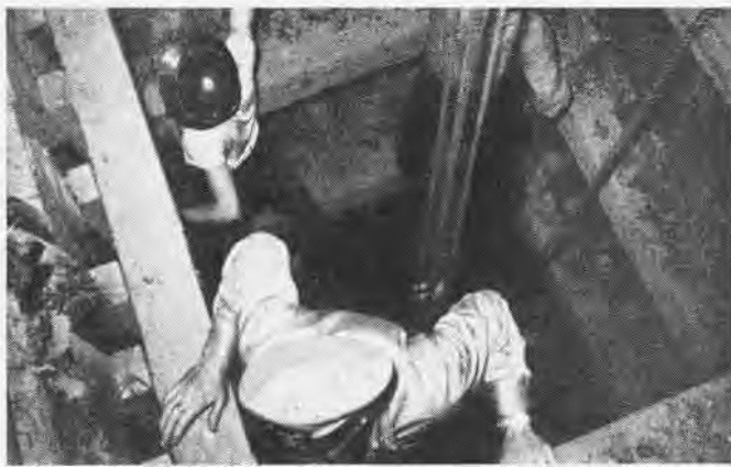
2 STRONG TIMBERING keeps shaft from caving in; crews use no nails in shoring up their pits
