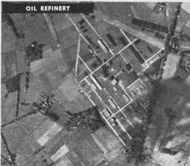
German decoy oil refinery with elaborate layout of three-dimensional structures simulating real target. Photo shows lack of activity
