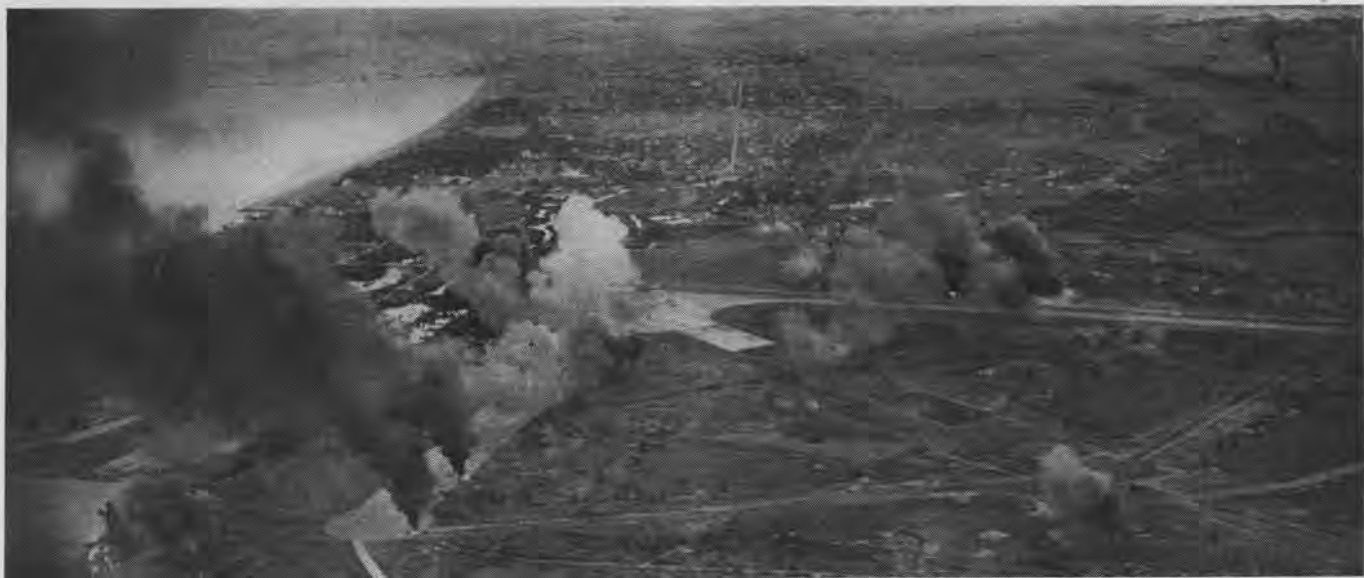
NICHOLS FIELD, 5½ MILES SSE OF MANILA HAD TWO COMPLETED CONCRETE RUNWAYS. THIRD WAS UNDER CONSTRUCTION IN CENTER
