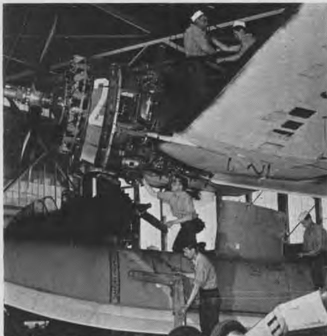
THROUGH Fleet Supply Officer, SOSU gives new units planes. All arrive with landing gear. Wheels are removed, floats installed
