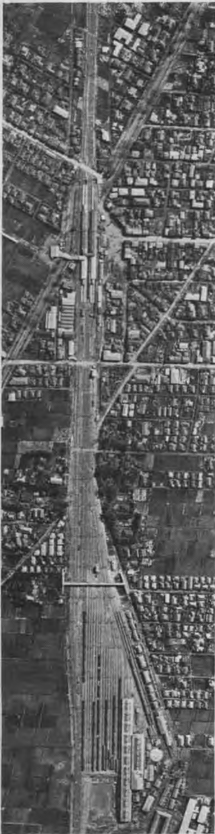
Marshalling yard near Tokyo apparently is for motorized suburban cars. Almost all lines in Tokyo vicinity are electrified and double tracked. Power is from overhead.
