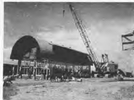
CRANE LIFTS QUONSET ONTO FOUNDATIONS
