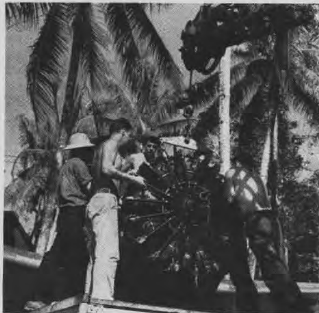
INTEGRATED PROGRAM IS ELIMINATING MAJOR REPAIR IN OPEN
