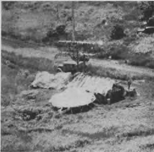
Jap radar installation first seen at Wewak is known as Wewak-Yagi type. Antenna has two rows of horizontally aligned rods
