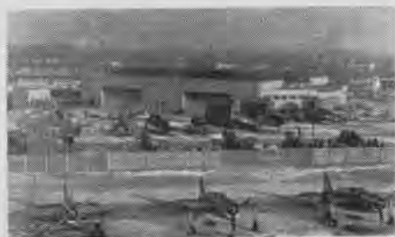
FOUR TYPES MAKE UP 180 FT. BLAST FENCE
