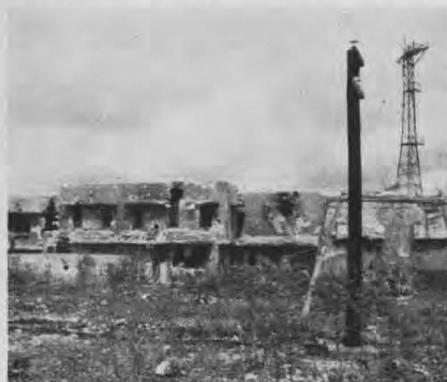
This was formerly the radio station building in the town of Tinian. Note three typical platforms on steel lattice mast at right
