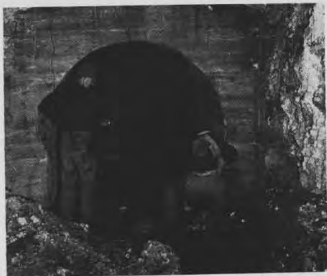
Underground barrel-vaulted concrete structures found near Agana airfield on Guam were used by Japanese to store radio equipment
