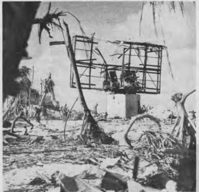
Destroyed Japanese radar of Attu type at Tarawa. Attached to a concrete base, it has a box screen and rotates on steel turntable
