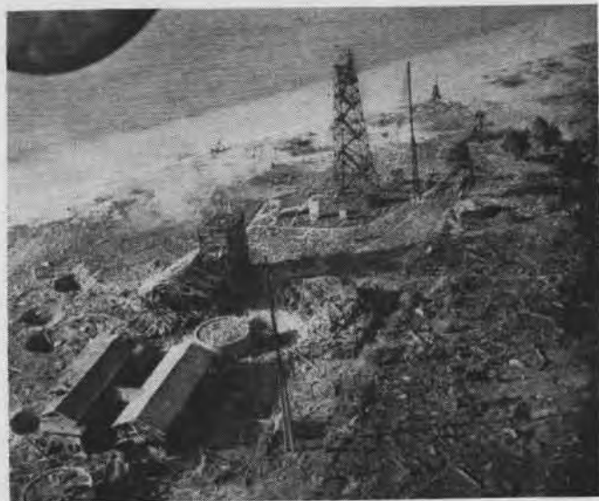
Photographs of Jap weather stations usually show three small instrument houses, painted white. Tower is another standard feature
