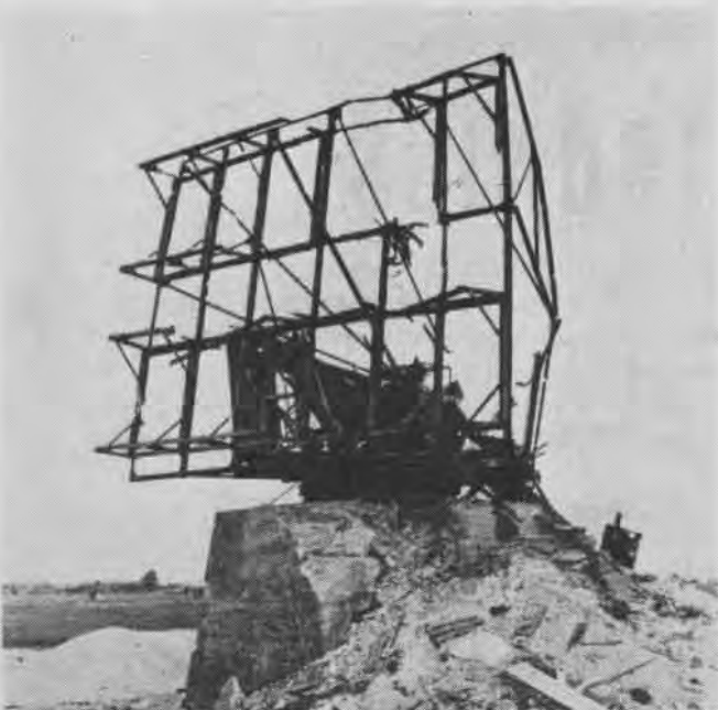
Captured Guadalcanal type radar at Kwajalein is mounted on high concrete base. Antenna rotates with shack to which it is attached
