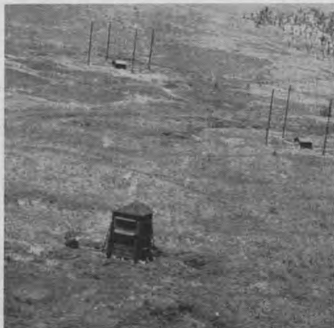
Housed high frequency Japanese direction finder is situated near two open Adcock-type medium frequency installations at Rabaul
