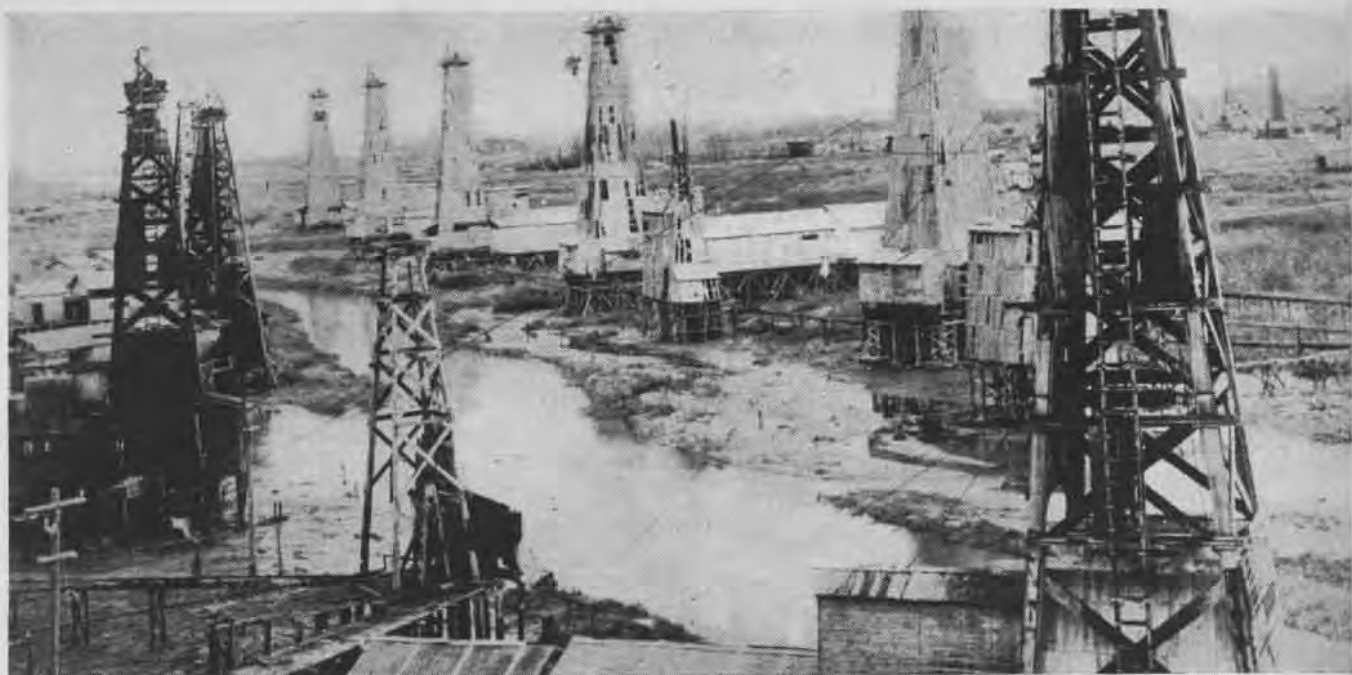
JAPANESE USE BOARDED-UP WOODEN DERRICKS AT ONE OF THEIR FEW REMAINING OIL FIELDS AT AKITA IN NORTHWEST HONSHU
