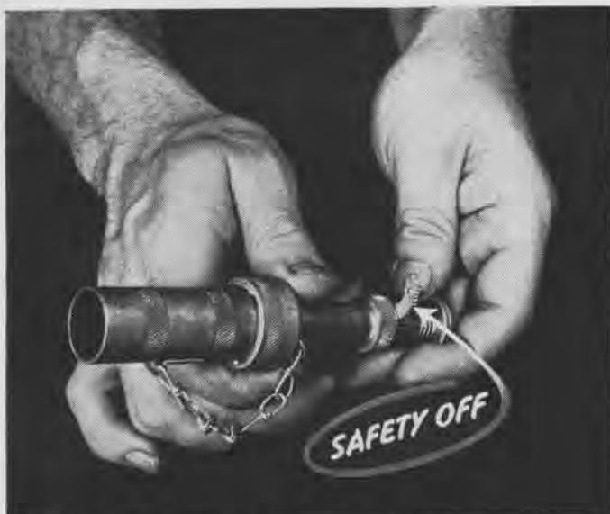
WITH SAFETY ARM IN THIS POSITION, THE PISTOL CAN OPERATE
