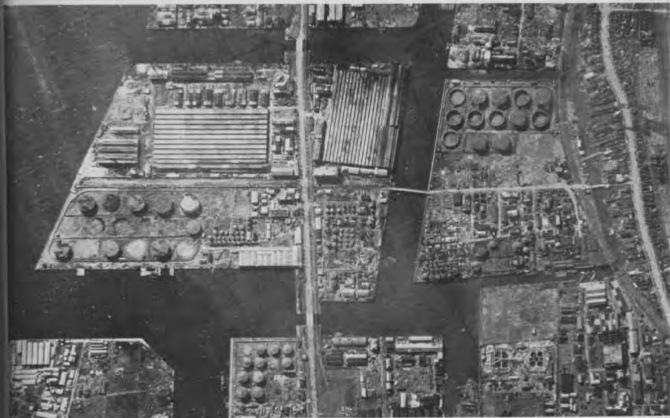
AMERICAN COMPANIES BUILT MANY OIL FACILITIES IN FAR EAST; INSTALLATIONS CONSEQUENTLY ARE SIMILAR TO THOSE IN U. S.
