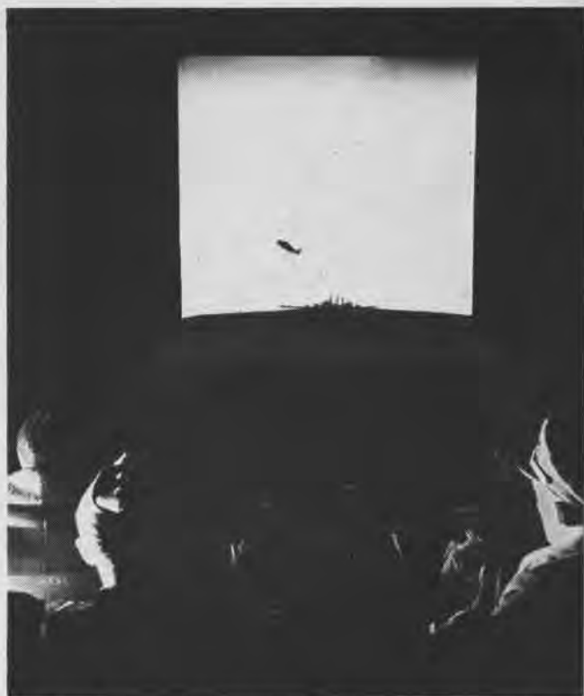
Pilots' eyes must be night-adapted to distinguish between friendly and enemy plane shadows on the night recognition screen. Pilots sit at distances simulating actual ranges of 550, 400, 250 feet.
