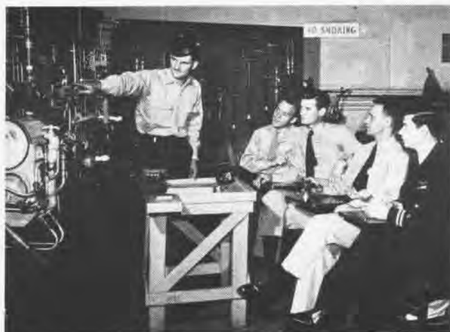
OPERATION OF NEW EQUIPMENT IS PART OF RESERVE TRAINING
