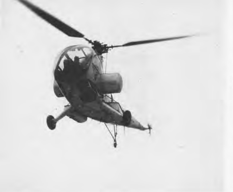
With stretcher case aboard a helicopter ambulance heads out on mercy flight. Blisters on each side cover up ends of stretcher
