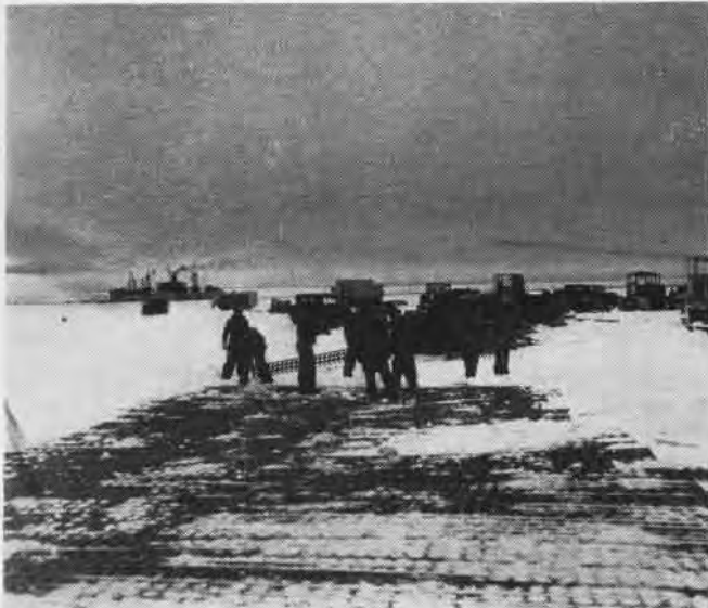
Workmen use steel matting to bridge a crevasse on Ross Sea ice shelf as transport Yancy unloads supplies for Little America.
