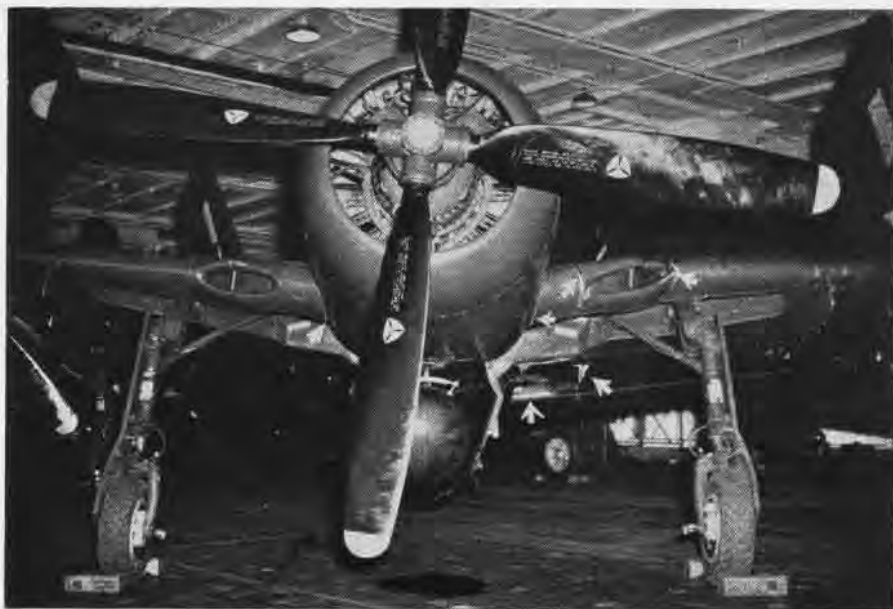
HARD LANDING PUTS PLANE OUT OF COMMISSION, SOMETIMES DAMAGES ARRESTING GEAR
