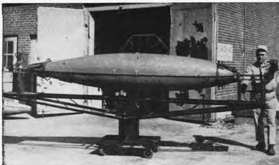
TANK MOUNTED IN SLOSHING CRADLE IS ROTATED BY HAND CRANK; EITHER END CAN BE RAISED
