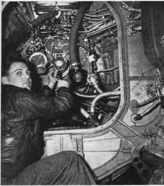
VP-ML-8 man demonstrates accessibility of rear of Neptune's engine for repairs; this feature makes the plane popular
