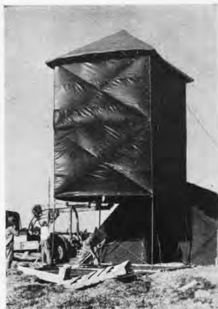
Portable parachute loft goes up as SMS-33 gets ready to service Marine pilots.
