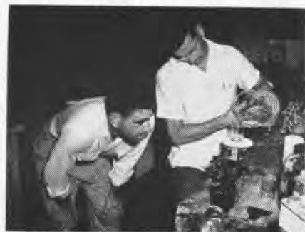
WEIGHING RESIN IS ONE STEP IN REPAIR WORK
