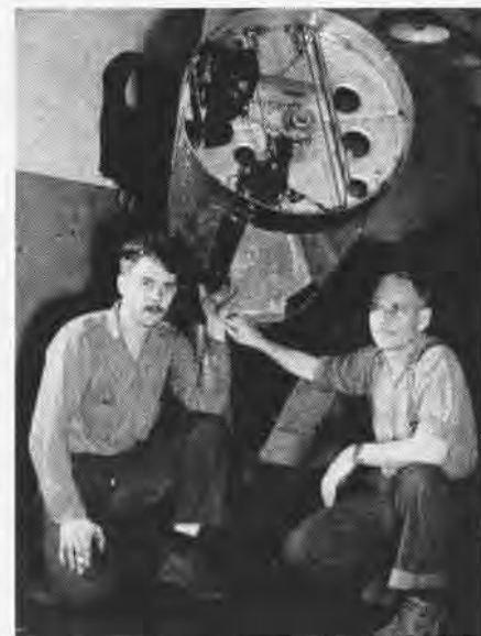
WINIGAR, FOREMAN DISPLAY WORKINGS OF TANK
