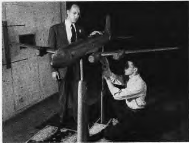
AERONAUTICAL ENGINEER Fresh watches L. Money make final adjustments on R5D model already rigged on struts for testing
