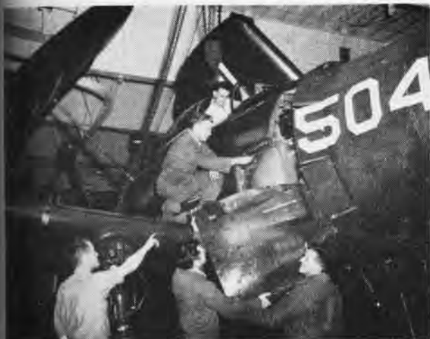
REPAIRING attack bomber for next flight are Budzinski, Rhodes, Litinski, McElroy and Barth—VA-728 mechs on the Antietam
