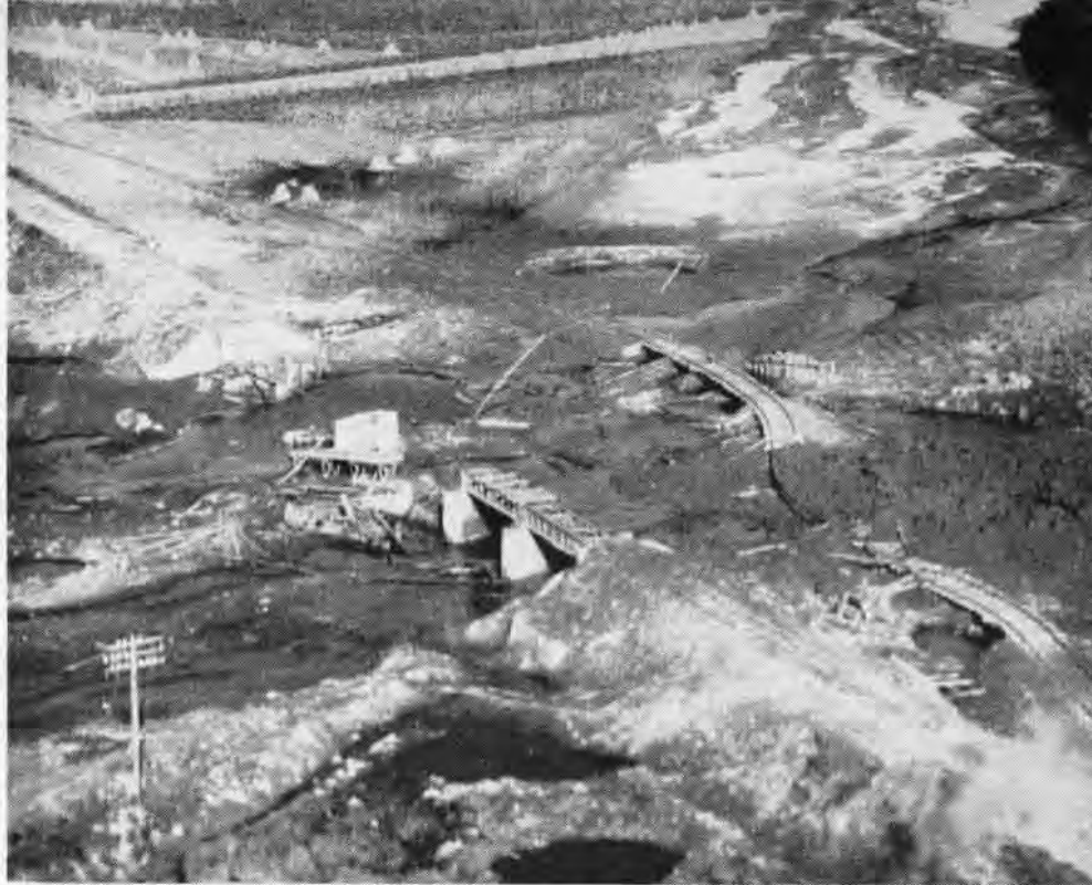
KOREAN railroad stock went down after the Navy sent Essex planes in to plaster this Communist rail bridge; note by-pass built after original tracks were destroyed by earlier raids
