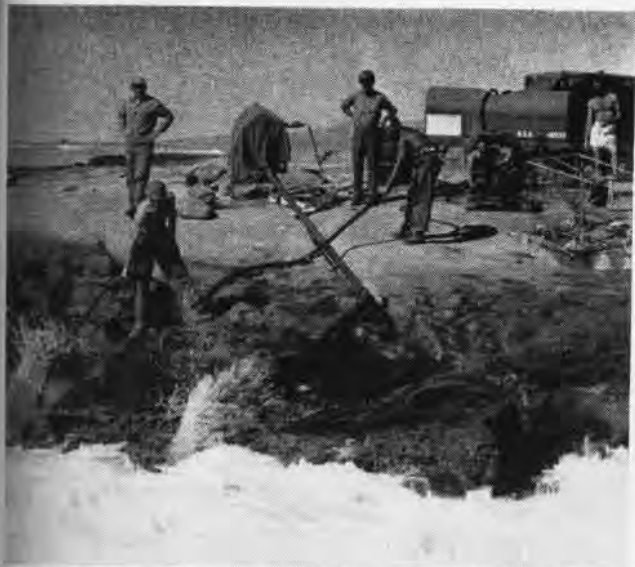
NO FRESH water supply was available on the island. Salt water distillation unit provided some 600 gallons of water daily
