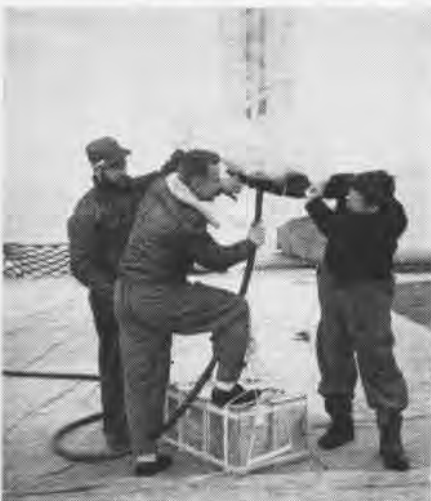
TECHNICIANS FINISH 'WEIGHING OFF' BALLOON
