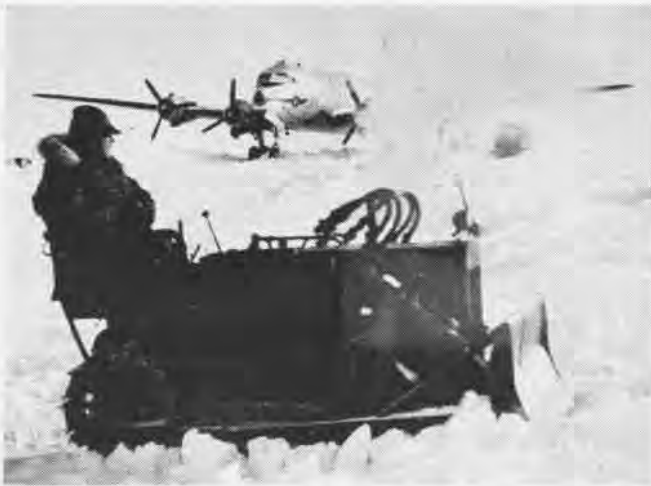
CATERPILLAR BROUGHT BY AF C-47 MAKES RUNWAY FOR STRANDED C-54
