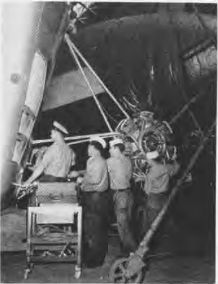
WITH erection of airship nearly completed engine on car on outrigger is installed
