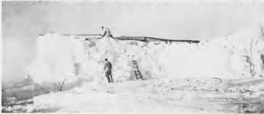
AIRPLANE SHELTER, ANTARCTIC STYLE, DIDN'T KEEP PLANE ENGINES FROM ICING BADLY
