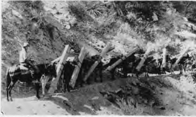
PACKING lumber by burro train up mountain trails is technique of hydrographic surveying now made obsolete by helicopter use
