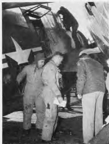
COD MEN MULL OVER DETAILS OF LOADING TBM
