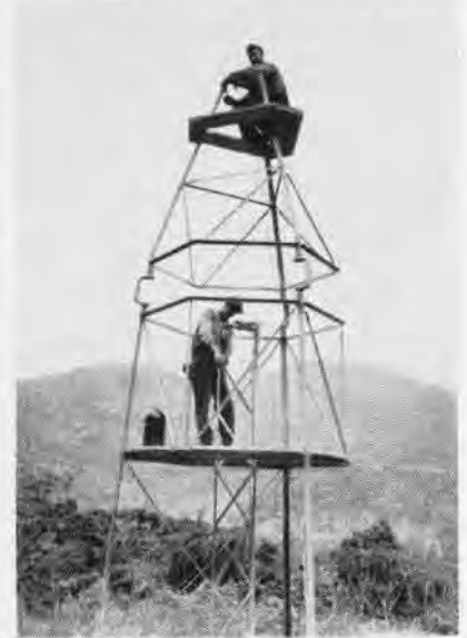
WORKERS in Venezuela jungle erect tower for taking triangulation sights
