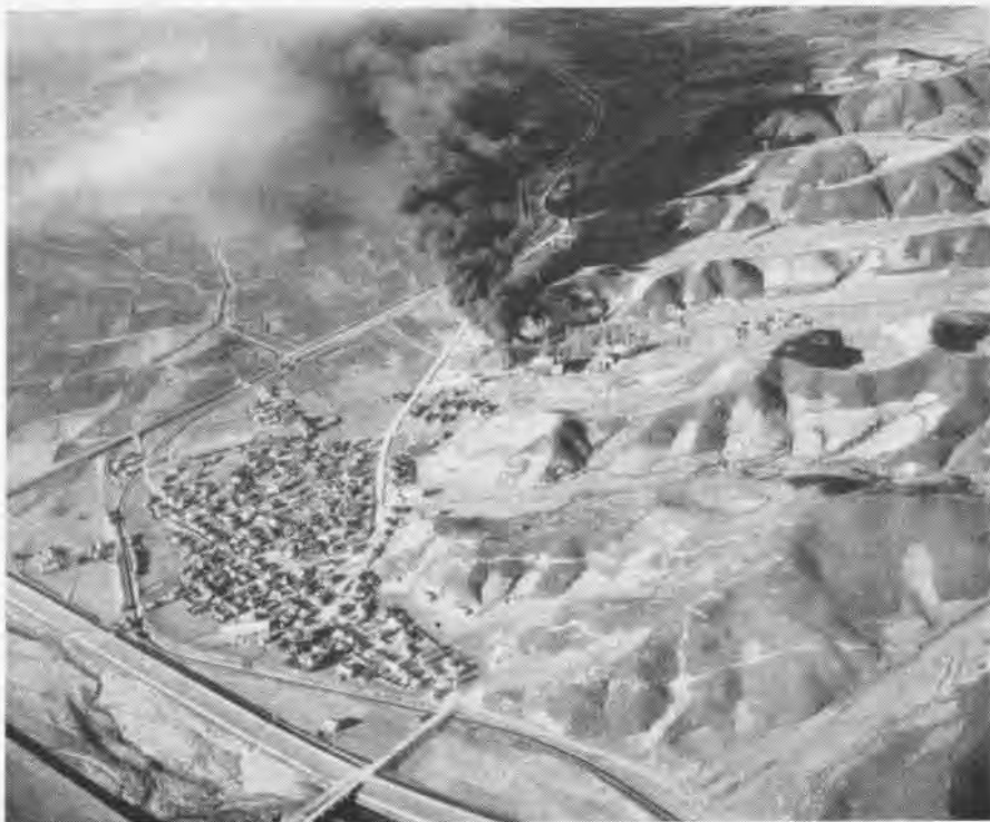
BLACK SMOKE pours out of transformer station at Chongjin, near Manchurian border, after Boxer's Skyriders and Corsairs deliver heavy bombloads to seacoast town's main "industry"
