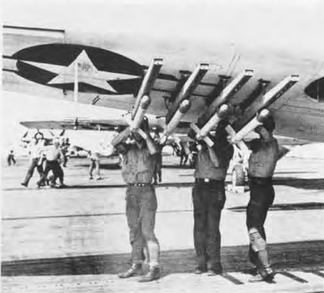
RAILS —First Navy rockets were fired from TBF's rails
