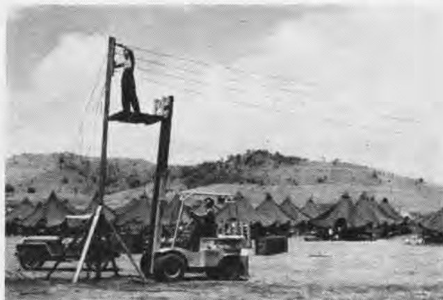
POWER LINES ARE STRUNG BY COLE AND PATCHETT IN FASRON CAMP
