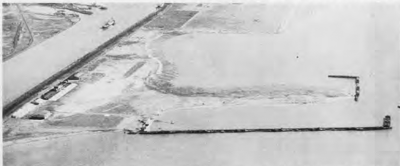
PHOTO TAKEN IN 1937 SHOWS OLD NAVY DESTROYERS FORMING BREAK-WATER (FOREGROUND) TO AFFORD MOORING CHANNEL FOR CHINA CLIPPER
